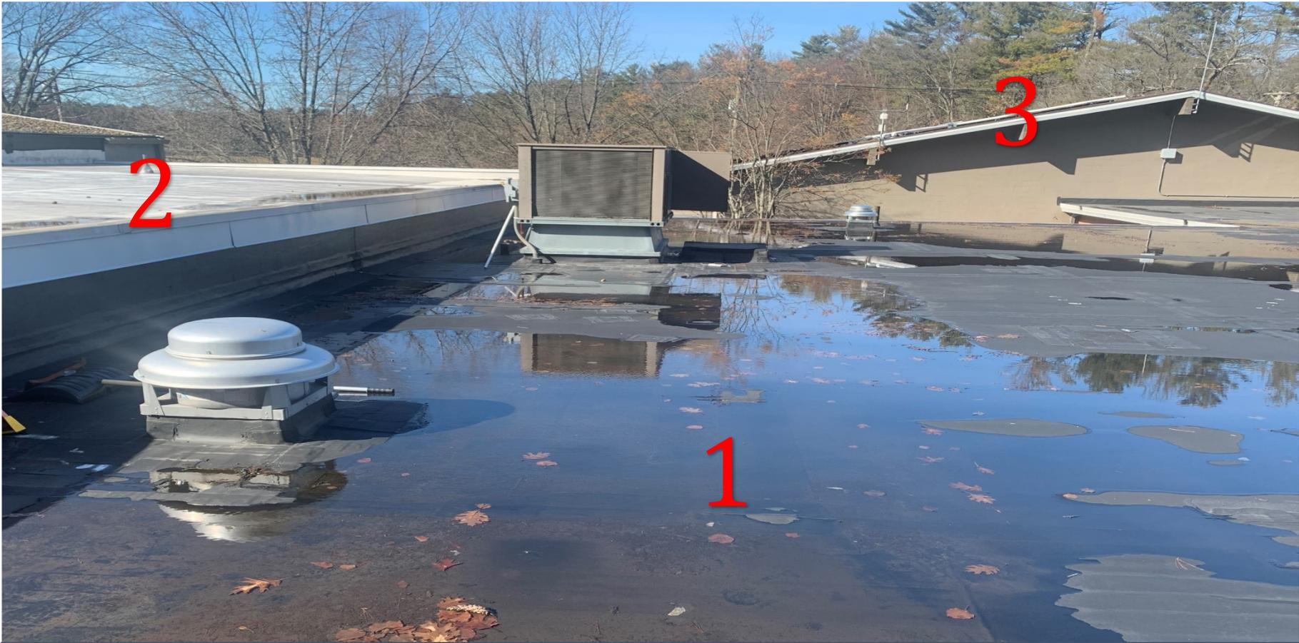
Pooling of water on roof of building. Note there are three levels of roof lines.
