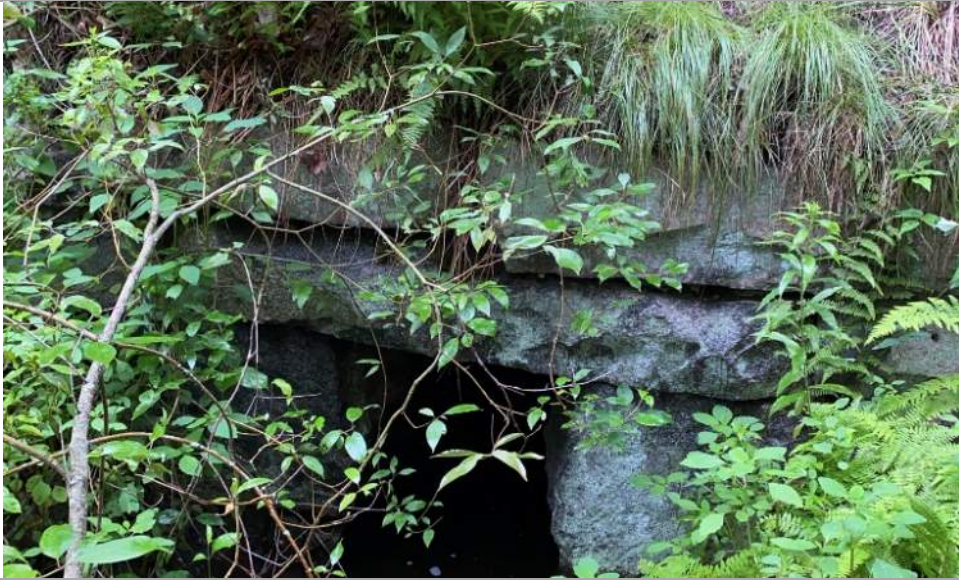
South (outlet) end
