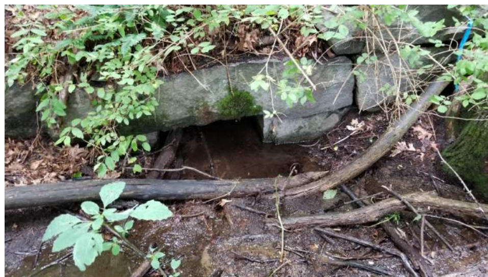
View of northern end of Structure 1271
