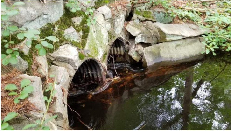
View of southern end of Structure 127F from western bank
