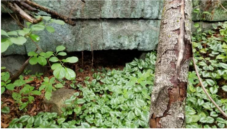
View of southern end of Structure 127H
