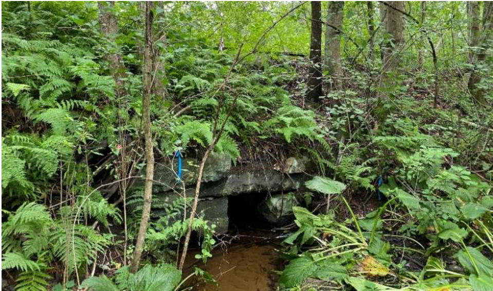
North (inlet) end and embankment
