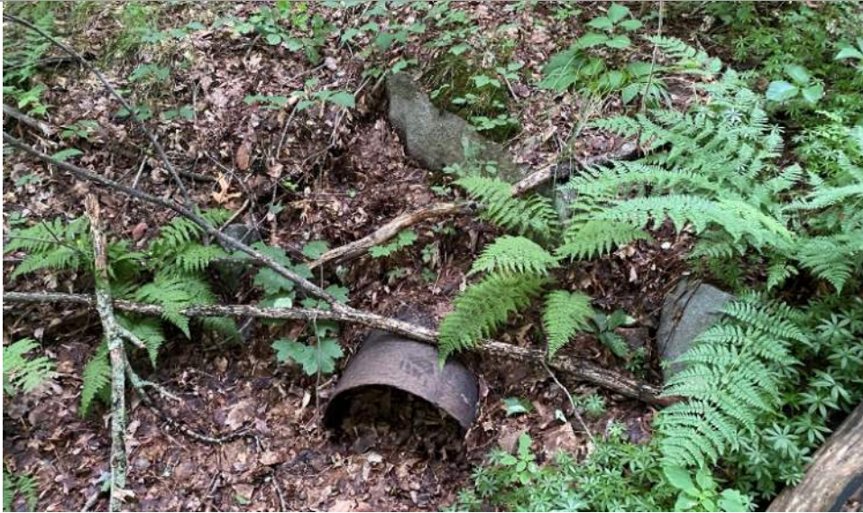
North end and embankment
