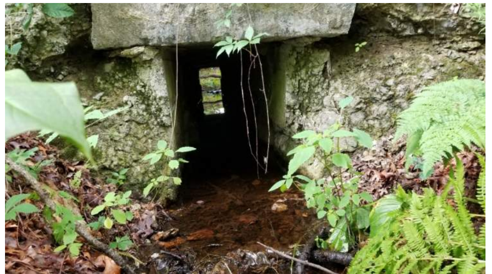
View through northern end of Structure 127E; visible straight through culvert
