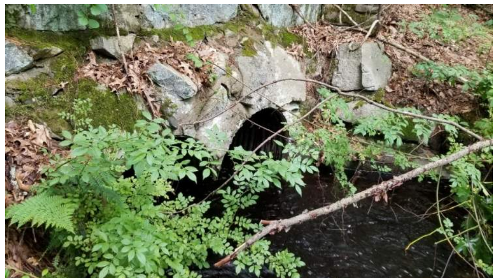
View of northern end of Structure 127F from eastern bank
