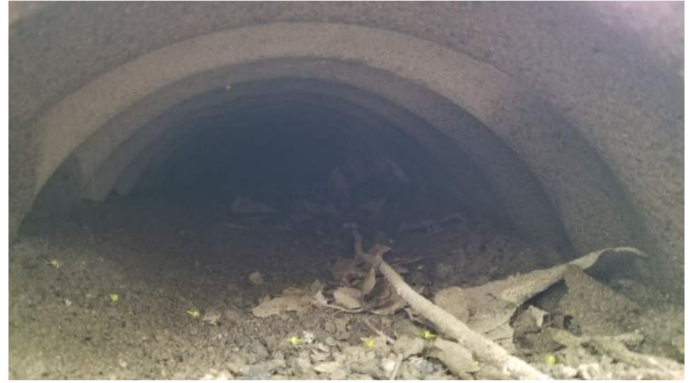
View through culvert from south end
