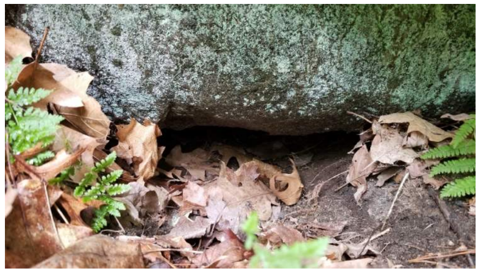
View of southern end of Structure 129A with limited wildlife passage
