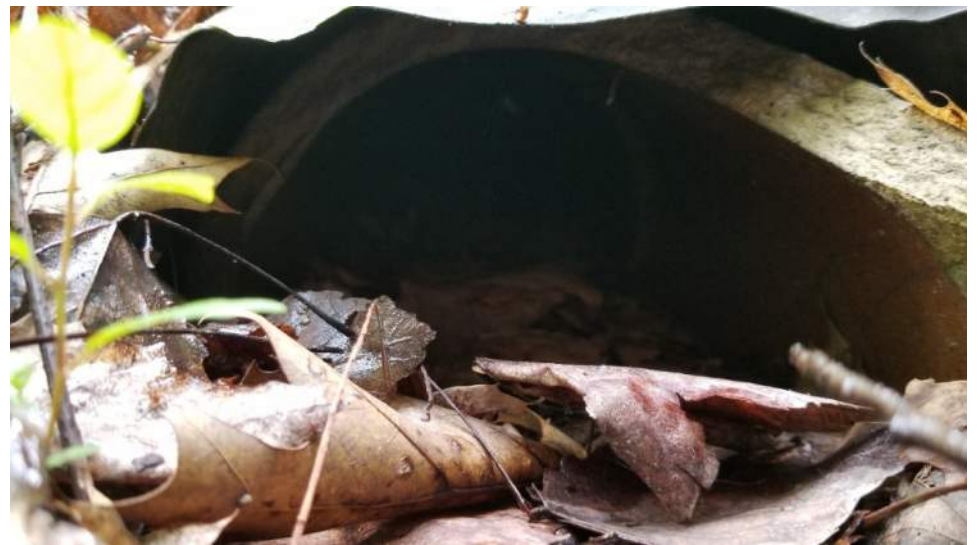
View through northern end of pipe
