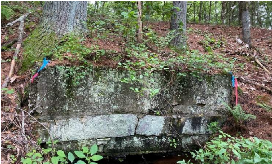
View of headwall at northern end and embankment.
