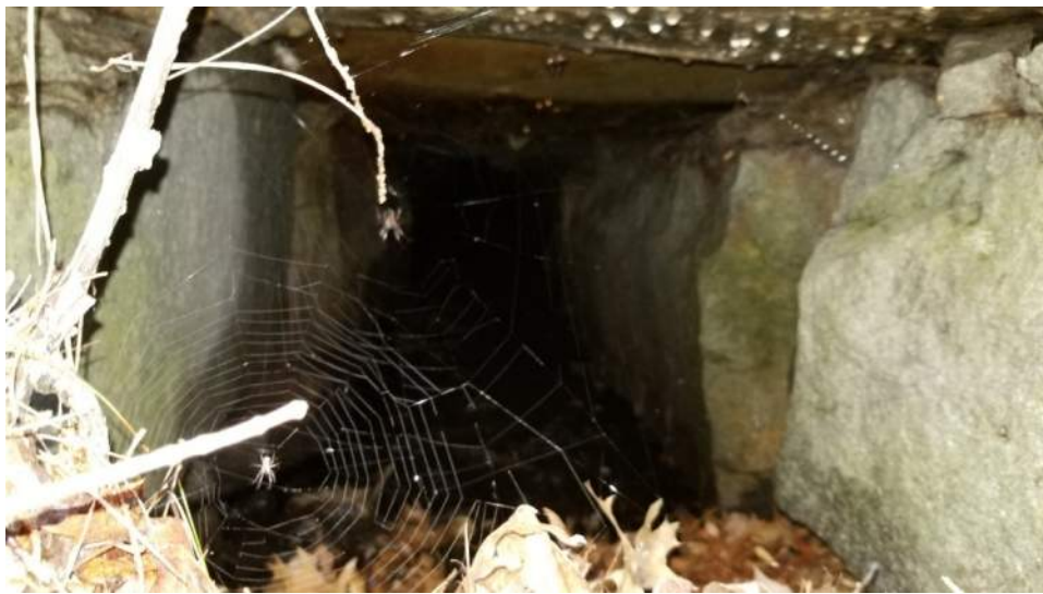
View through Structure 127J from southern end
