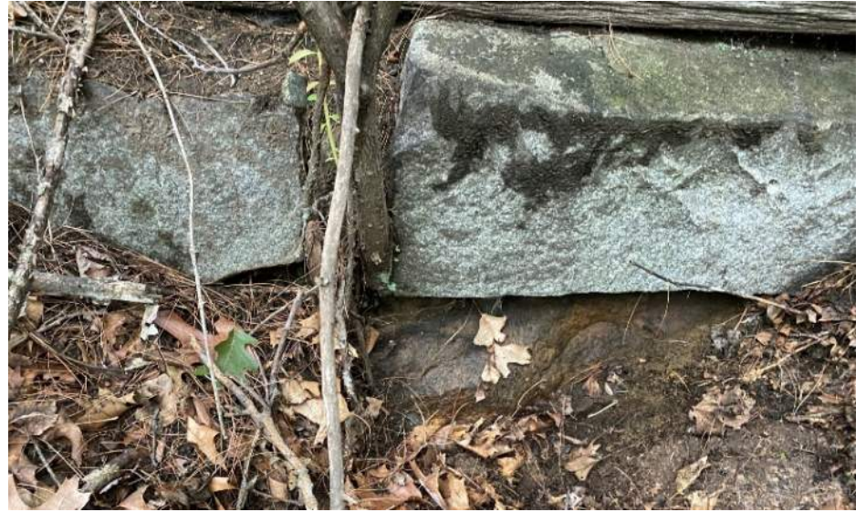
Debris at buried south opening
