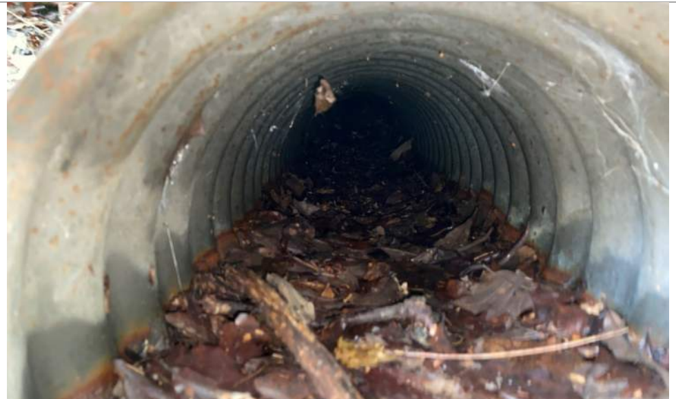
View of the inside of culvert from the north end.
