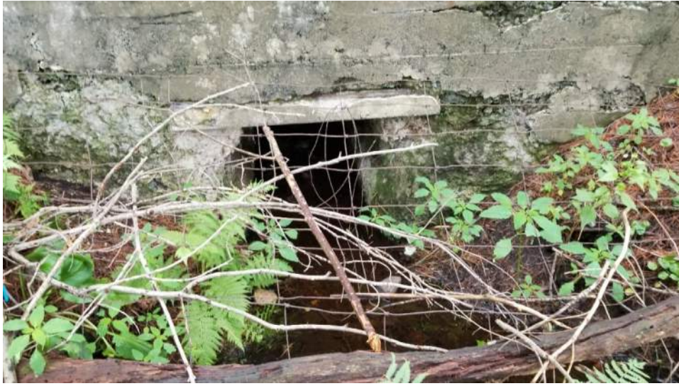
View of southern end of Structure 127E
