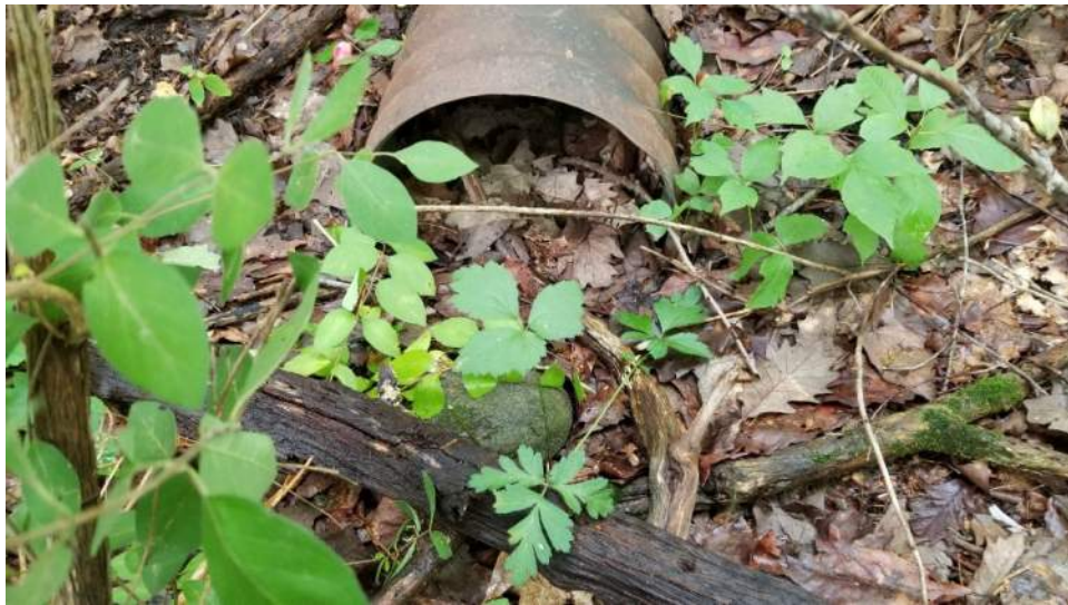
North end of culvert and embankment
