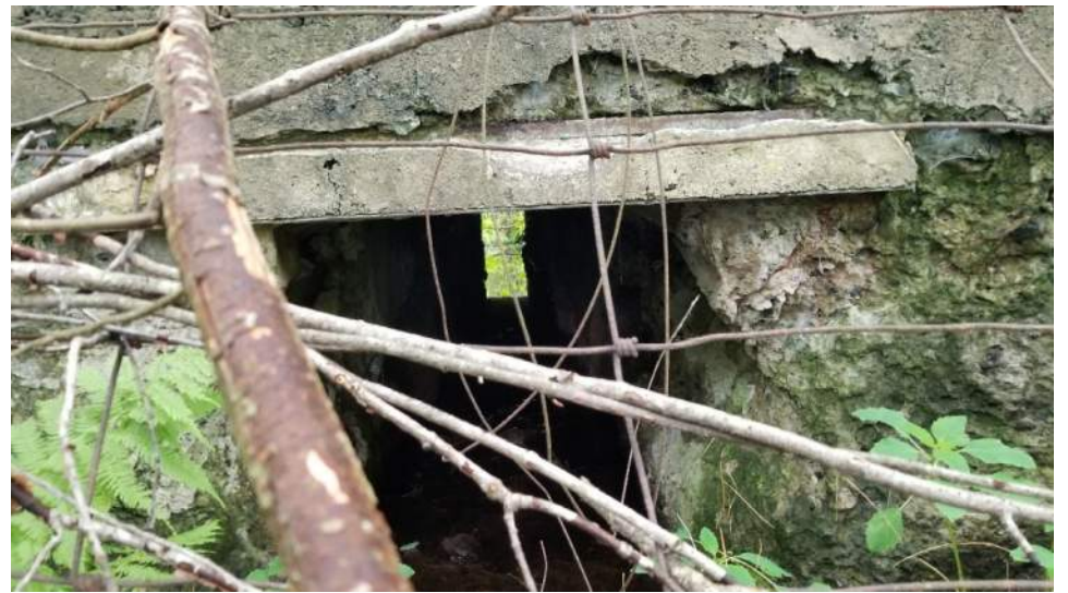
View through southern end of Structure 127E; visible straight through culvert
