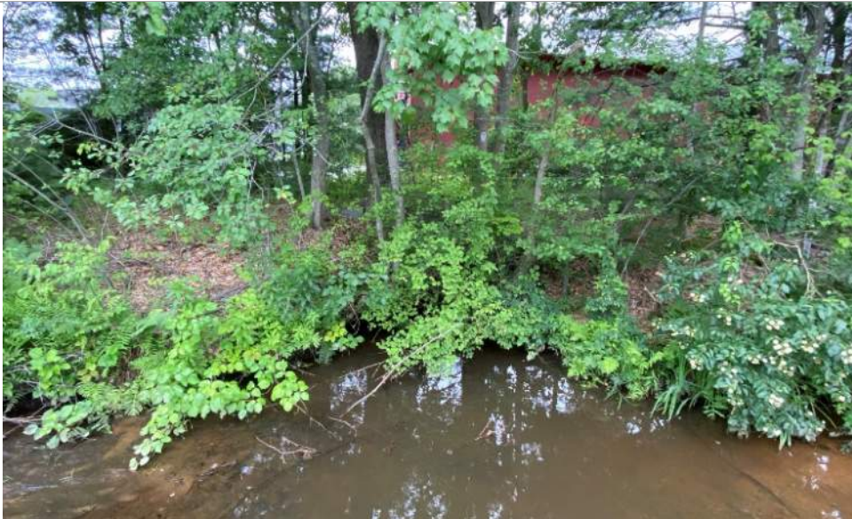
North end and embankment
