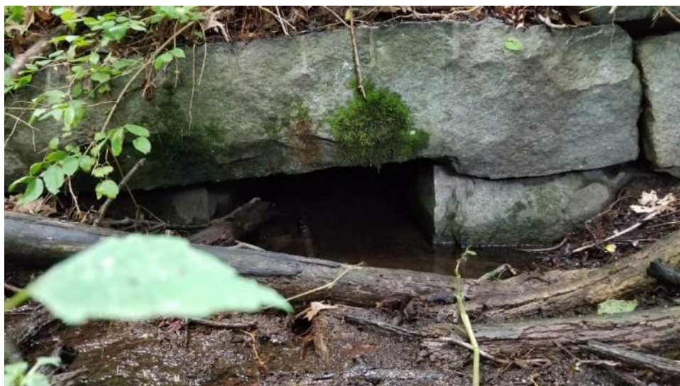
Alternate view of northern end of Structure 1271
