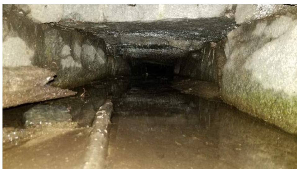
View through Structure 1271 from the northern end
