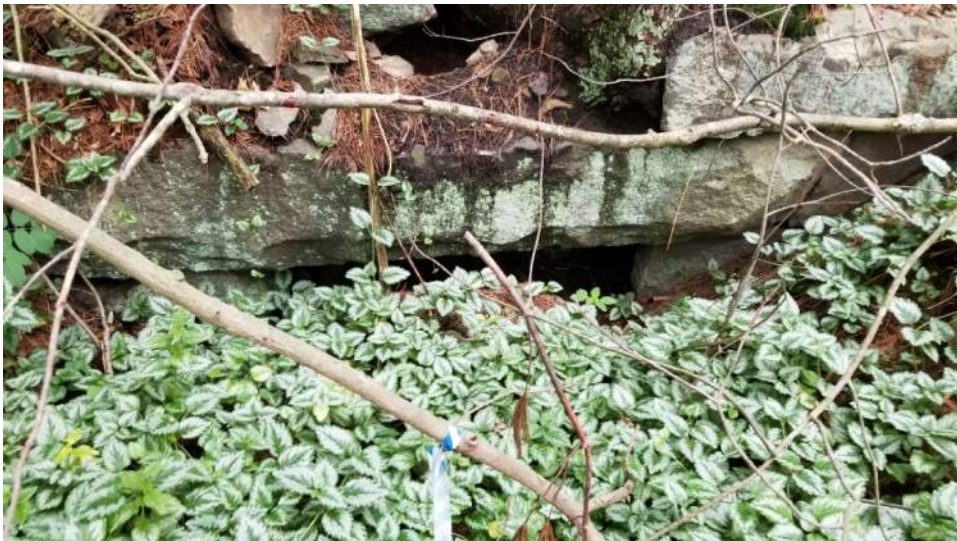
View of northern end of Structure 127H
