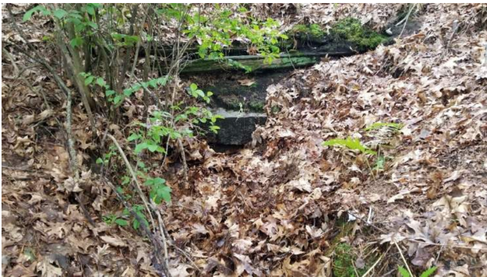
View of north end of Structure 127C
