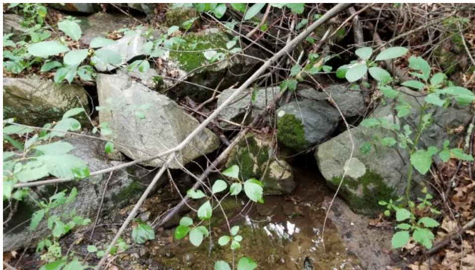
View of southern end of Structure 1271
