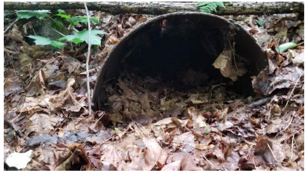
Looking through the northern end of the pipe
