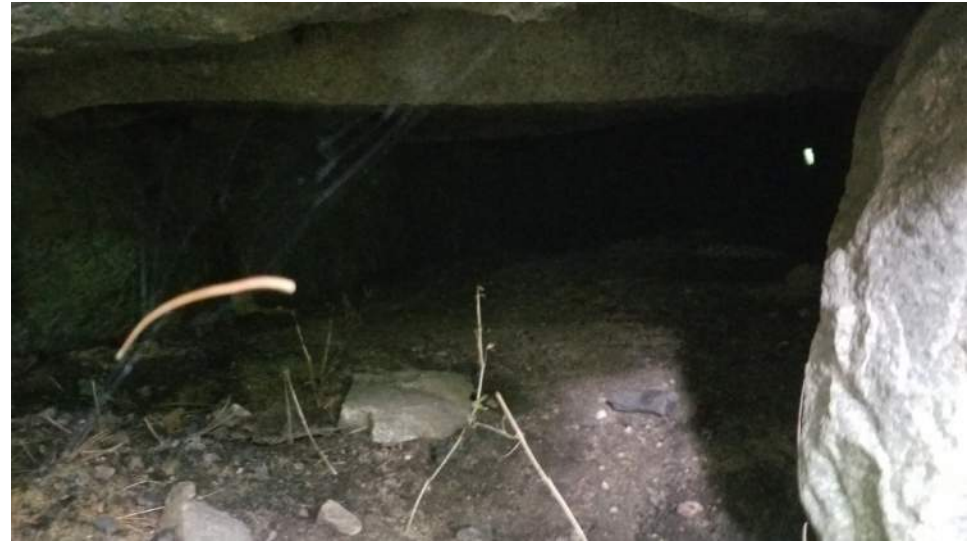
View through northern end of Structure 127H; light through the southern end is visible
