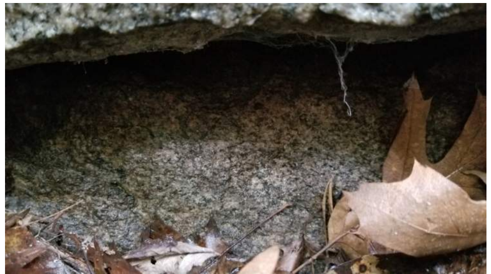
View inside north end of pipe
