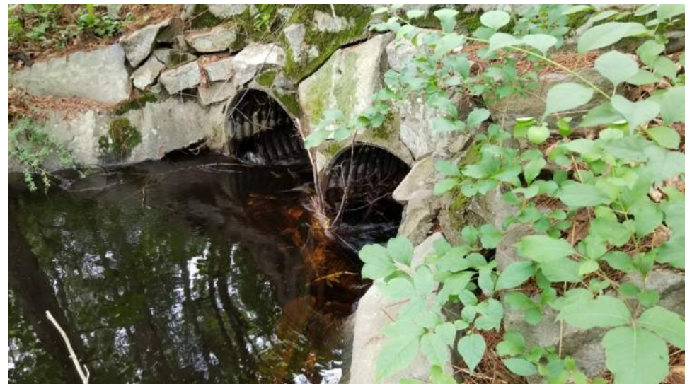
View of southern end of Structure 127F from eastern bank
