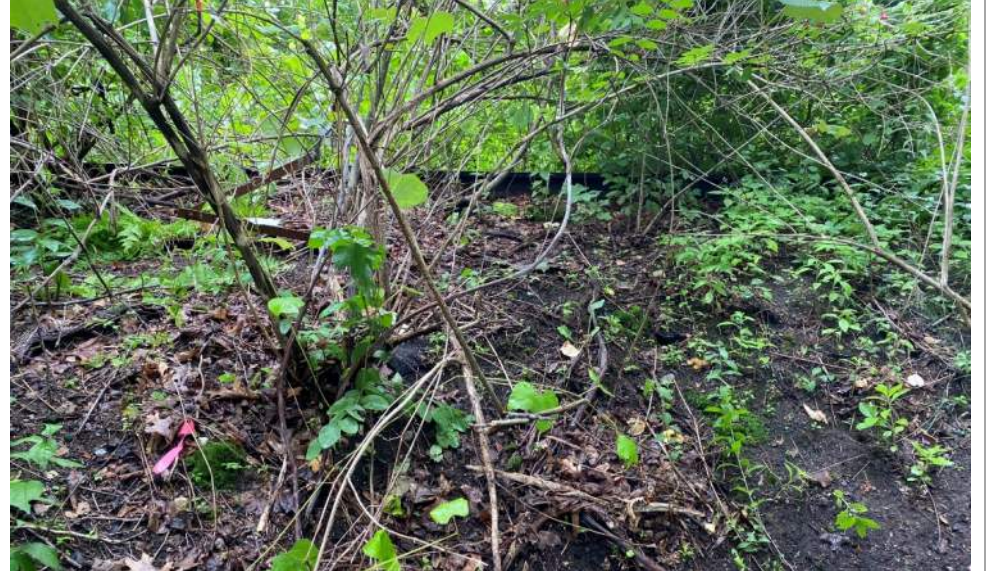
View of south embankment.
