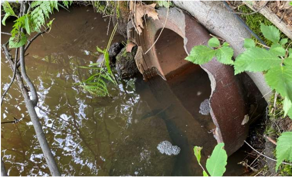
North end (outlet) of Structure 127B
