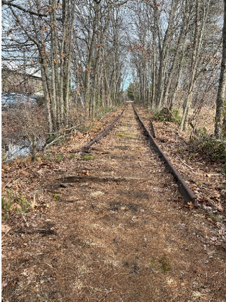
Photo 1: Near Sta. 108+50 looking north. Rails have not been removed in this location, but low brush has been cleared.
