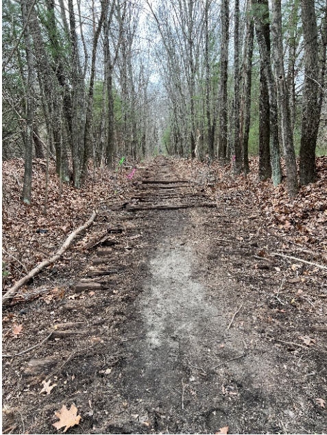
Photo 5: Near Sta. 215+75 looking south. Rail in this section has been removed
