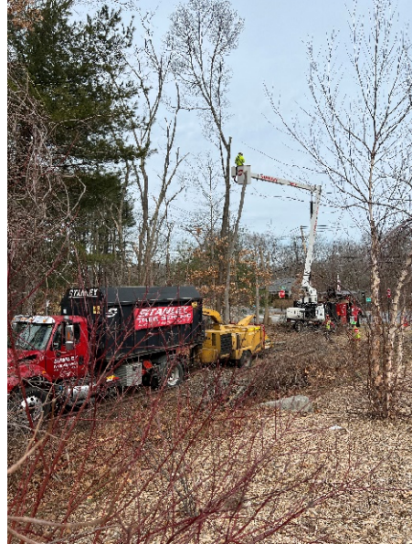
Photo 2: Near Sta. 174+50. Tree cutting and removal has begun.
