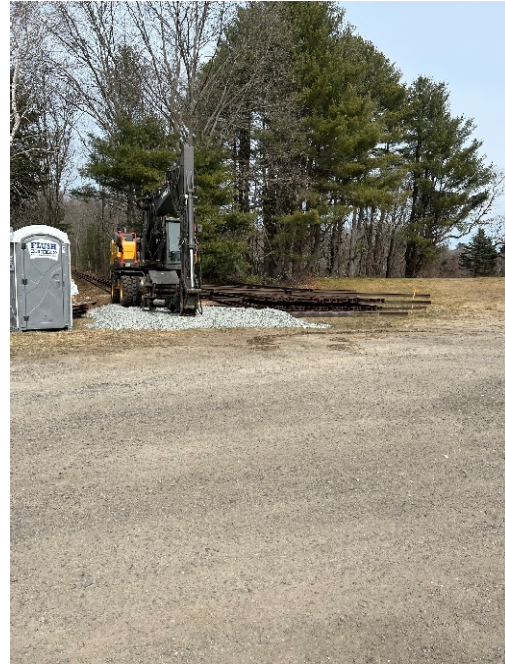
Photo 10: Sta. 320+00 looking north
