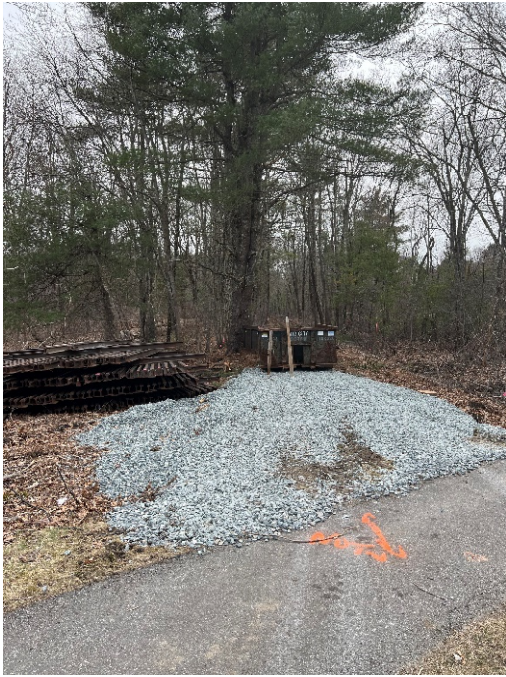
Photo 9: Sta. 307+50 looking south, standing at North Road
