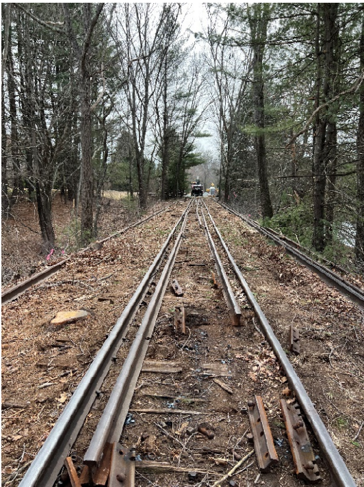
Photo 11: Sta. 325+00 looking south
