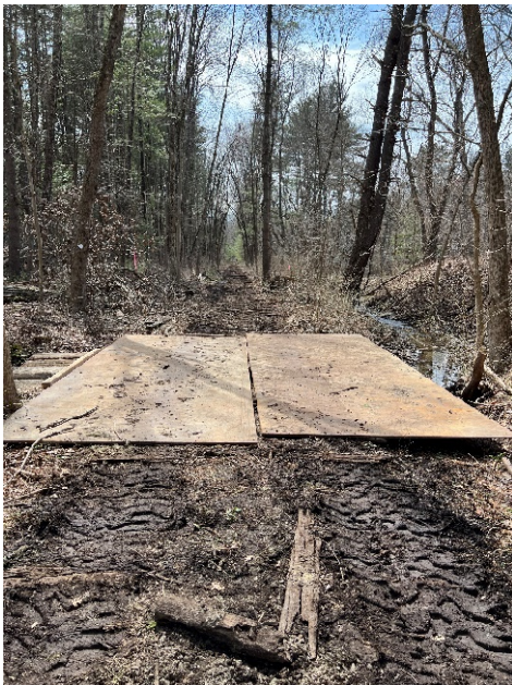
Photo 3: Sta. 167+50 looking south
