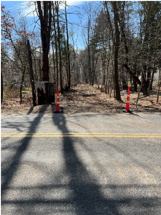
Photo 15: Sta. 143+00 looking south, standing at Old Lancaster Road
