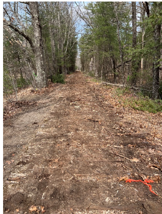
Photo 16: Sta. 266+00 looking north
