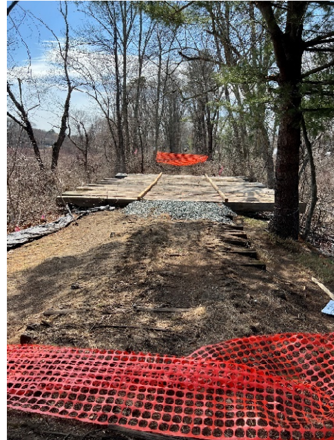
Photo 2: Sta. 127+00 looking south towards Hop Brook
