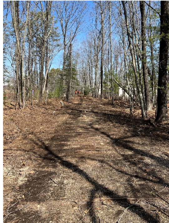
Photo 12: Sta. 101+00 looking north
