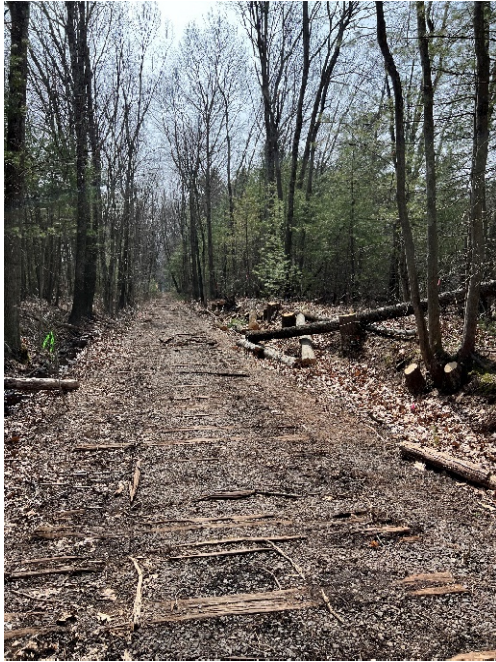
Photo 5: Sta 215+50 looking south
