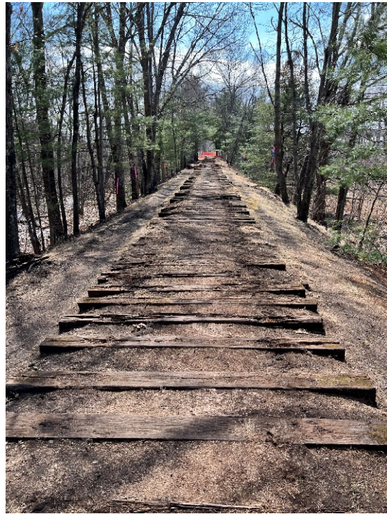
Photo 14: Sta. 129+00 looking south
