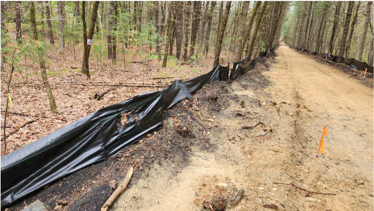
Photo 6: Silt fence ripping and a broken stake in the fence along segment 10. Photo taken on 5/05/23
