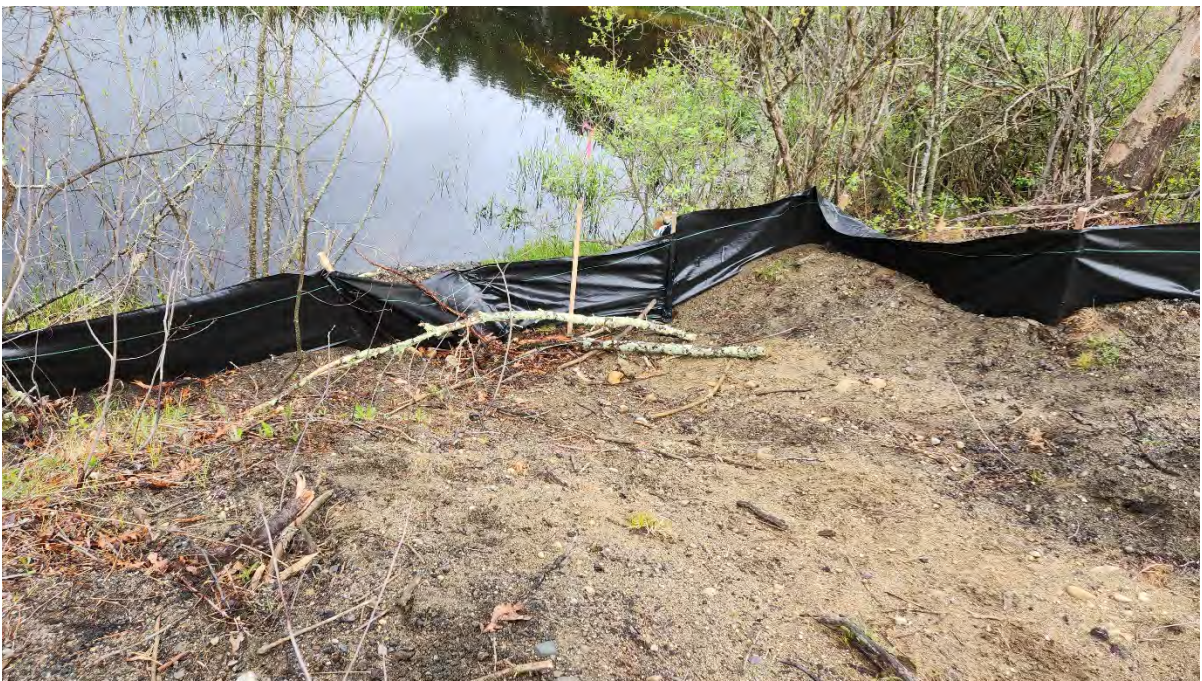
Photo 9: Silt fence sagging and broken stake in the fence at Hop Brook Bridge along segment 8. Photo taken on 5/05/23
