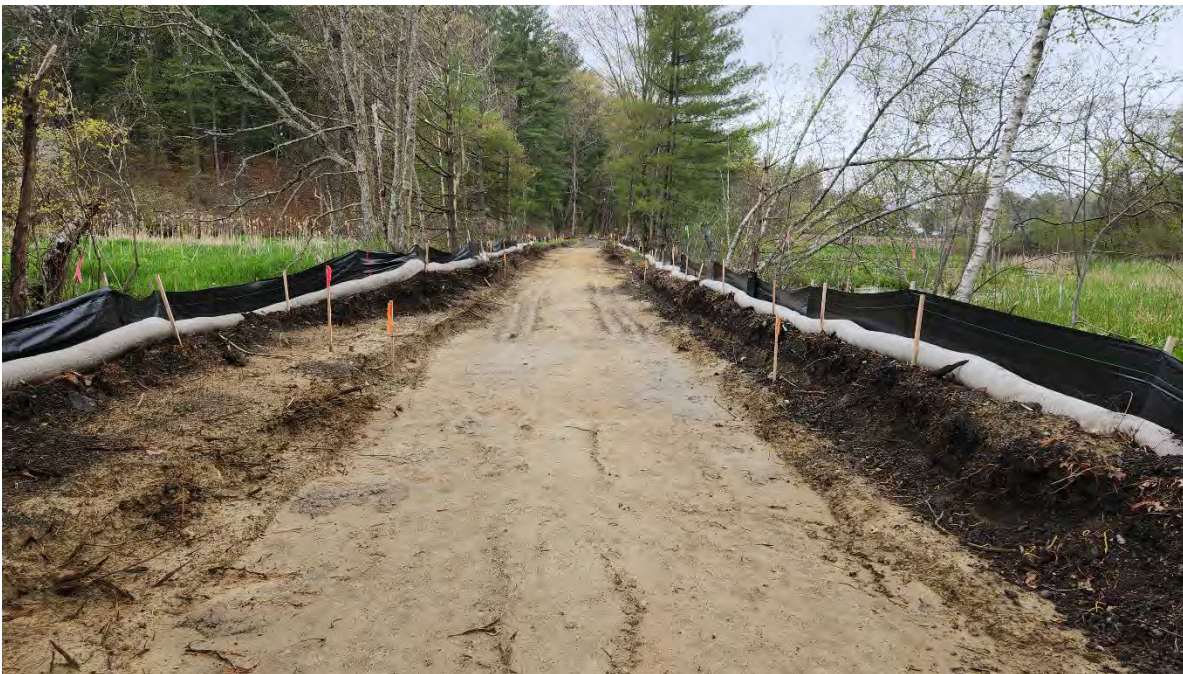
Photo 1: Silt fence and filter tube functioning properly along segment 14.
