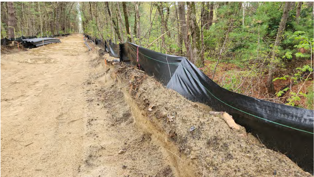
Photo 7: Broken stake in the silt fence along segment 10. Photo taken on 5/05/23
