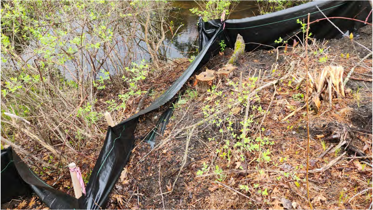
Photo 10: Silt fence sagging at Hop Brook Bridge along segment 7. Photo taken on 5/05/23
