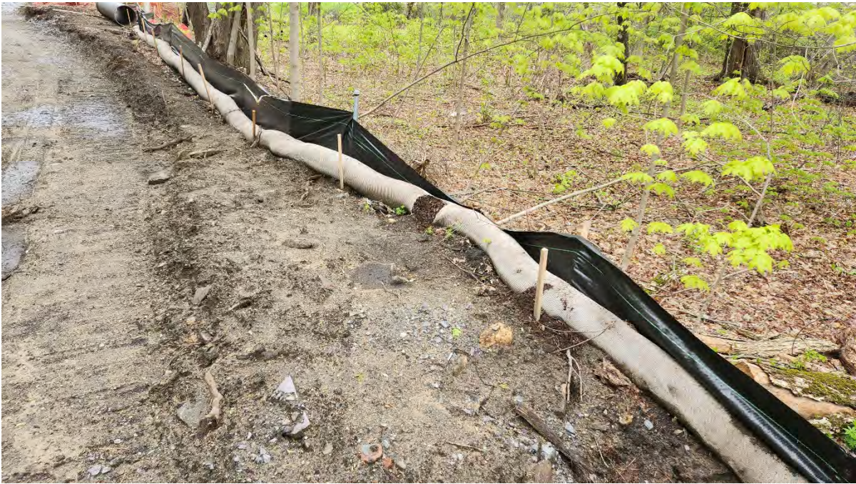
Photo 2: Broken filter tube and notable sagging in the silt fence along segment 13. Photo taken on 5/05/23
