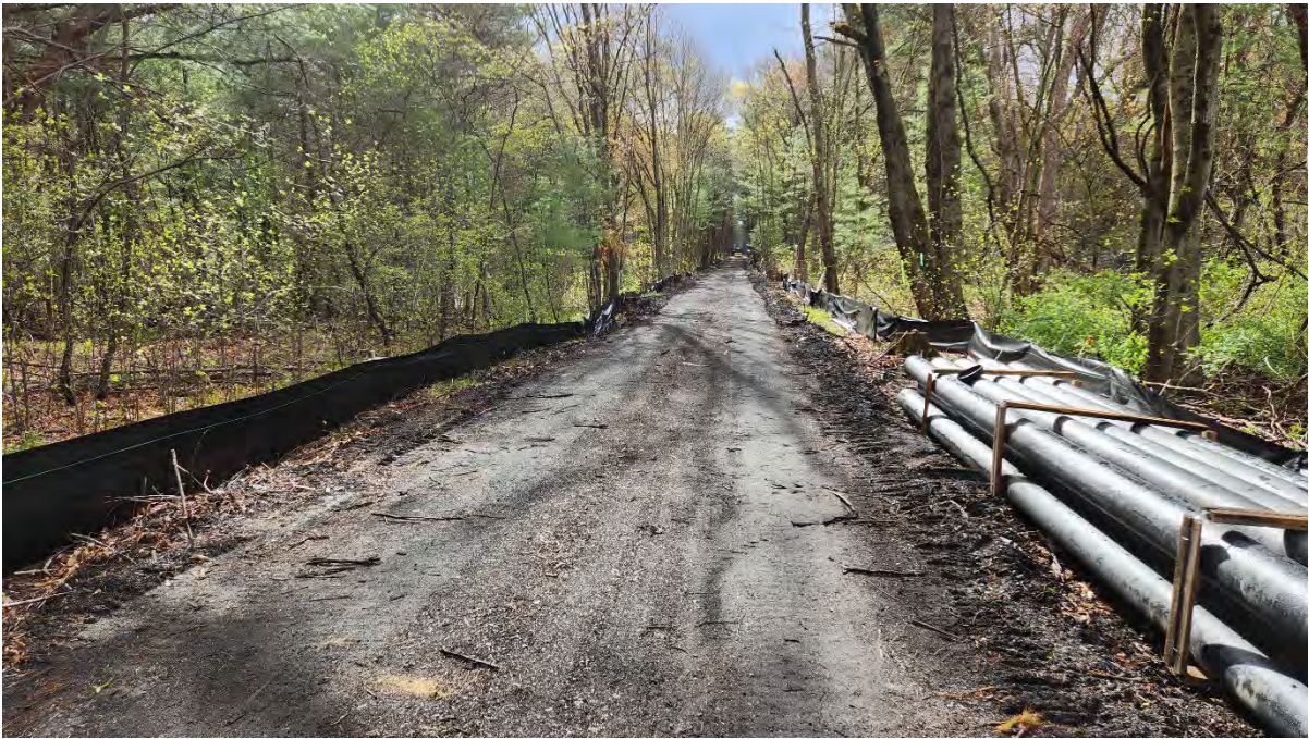
Photo 4: Silt fence functioning properly along segment 11. Photo taken on 5/05/23
