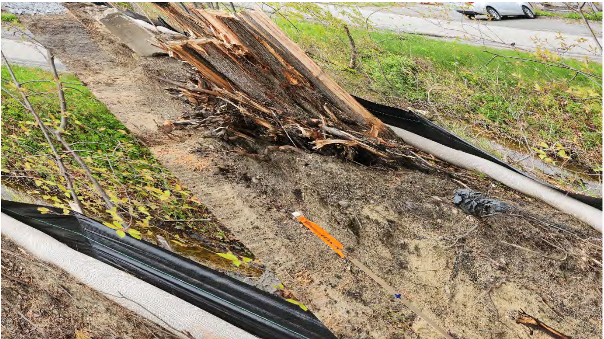
Photo 3: Notable sagging in the silt fence along segment 12. Photo taken on 5/05/23
