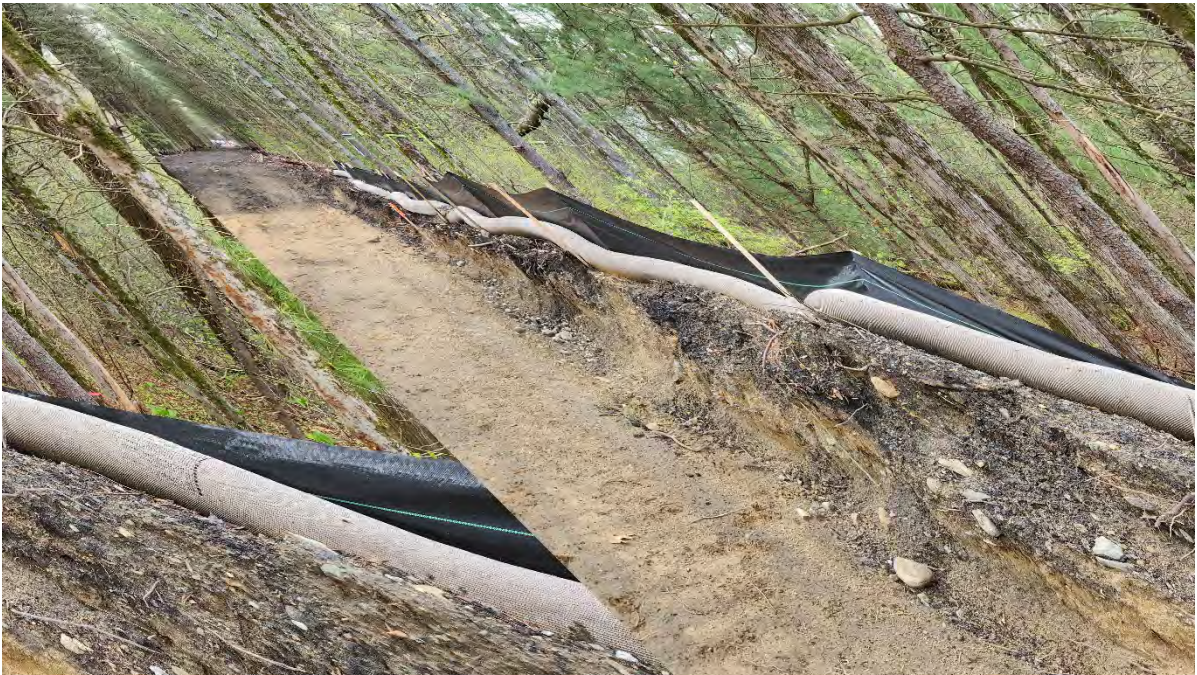
Photo 8: Broken stake in the silt fence along segment 9. Photo taken on 5/05/23
