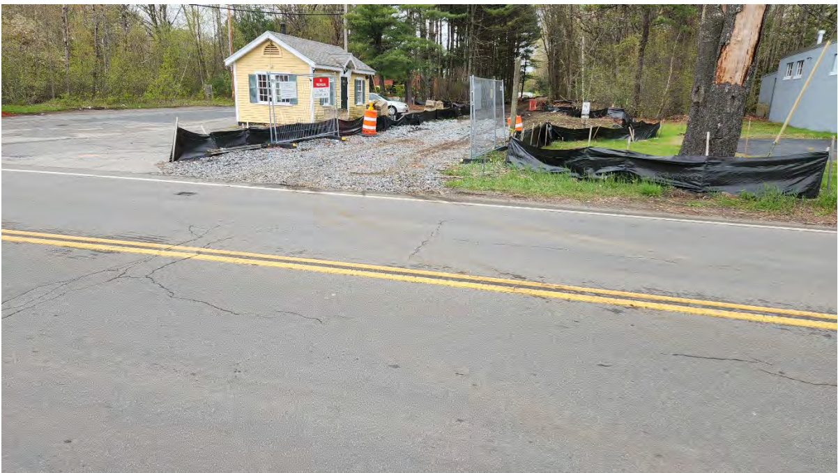
Photo 5: Construction entrance STA407+50 has visible sediment tracking into road. Photo taken on 5/05/23
