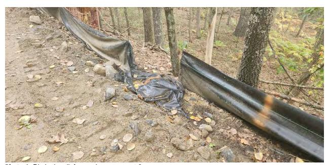
**Photo 1:** Rip in the silt fence along segment 8. Photo taken on 10/5/23
