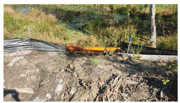
**Photo 5:** Rip in the silt fence near Bridge 127 along segment 14. Photo taken on 10/5/23
