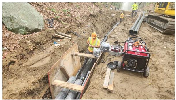
**Photo 2:** Conduit being installed along segment 9. Photo taken on 10/5/23
