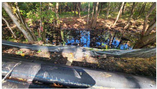
**Photo 4:** Stake in silt fence broken along segment 14. Photo taken on 10/5/23
