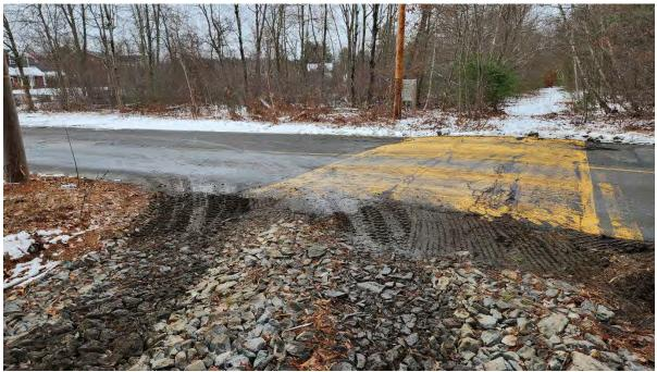
**Photo 5:** Sediment is tracked into the road at construction entrance STA 407+. Photo taken on 1/30/24
