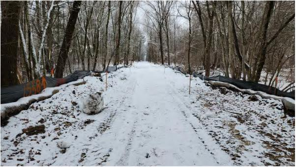
**Photo 4:** Stakes set along segment 9 at proposed path width for gravel base installation. Photo taken on 1/30/24
