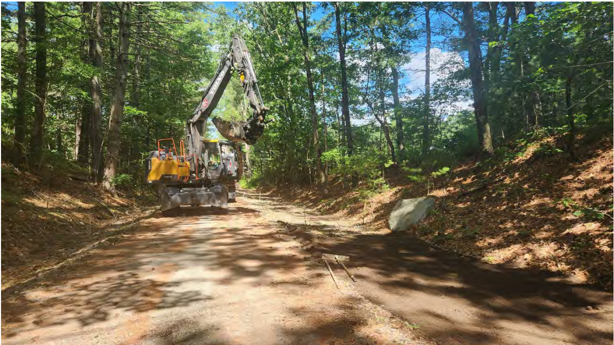
Photo 2: Loam installed along segment 9. Photo taken on 7/1/24
