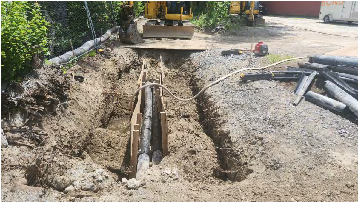
Photo 4: Dewatering during conduit work along segment 12. Photo taken on 7/1/24
