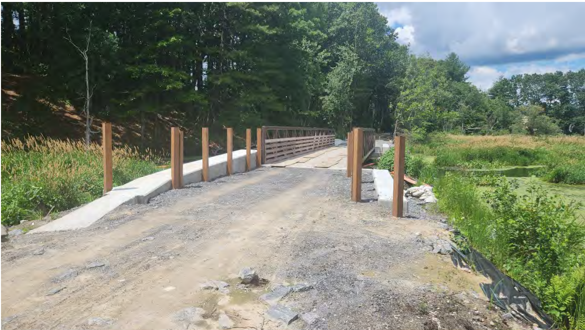
Photo 5: Timber rail installation in progress at bridge 127. Photo taken on 7/1/24.
