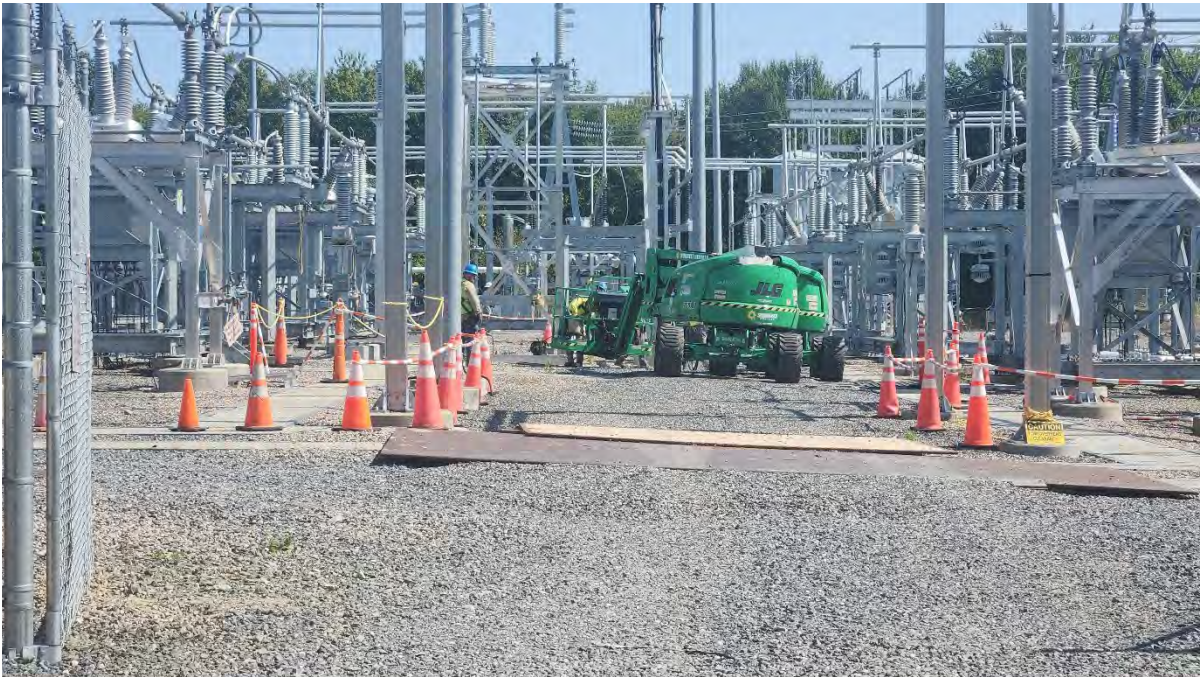
Photo 6: Cable splicing was conducted at the Eversource Substation. Photo taken on 9/16/24.
