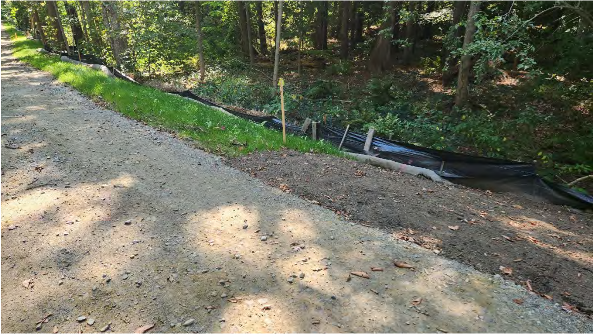
Photo 4: Loam and planting soil installed along segment 13. Photo taken on 9/16/24
