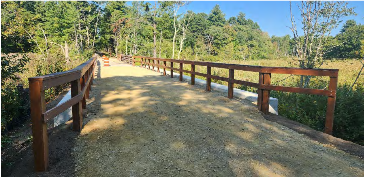
Photo 1: Timber rail post installation is complete at bridge 128.
