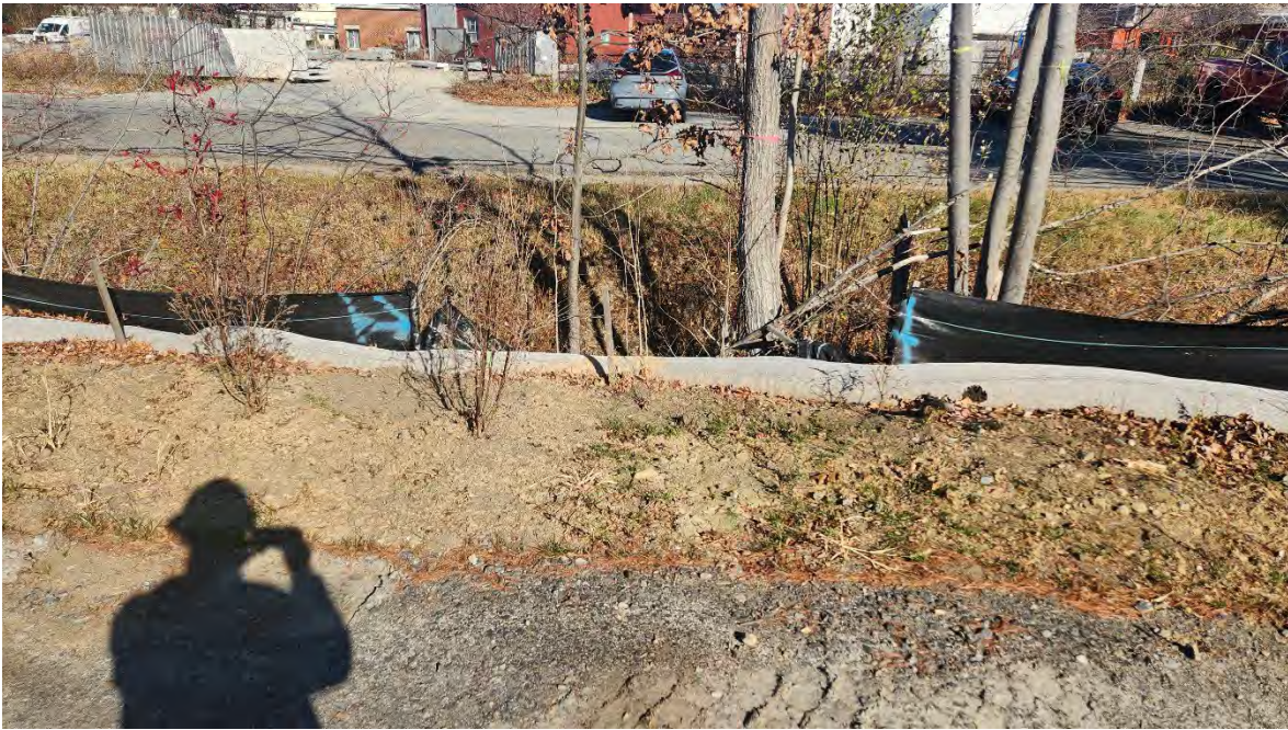
Photo 4: Broken stakes and rip in the silt fence along segment 12. Photo taken on 11/15/24
