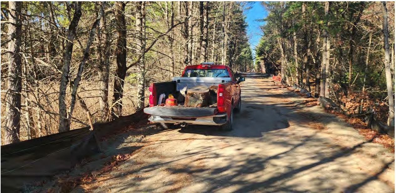
Photo 1: Tree stumps removed along segment 7. Photo taken on 11/15/24
