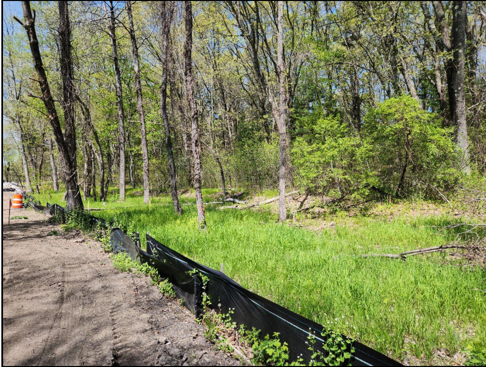
Photo 117. Native seed mix emerging densely in a large mitigation area. This photo was taken in Segment 14 at STA 740+50 facing west in 2024.
