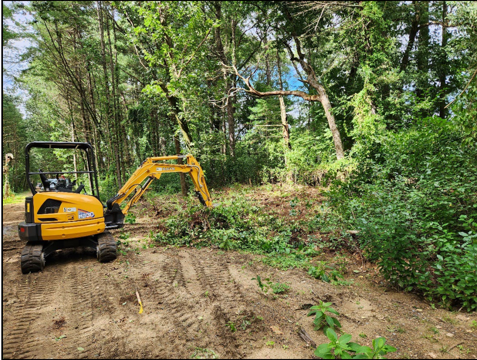
Photo 7. A mini excavator is shown removing invasive plants in Segment 10 in 2023. A dense patch of glossy buckthorn is visible to the right.
