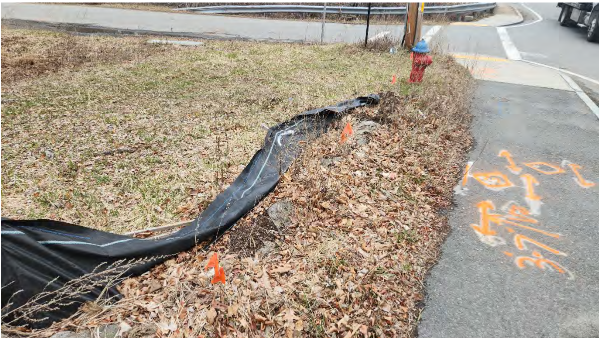
Photo 5: Rip in the silt fence along segment 12. Photo taken on 3/31/25.
