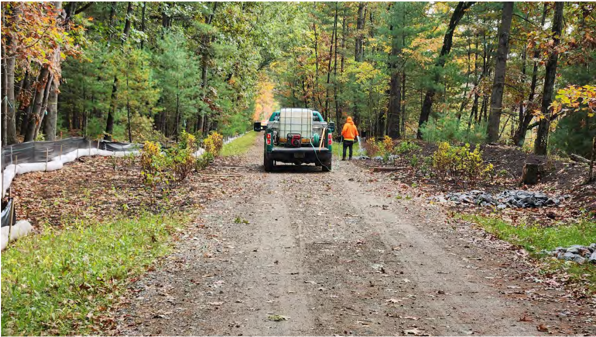
Photo 8: Installed plantings along segment 11. Photo taken on 10/15/24.
