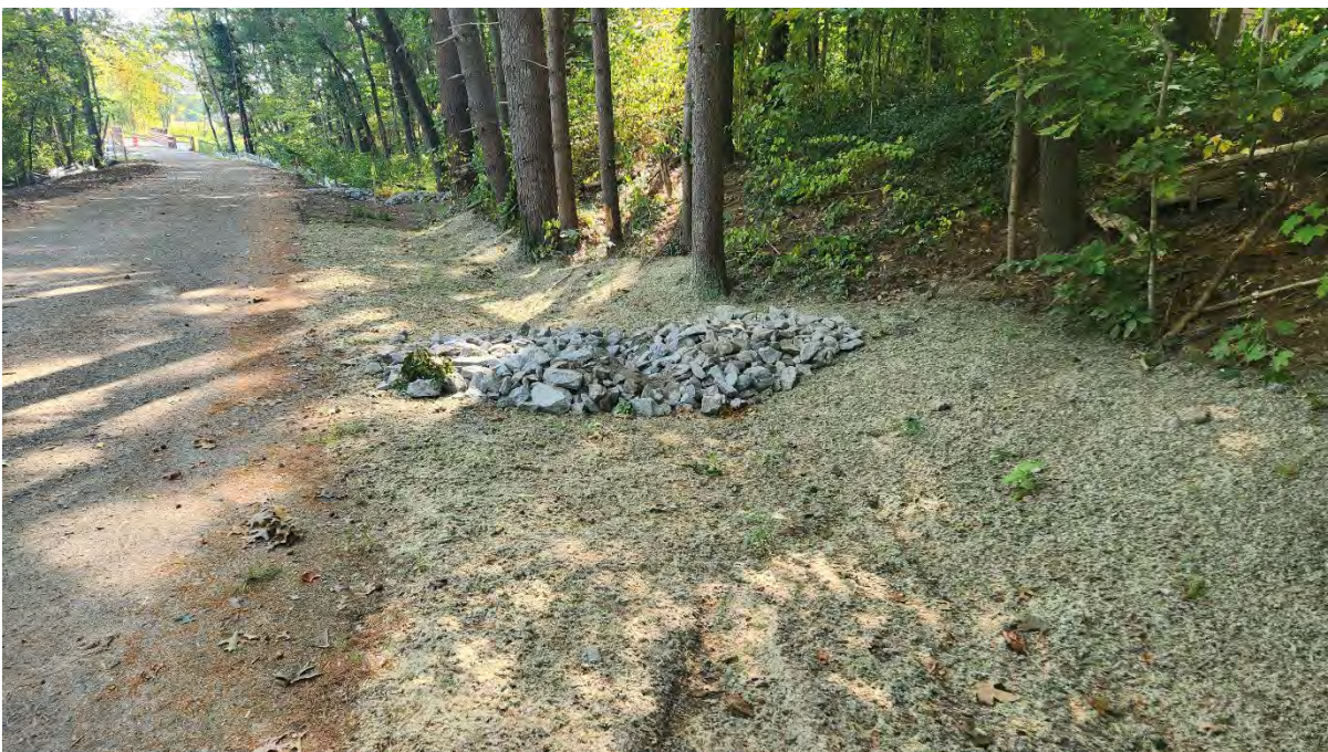
Photo 9: Installed check dam along segment 13. Photo taken on 9/16/24.
