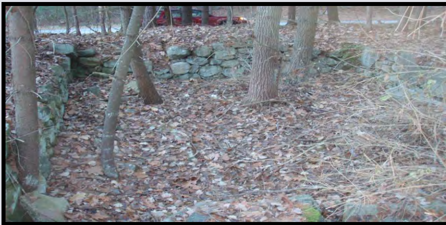
House foundation, near Nashoba Brook, North Acton
