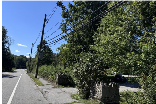
Route 20 where the existing sidewalk ends, looking westbound. The fragmented paved edge is constrained by driveways, stone walls, vegetation, and utility poles.
