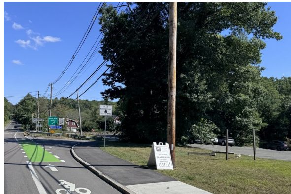
Route 20 approaching Hager Street, looking eastbound. Accessible curb ramp and short sidewalk/bicycle-lane segment; the facility does not continue through the corridor.
