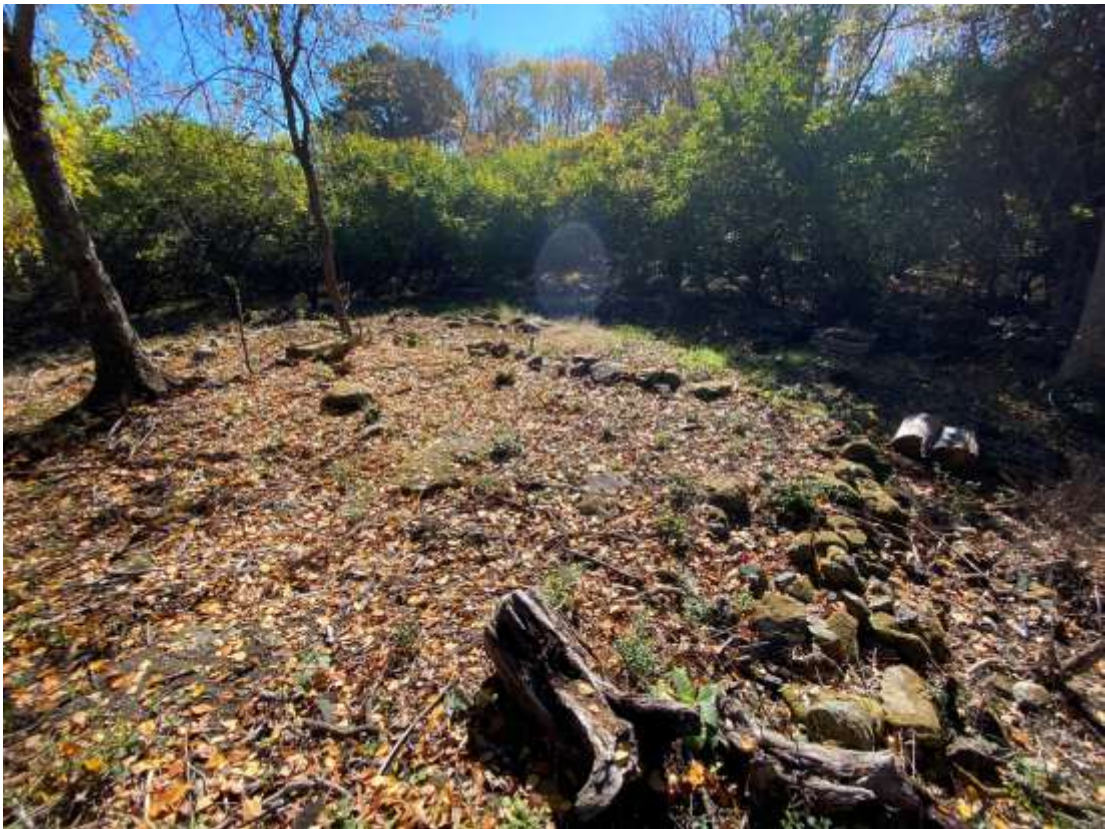
Photo 6: Foundation of the Barn
