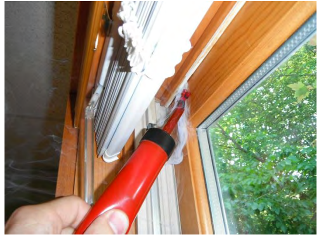
Windows – air leakage shown by smoke tracer testing at the perimeter of the upper sash of the compression jamb double hung window.
