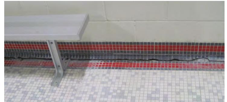
Figure 9 - Slab Settlement Near Diving Pool
