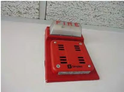
Figure 42 - Fire Alarm Horn Strobe
