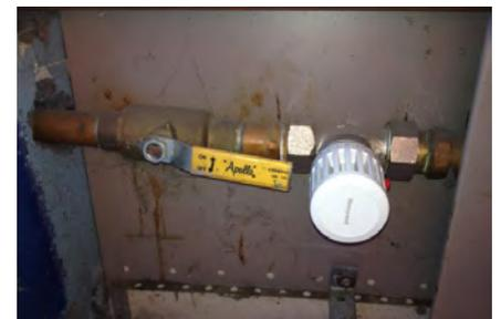
Figure 6 - Replaced Heating Valve
