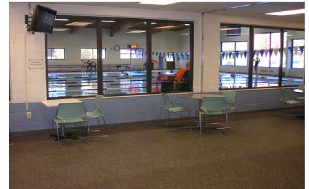
Fairbank Wing: The original glazed masonry units are visible in the corridor and some of the individual spaces. The wall surface above the glazed masonry is painted CMU. Walls separating program space are painted CMU. A small section of wood wainscoting was installed in the Teen Center lobby area.
