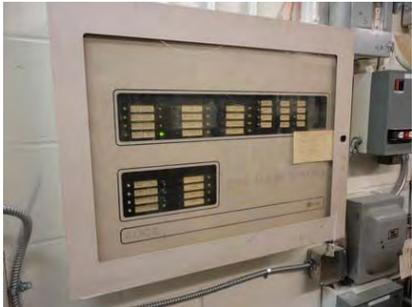
Figure 40 - Fire Alarm Control Panel - Closed
