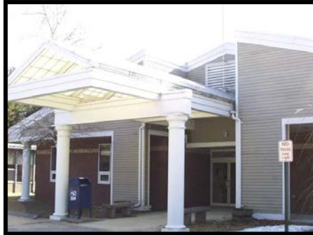
Sudbury Senior Center at the Fairbank Community Building
