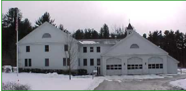
Sudbury Fire Headquarters
