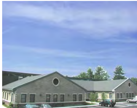
Public Works Building
