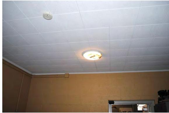
The lighting seems inadequate in general and the light fixtures are in poor condition. Refer to the electrical section of this report for more information.
