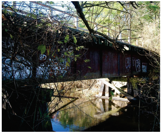
Modifications to Bridge #128
