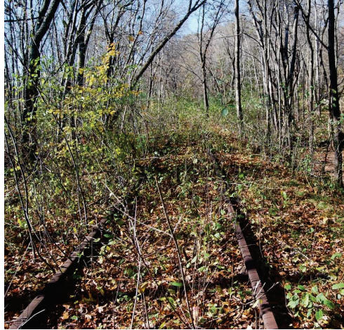
Removal rails and wood ties
