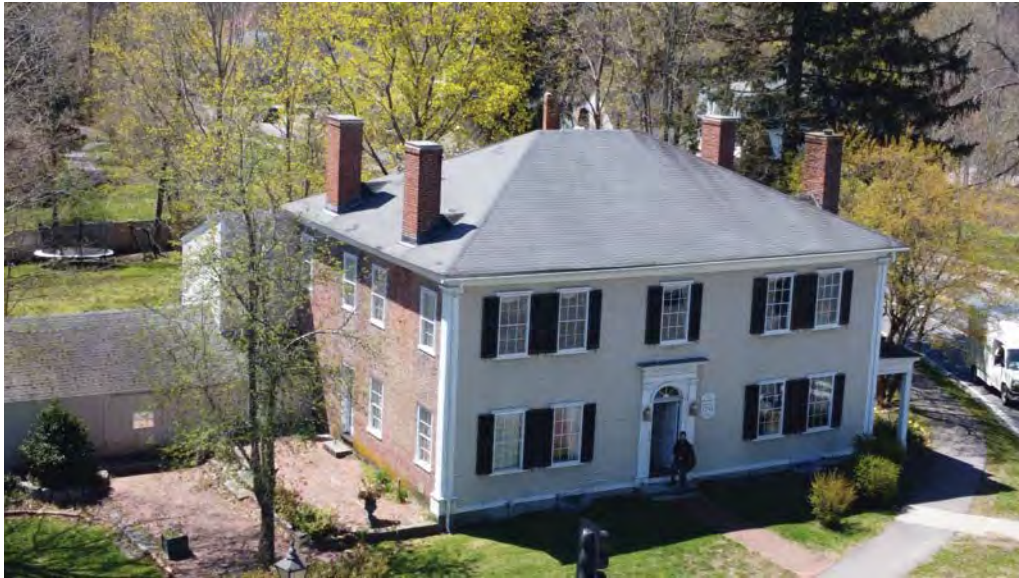
Figure 4.6-2 The main roof of the Hosmer House is a moderately pitched hip roof, finished with asphalt shingles.
