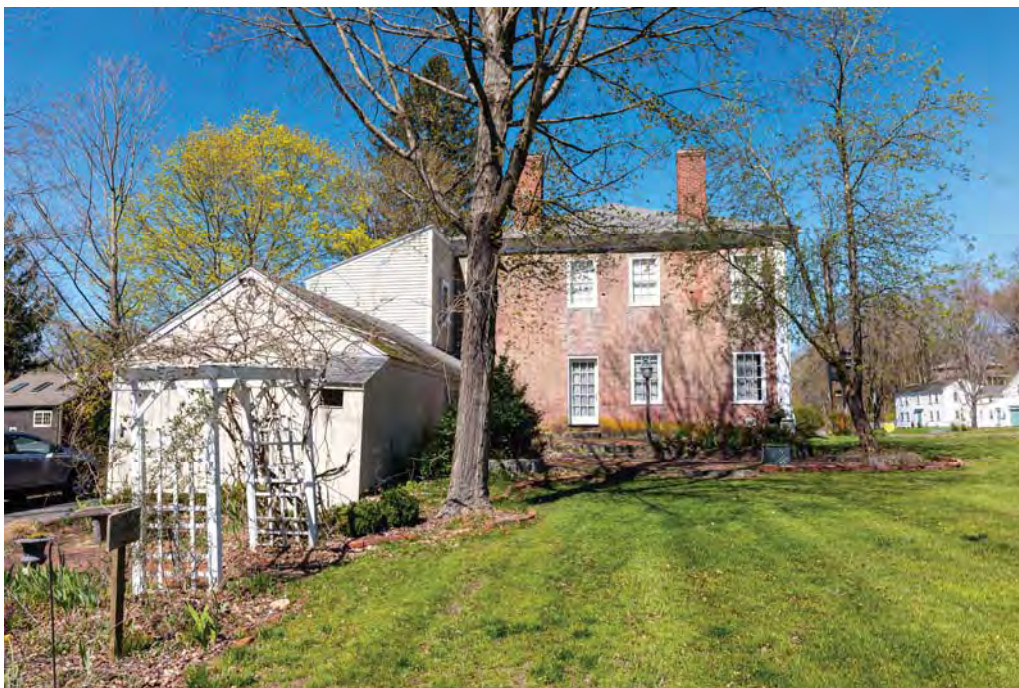
Figure 1.6-3 Date: 2024 Source: APS Hosmer House east elevation
