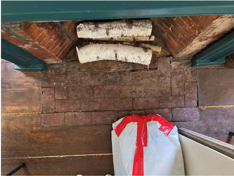
Figure 4.12-6 Standard bricks used to build the fireplace hearth in S-09.
