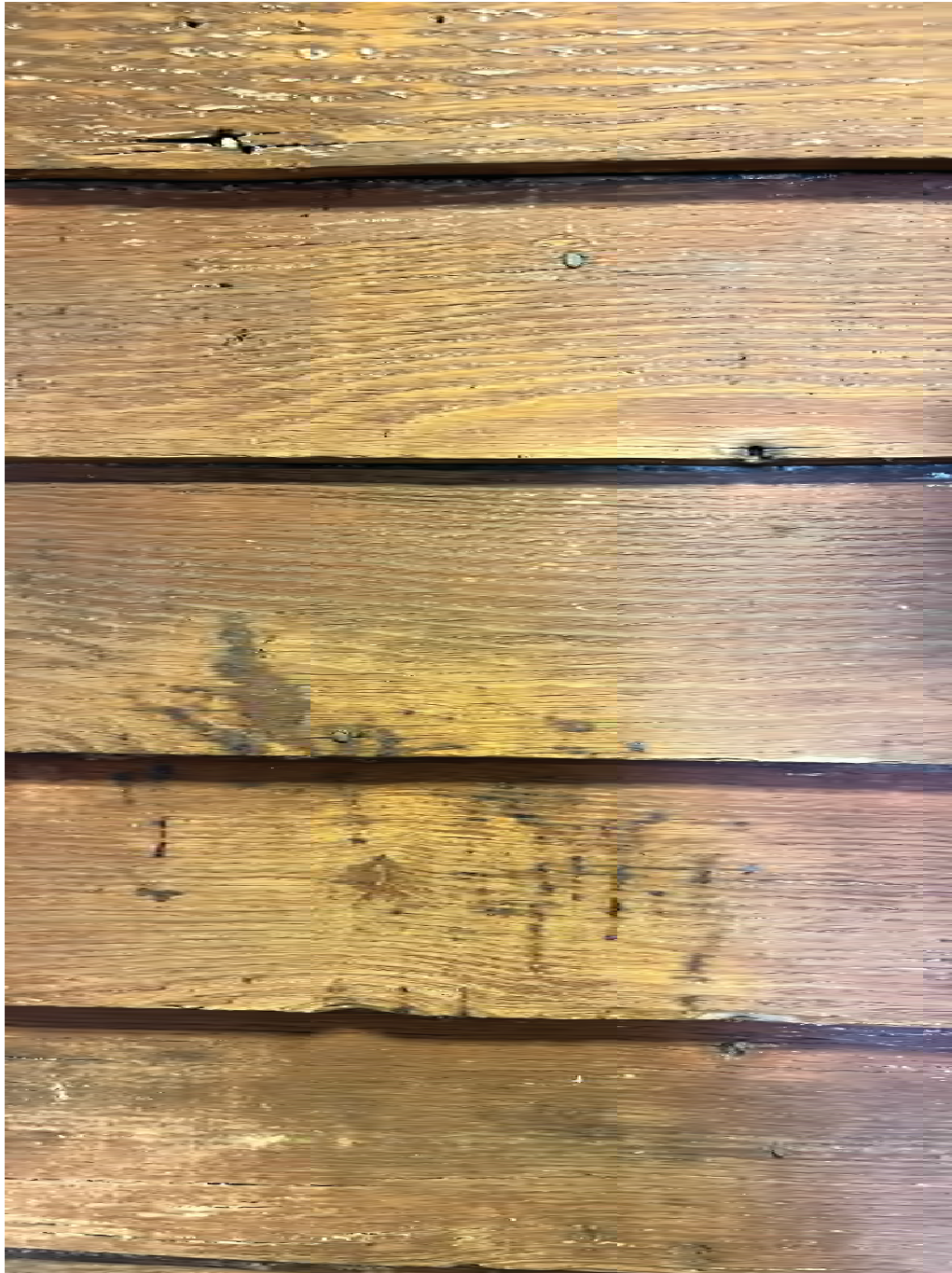
Figure 4.10-20 Wall finish of room F-07, which currently houses the SHC.
