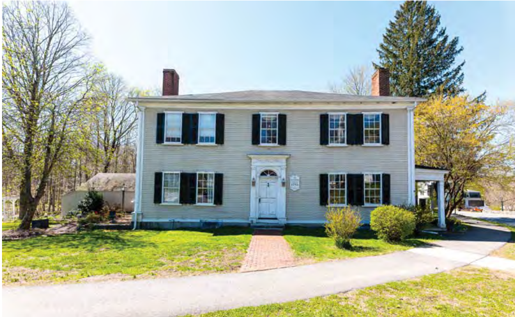
Figure 1.6-2 Date: 2024 Source: APS Hosmer House north elevation
