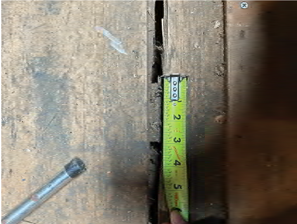
Figure 8.2-12 Attic floor framing.
