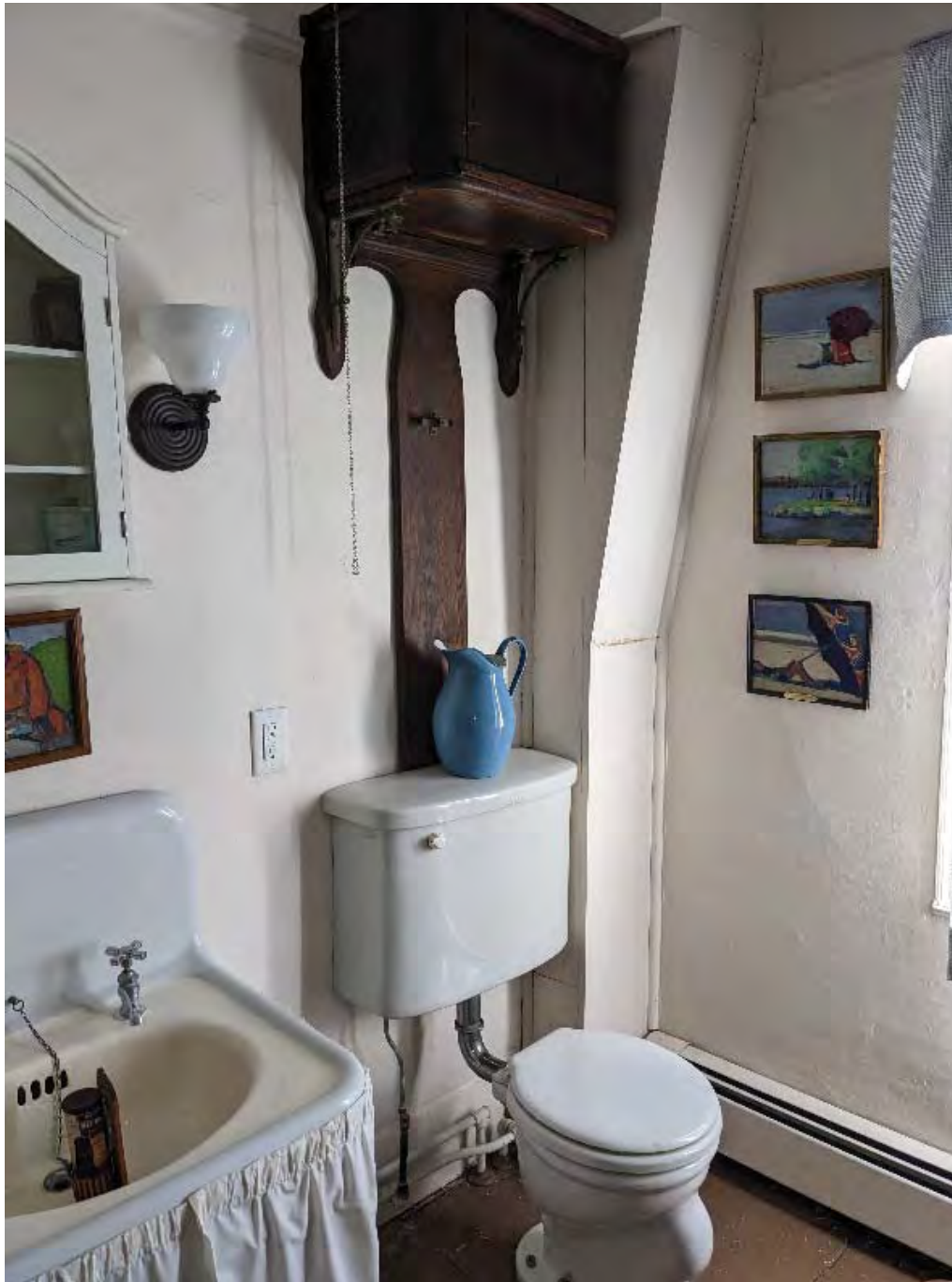
Figure 9.8-1 GFCI receptacle located in the upstairs bathroom.
