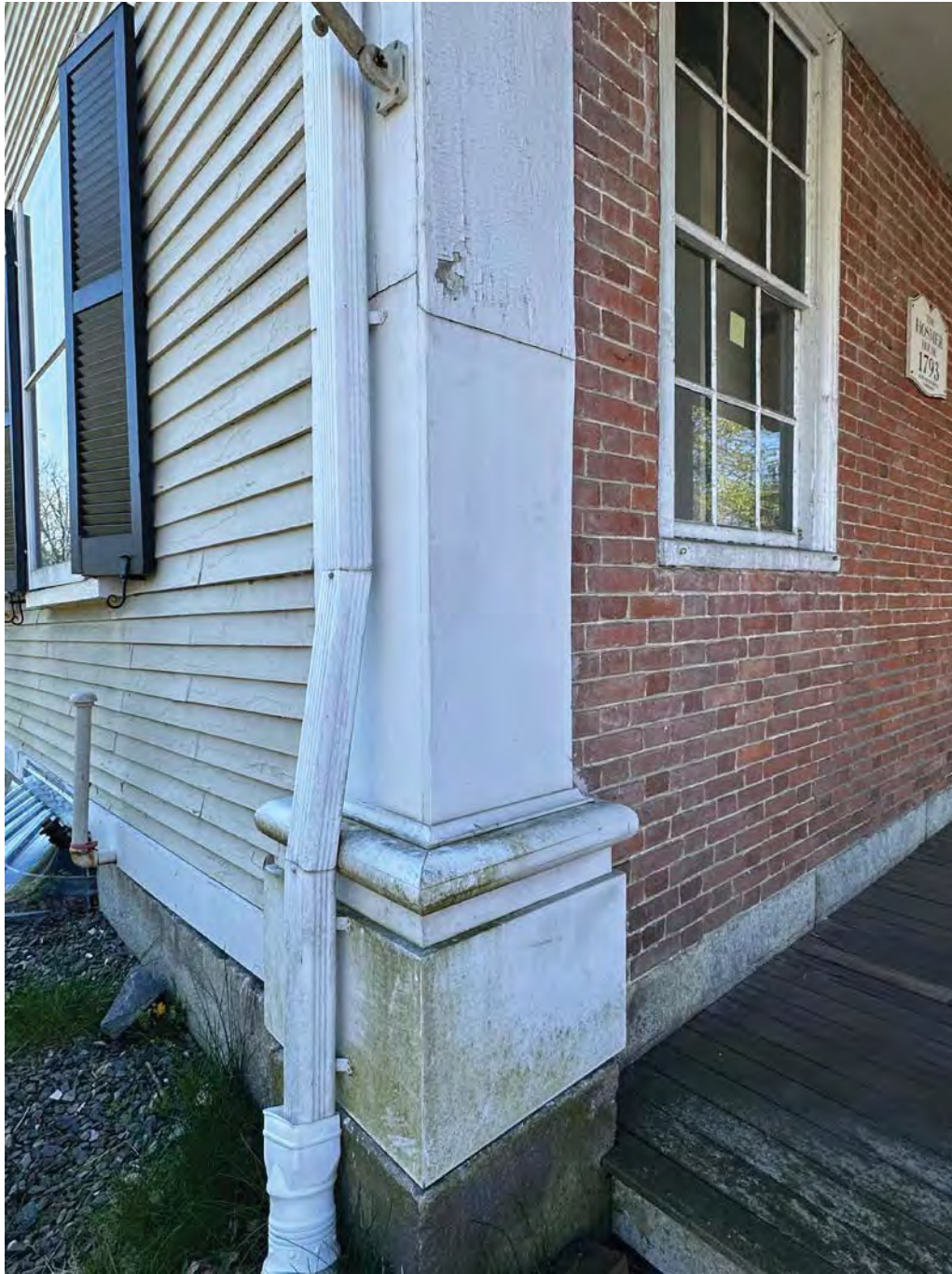
Figure 4.1-12 Bottom 3' of each pilaster shaft and both bases have been replaced.
