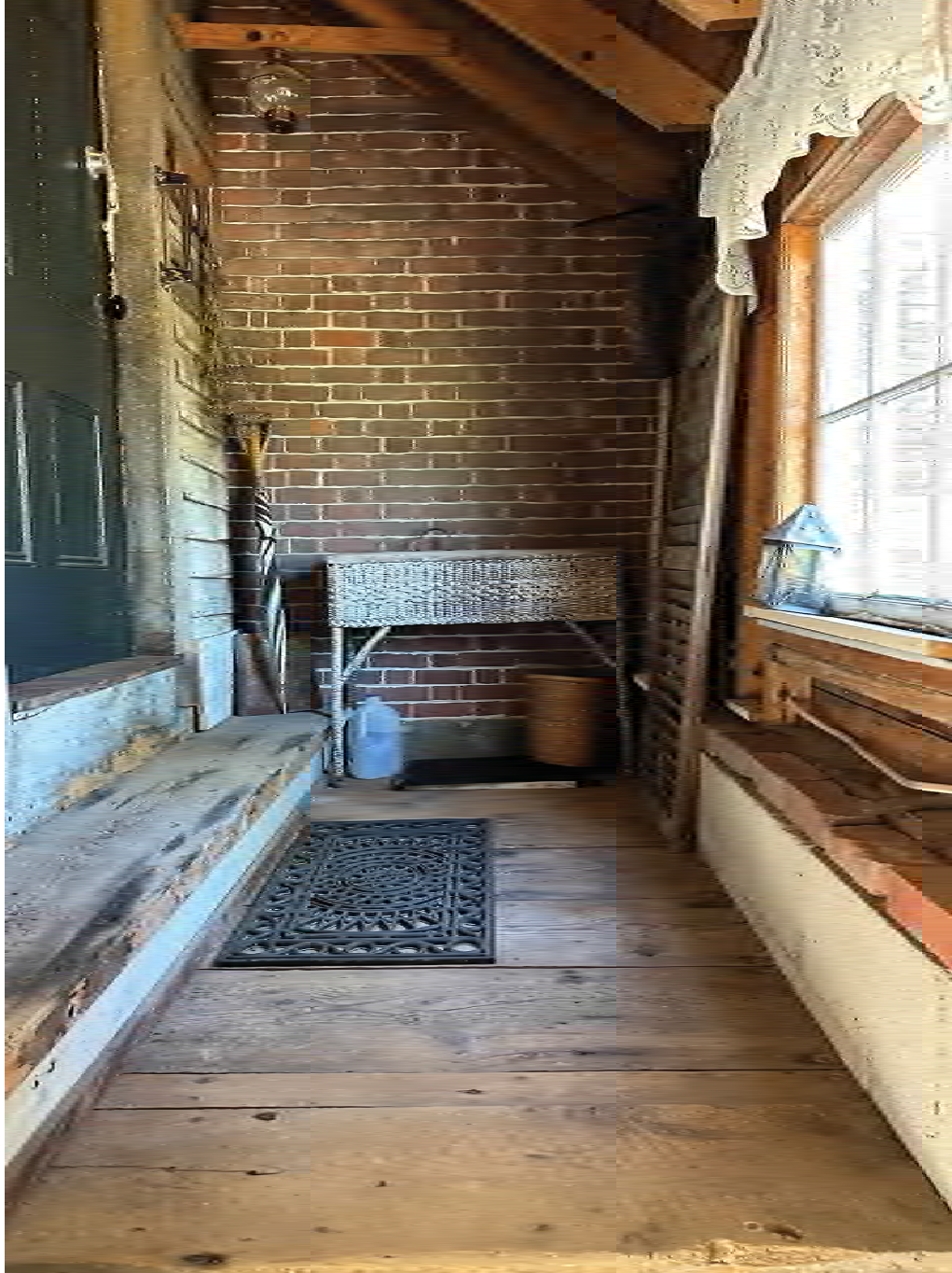
Figure 4.10-18 Interstitial space, which acts as a mudroom, between the open-air carriage house and room F-05, which currently houses the kitchen.
