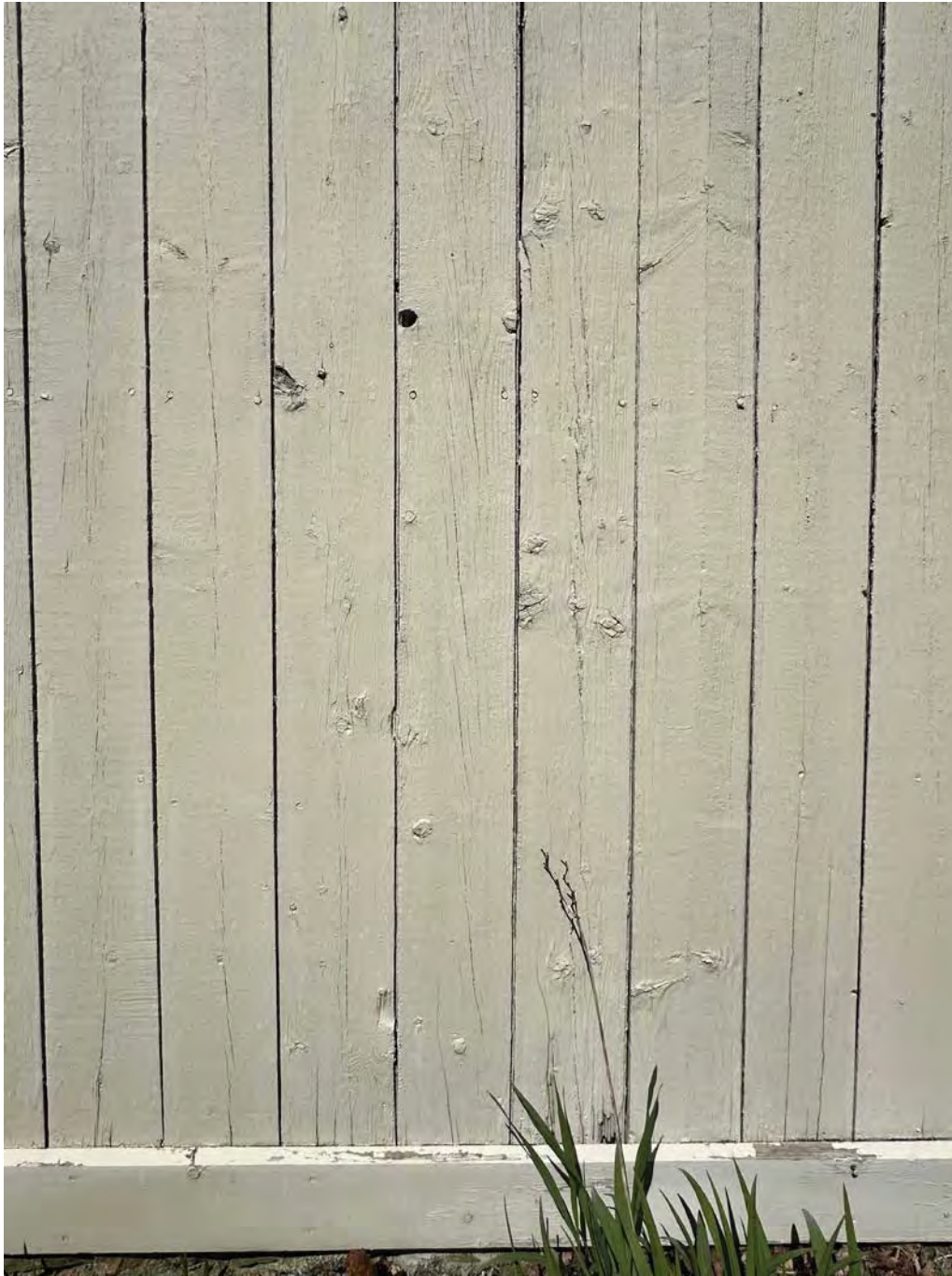
Figure 4.1-8 Vertical planks of carriage house with an average of 6-1/2" in width.
