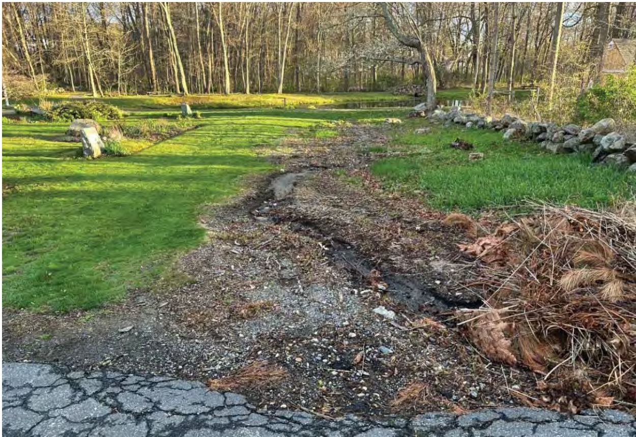
Figure 7.3-8 Soil washout and erosion extending downslope from the edge of the asphalt driveway and parking area. HL 2024.
