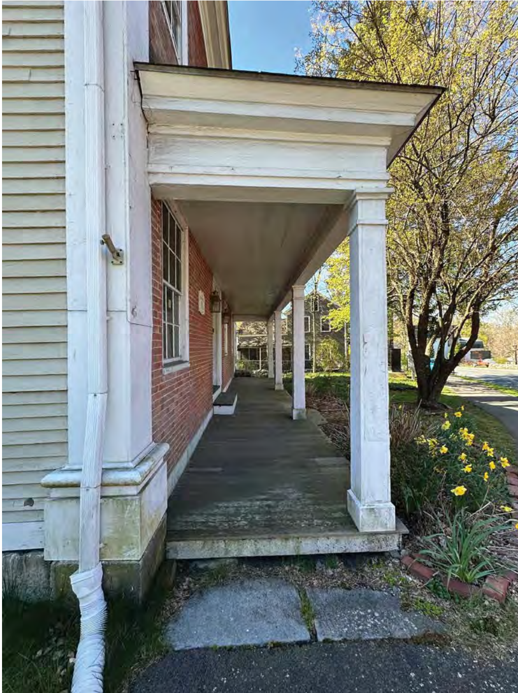
Figure 4.9-1 A single-story open porch extends along the entire length of the west elevation. It is constructed of a wood deck, wood columns and a shingled hip roof.
