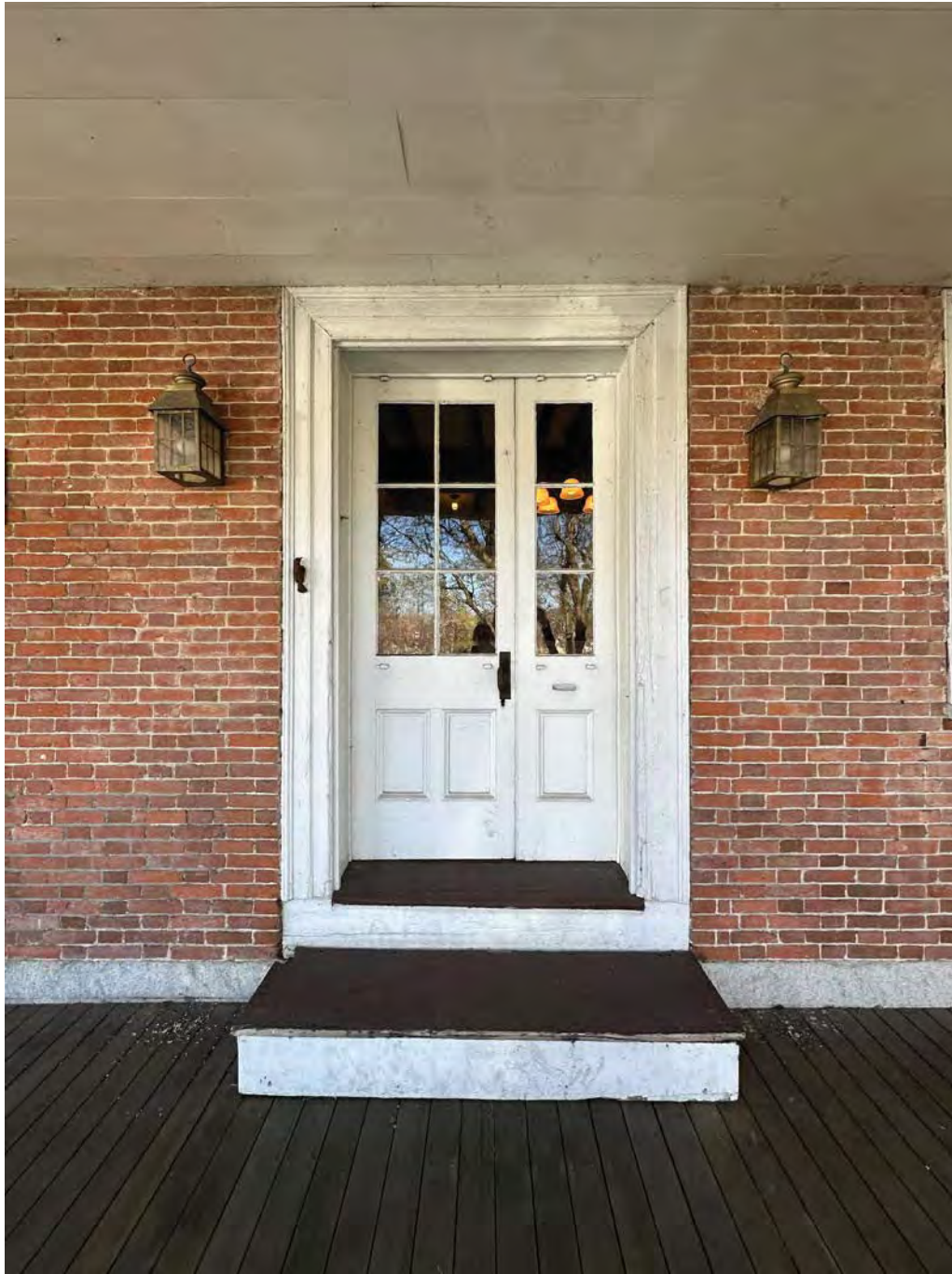
Figure 4.4-4 Throughout the house there are varying door configurations. Pictured here is D-22, a double door.
