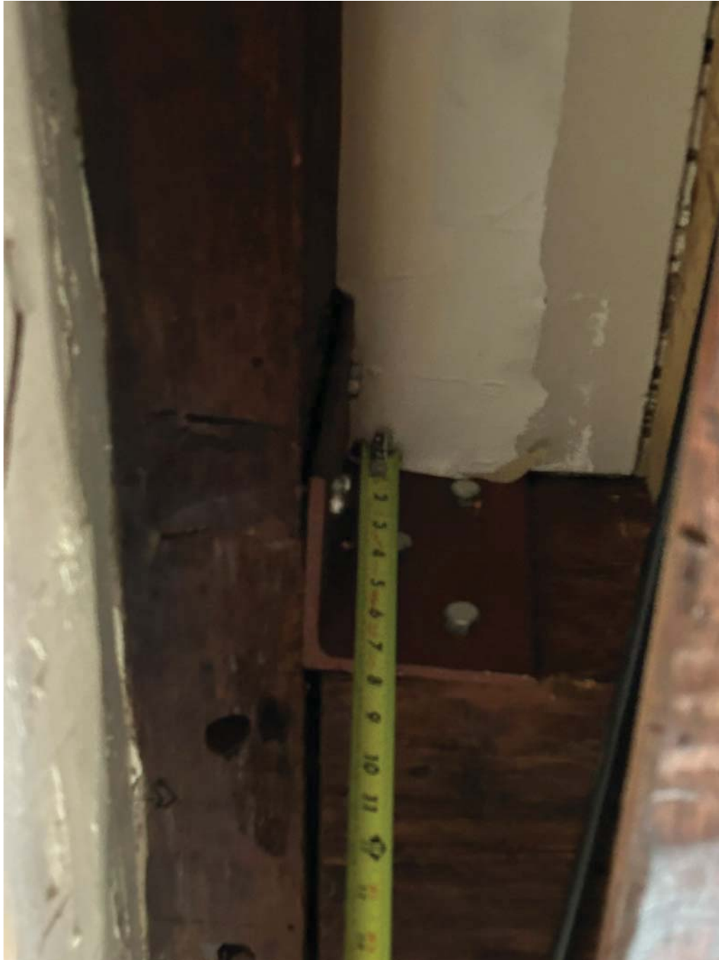
Figure 8.2-8 North end of high timber beam.
