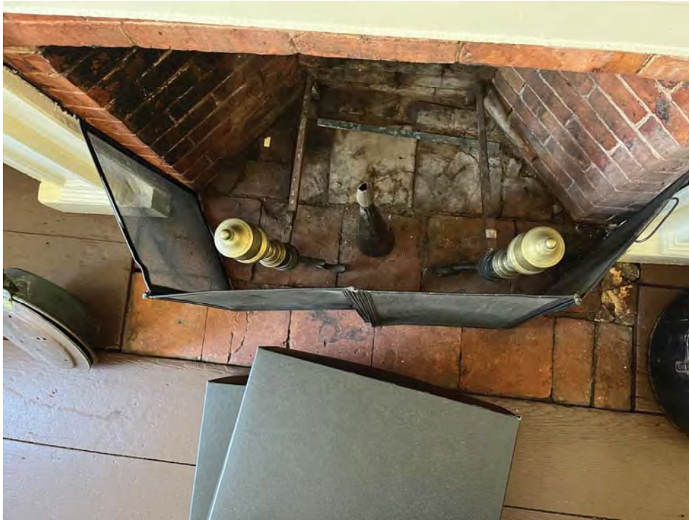
Figure 4.12-8 Standard square bricks used to build the fireplace hearth in S-02.
