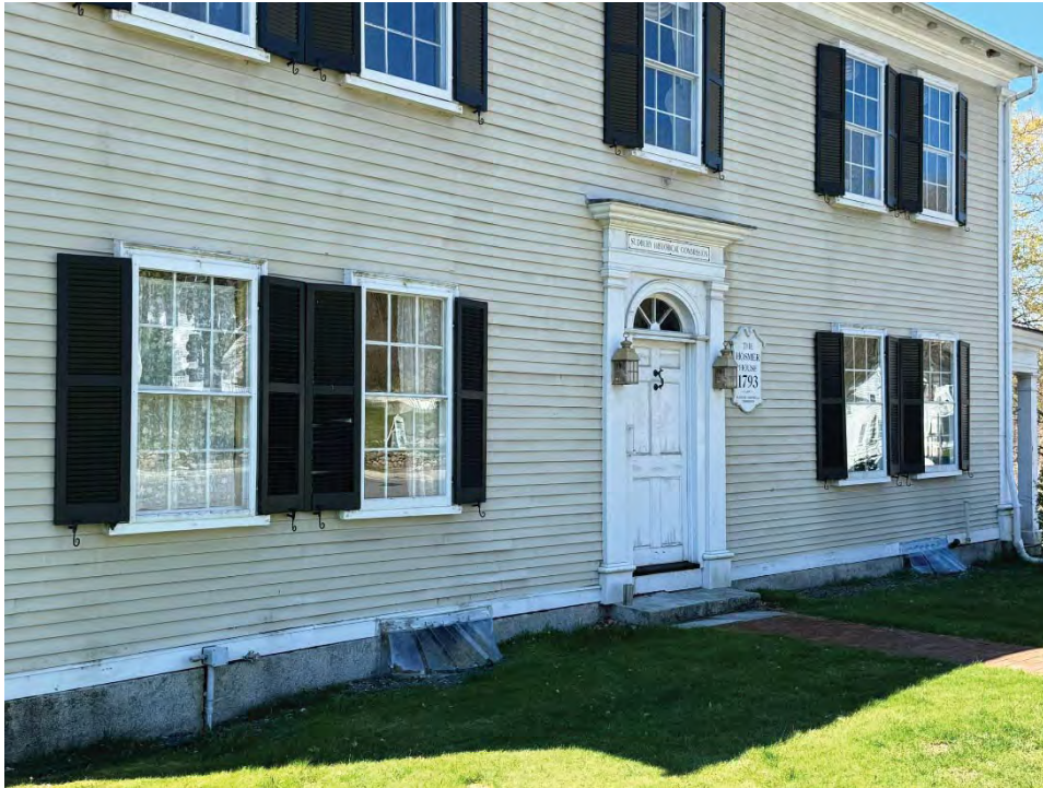
Figure 7.5-2b. Similar oblique view of the north façade shows no foundation plantings today. A thin strip of gravel divides the foundation from the lawn. HL 2024.
