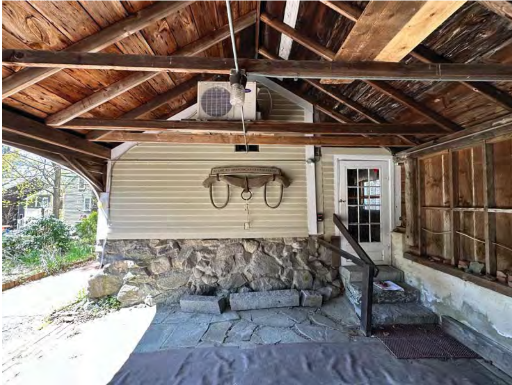
Figure 4.3-7 Ashlar foundation wall shared by the east wall of the southeast addition, and the carriage house.
