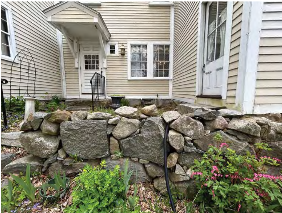
Figure 8.3-21 Rubble stone masonry retaining wall at south entry.
