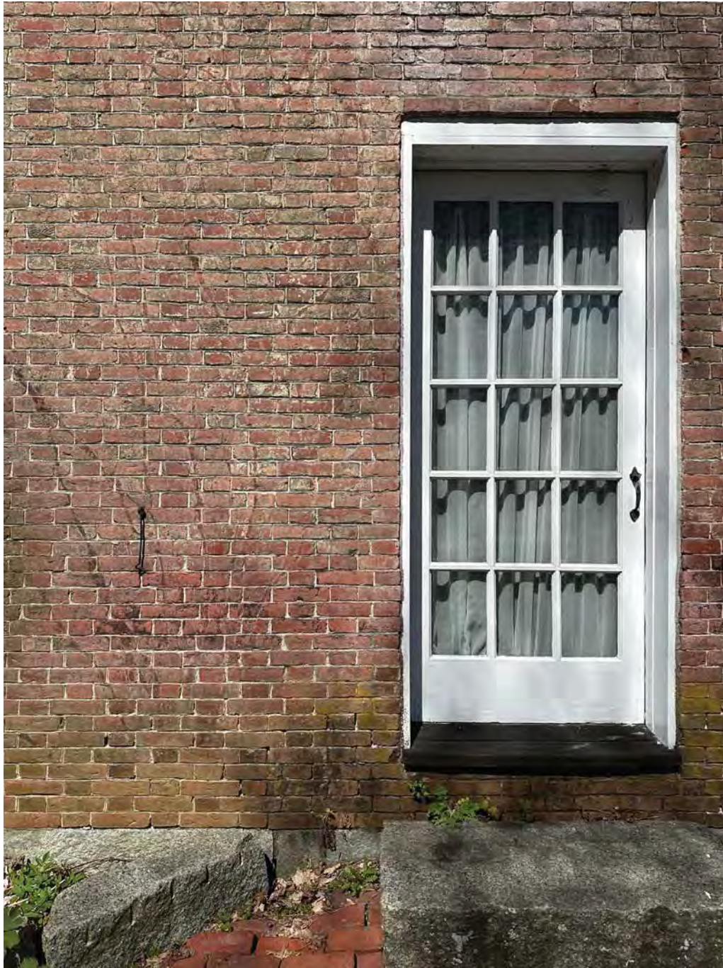
Figure 4.4-5 D-06 is a new tempered glass door.
