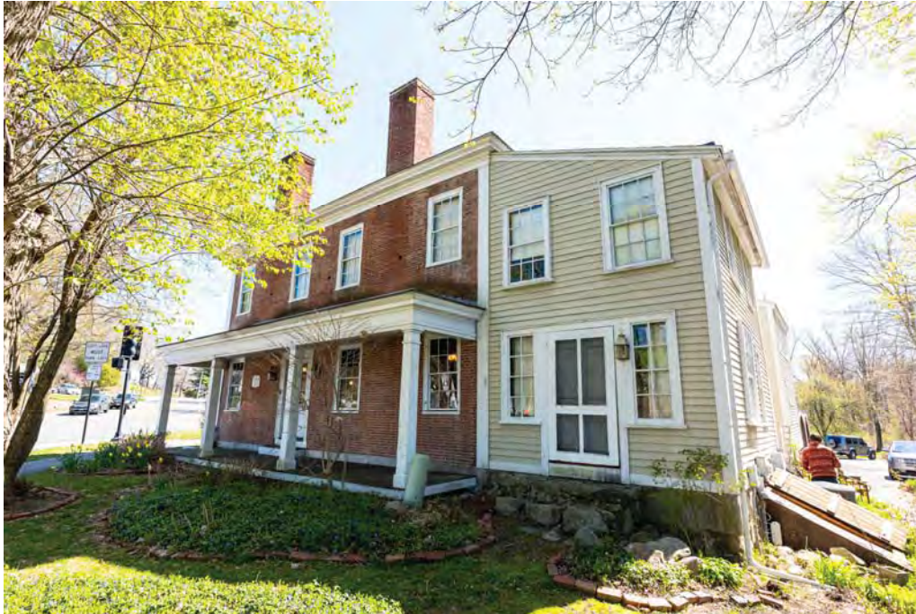
Figure 1.6-6 Date: 2024 Source: APS Hosmer House west elevation
