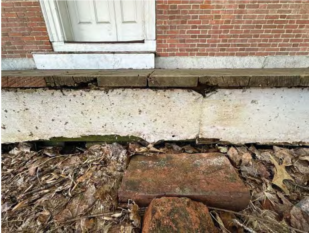
Figure 4.9-2 There is extensive mildew and mold on the deck fascia, most likely due to its proximity to the earth and surrounding vegetation and the section of fascia between the second and third columns is rotted through, the wood is cracked, and a portion of the fascia has fallen off.
