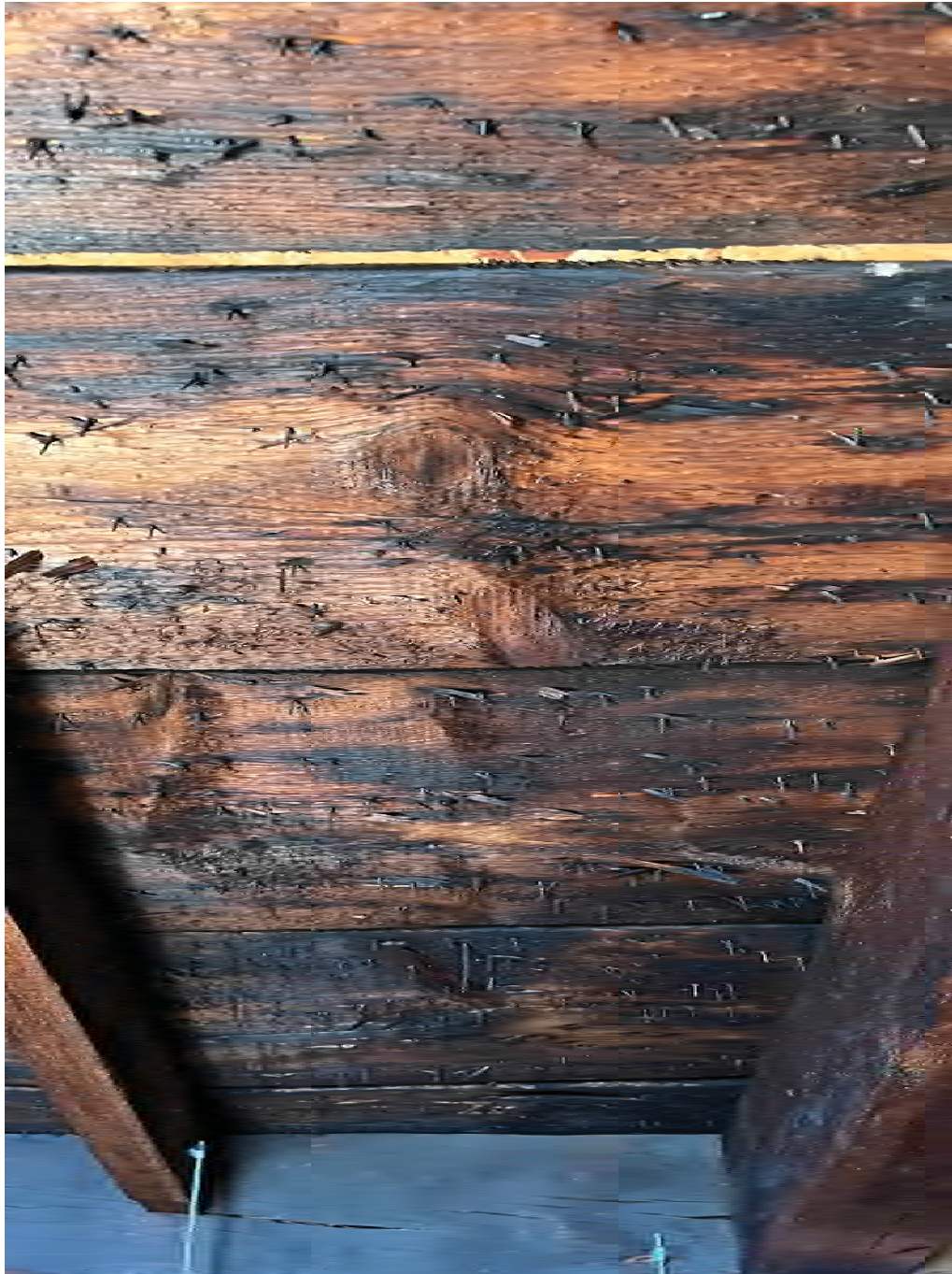
Figure 4.10-23 Roof sheathing of the main roof.
