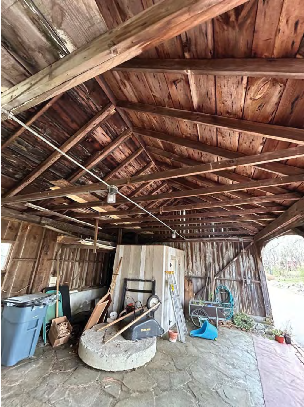
Figure 8.2-15 Carriage house roof framing.
