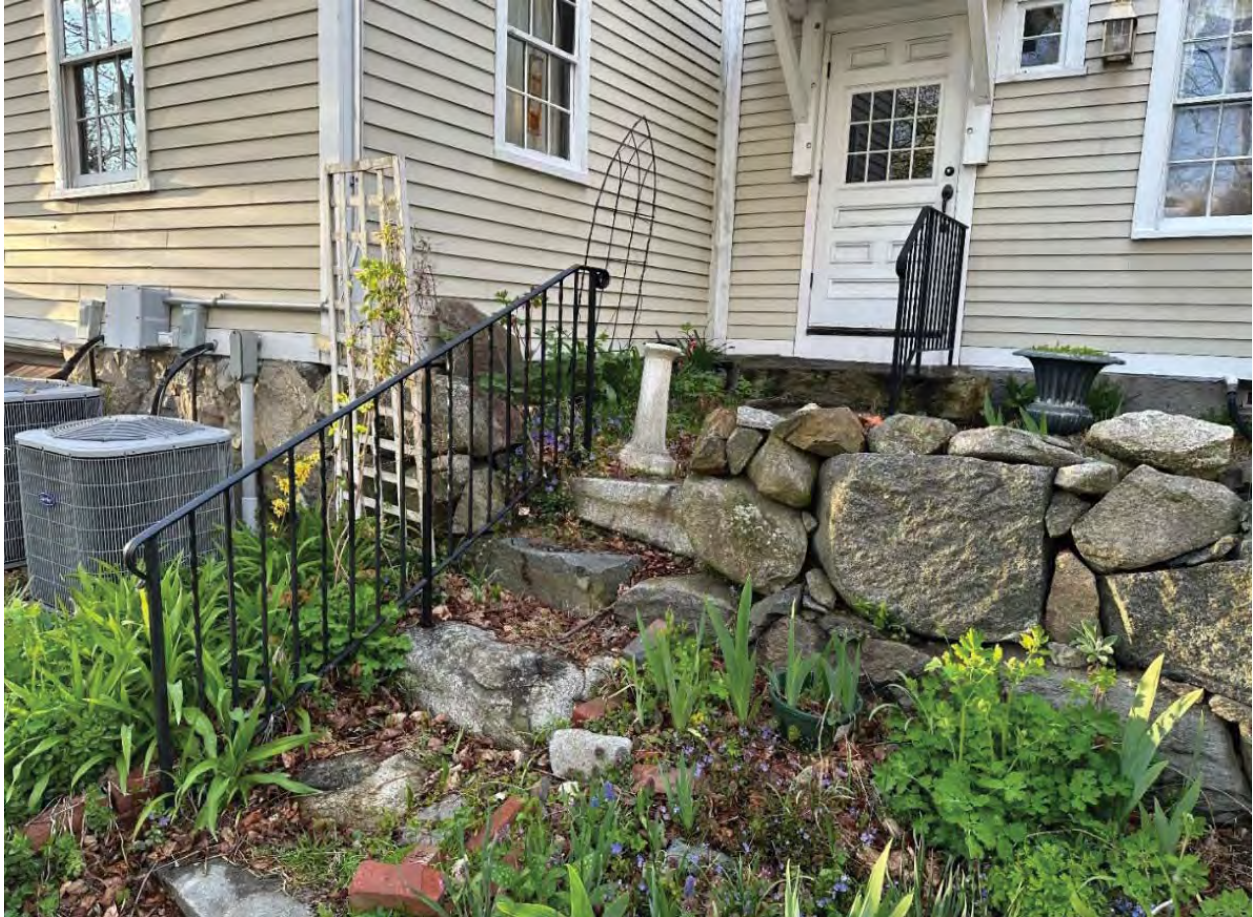
Figure 7.3-22 Two sets of irregular stone steps with metal railings, descend from the raised south façade door to a paved courtyard, and proceed down varied stone steps. A dry stone and boulder retaining wall holds the grade along the courtyard edge. HL 2024.
