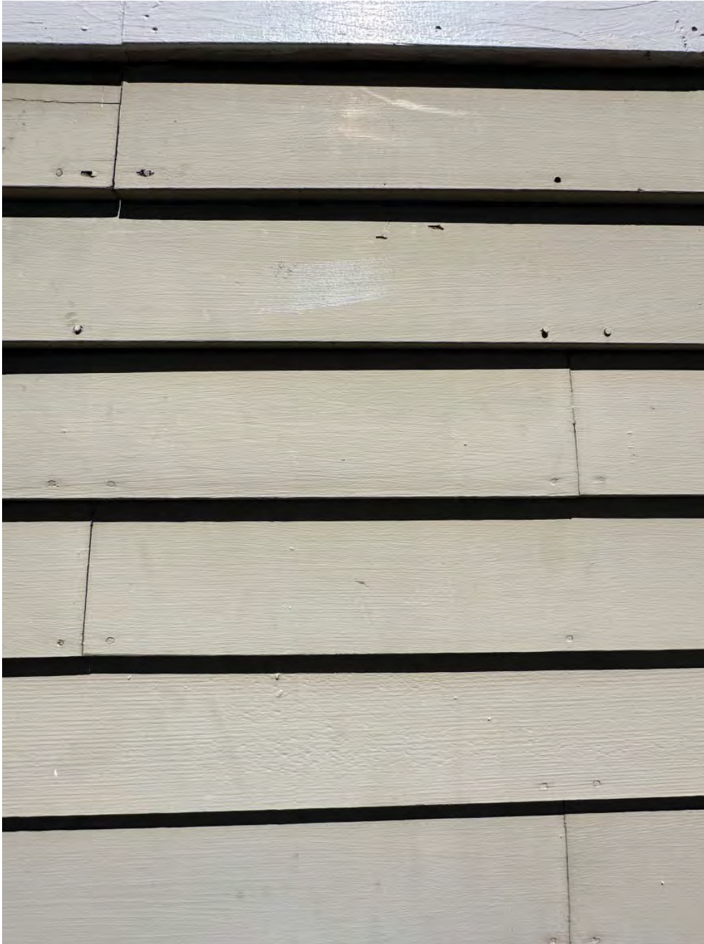
Figure 4.1-3 Butted-up laps to fasten the siding.
