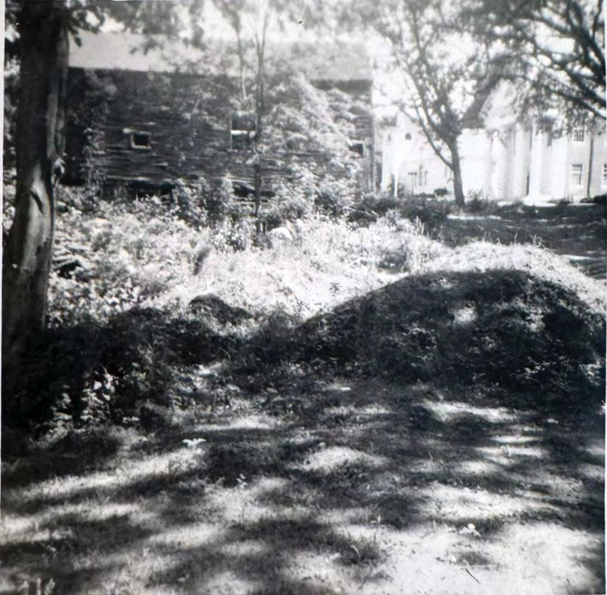
Figure 7.2-57. This 1975 north-facing photograph of the Barn, with deteriorated siding evident, and landscape captures an overgrown area of volunteer vegetation on the south side of the barn, with a pile on the right side of the image. Deciduous tree canopy overhead creates dappled light patterns on the ground. In the background, the Town Hall white columns and brick façade appears across the street. Courtesy Hosmer House Collections.
