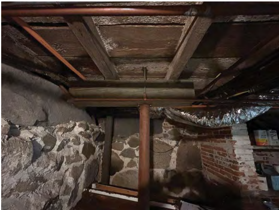
Figure 8.2-3 Southeast corner of floor framing with supplemental dropped beam and post.
