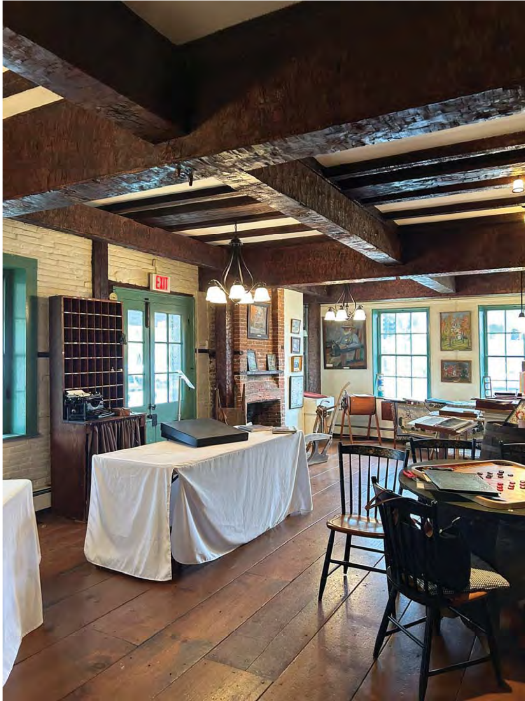
Figure 8.3-18 Ballroom floor framing.
