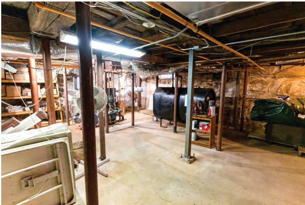
Figure 4.11-1 Poured concrete floor of B-01.
