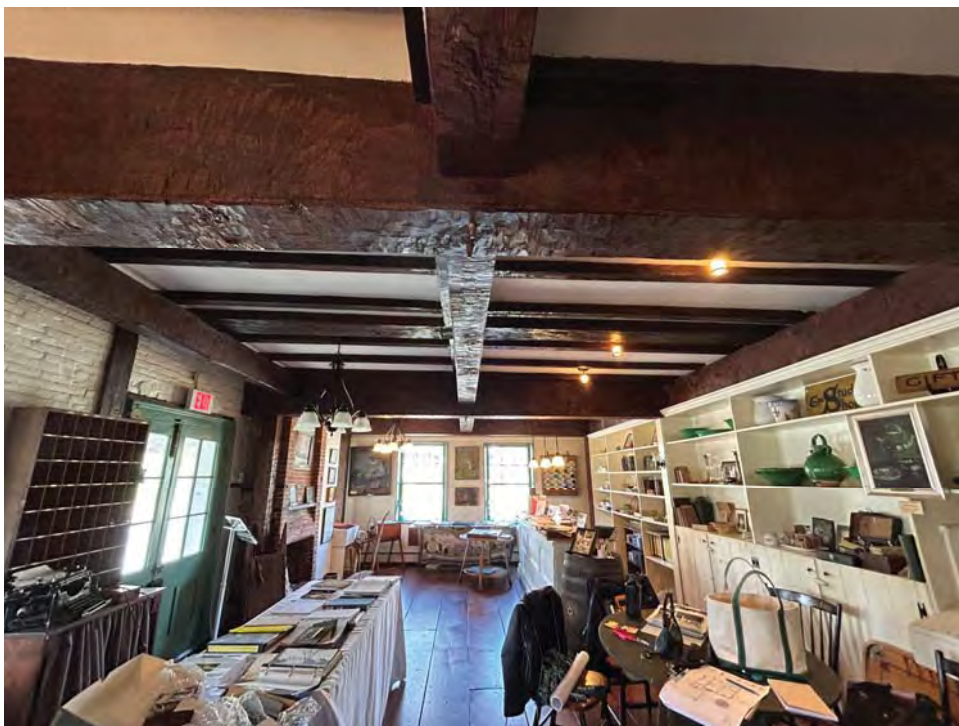
Figure 8.2-6 Dropped, wood clad steel beams in storeroom ceiling.
