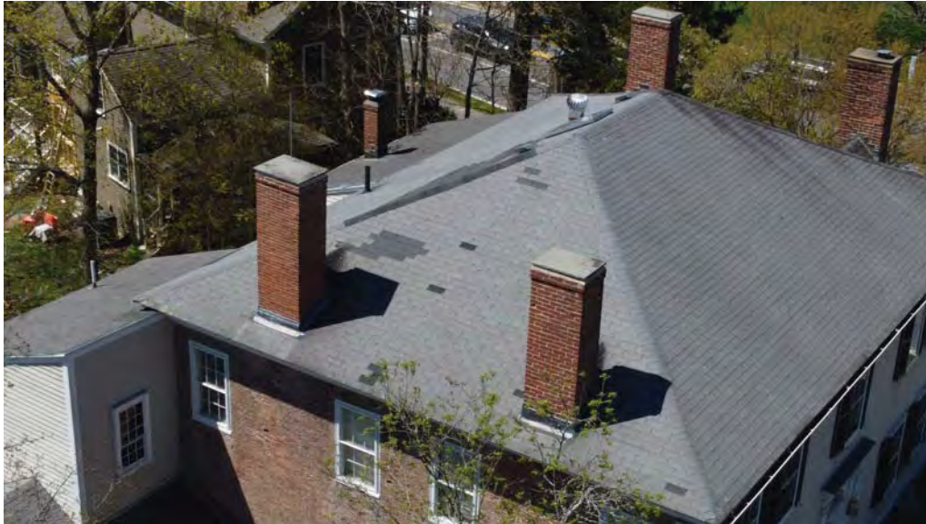
Figure 4.8-1 Four tall, brick-masonry chimneys are situated in pairs along the east and west elevations of the main house, slightly set back from the hipped roofline. The fifth chimney is located in the southwest addition.
