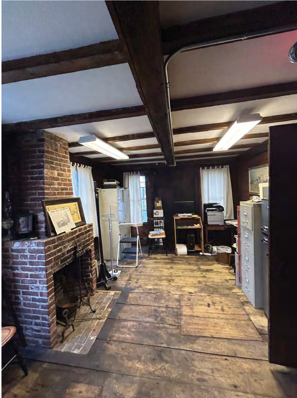
Figure 8.2-9 Dropped second floor framing above apartment/office addition.
