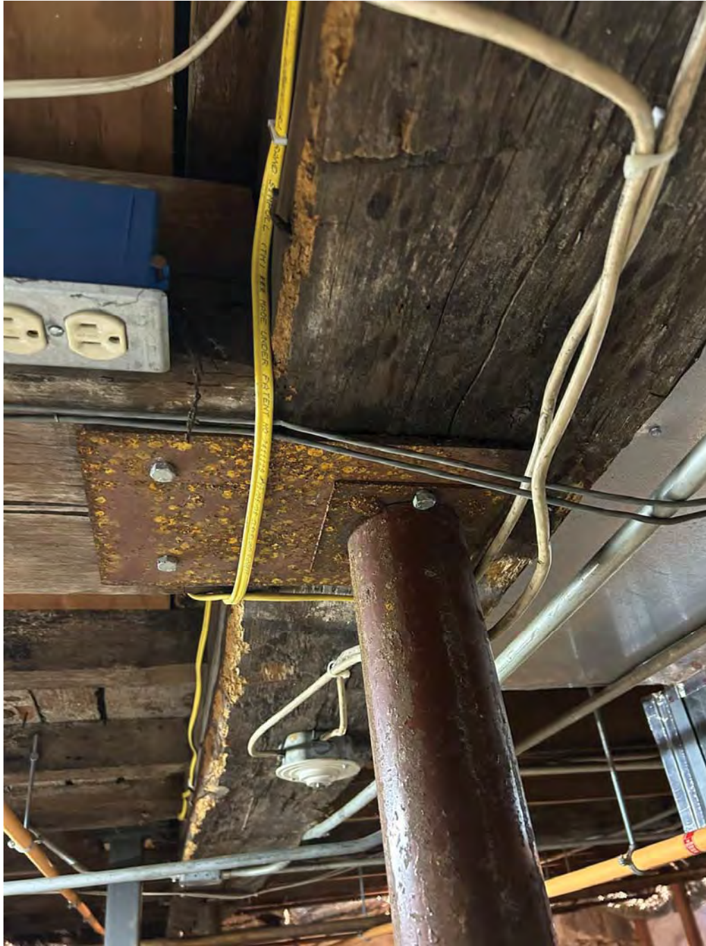
Figure 8.2-4 Central beam support at connecting transverse beam.
