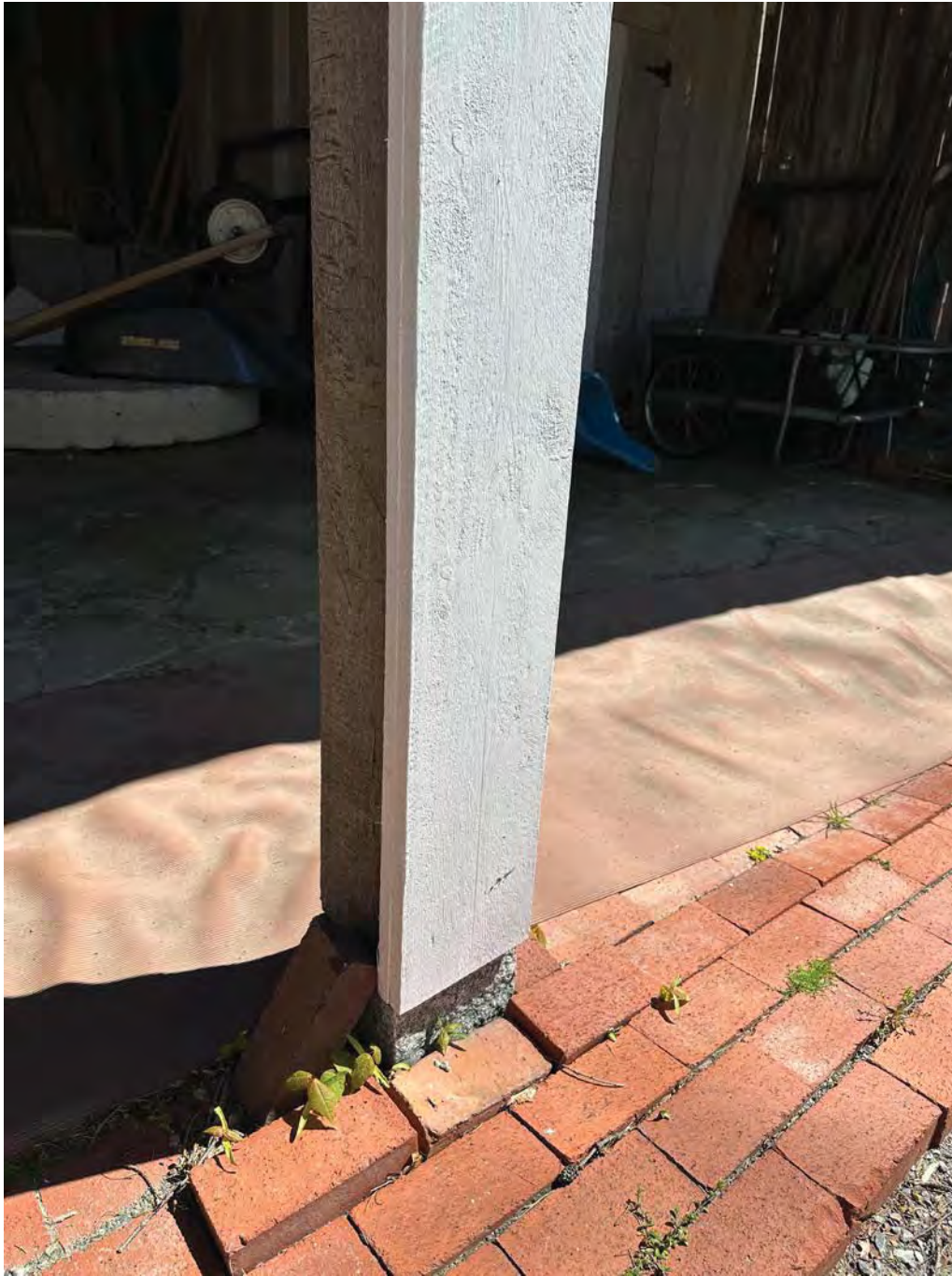
Figure 4.1-9 Carriage house column.
