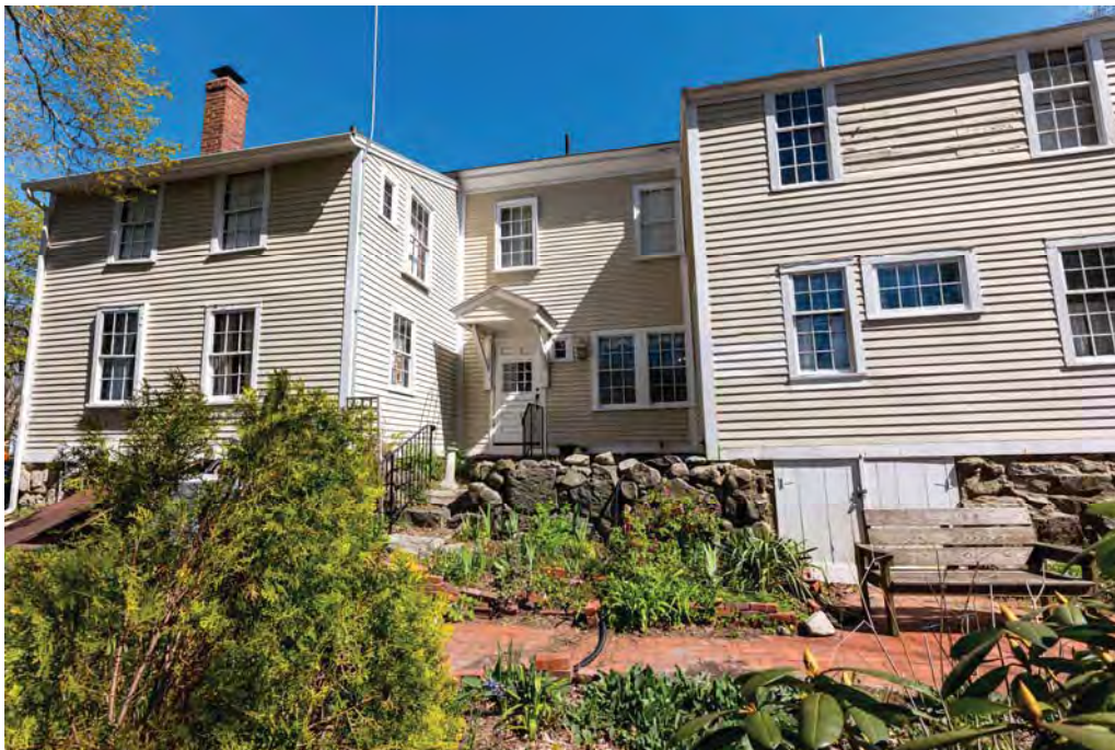
Figure 1.6-5 Date: 2024 Source: APS Hosmer House south elevation
