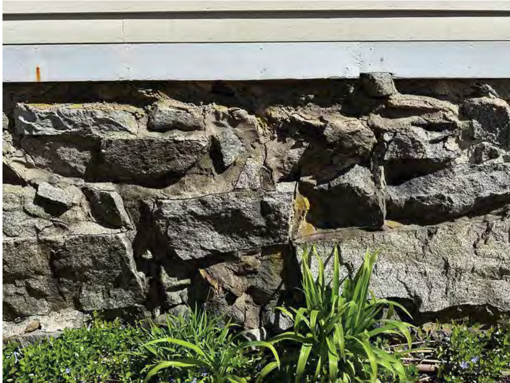
Figure 4.3-2 Foundation below rooms F-05 and F- 07 is constructed from ashlar masonry.
