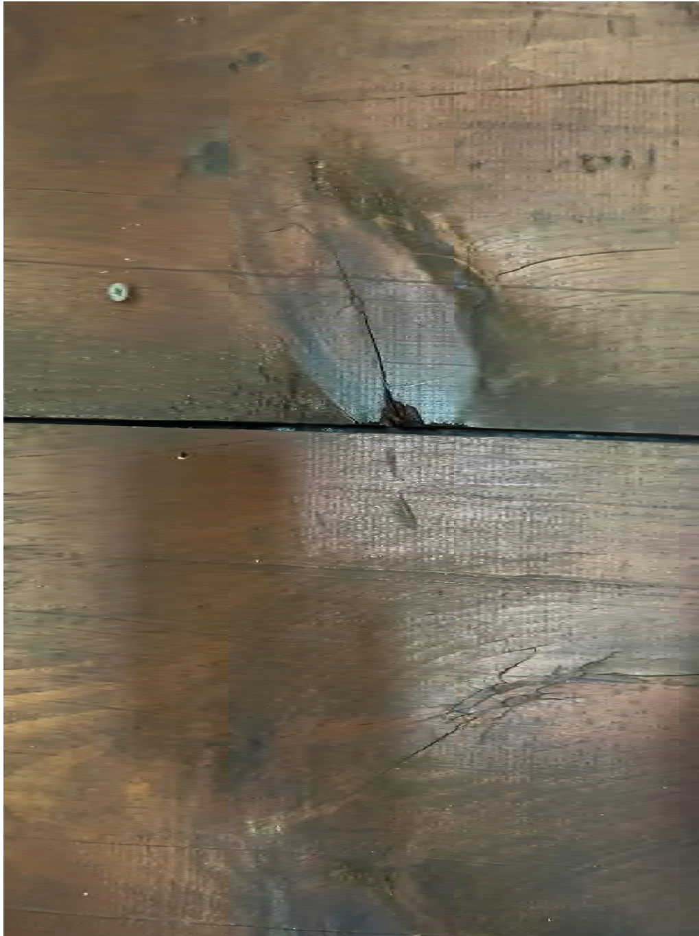
Figure 4.10-19 Wall finish of room F-07, which currently houses the SHC.
