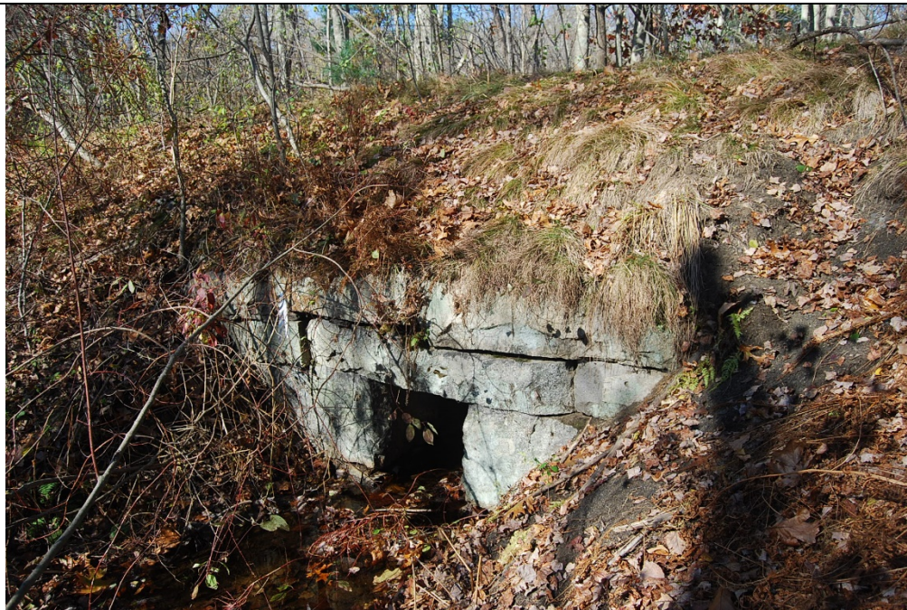
Culvert 126B. South elevation. View looking NW.
