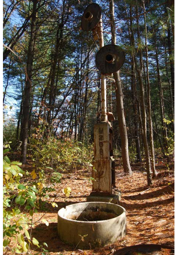
Signal M208 at MP 20.8. View looking E. Concrete battery well in foreground.
