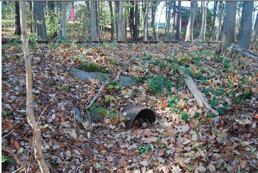
Culvert 127A. North elevation. View looking SW.
