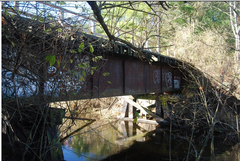
Bridge 128. (SUD.900) North elevation. View looking SW.
