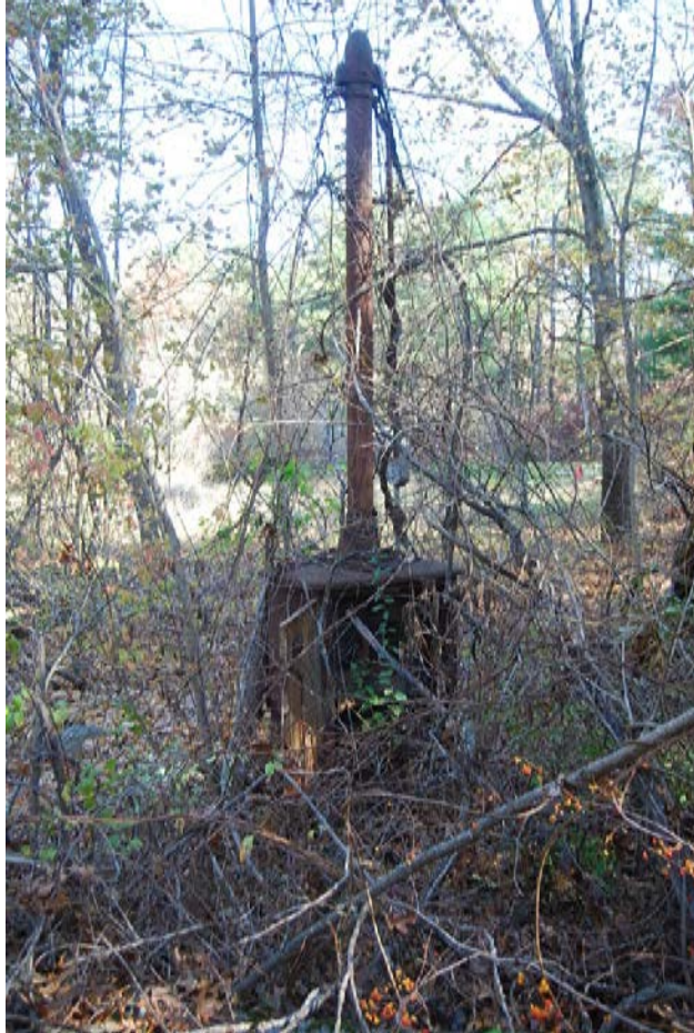
Auto Highway Flasher/ Signal Relay Box at MP 21.35 at NE corner of intersection of Peakham Road and ROW. View looking NE.
