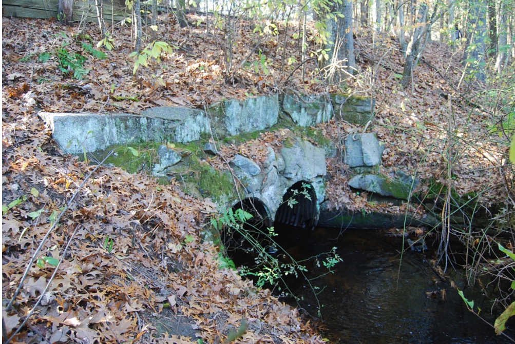
Culvert 127F. North elevation. View looking SW.
