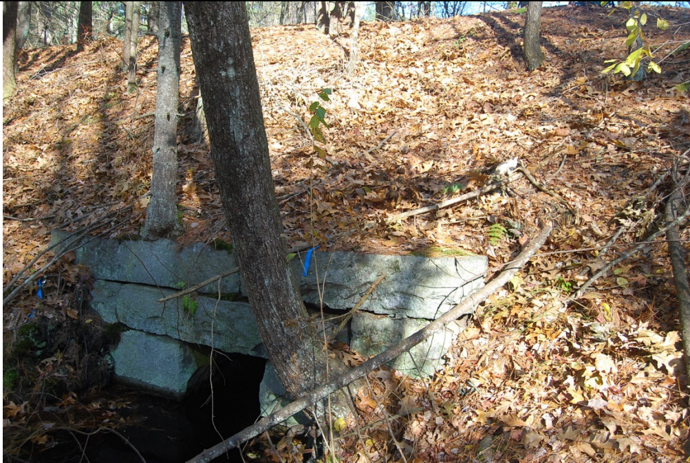
Culvert 127H. South elevation. View looking NW.
