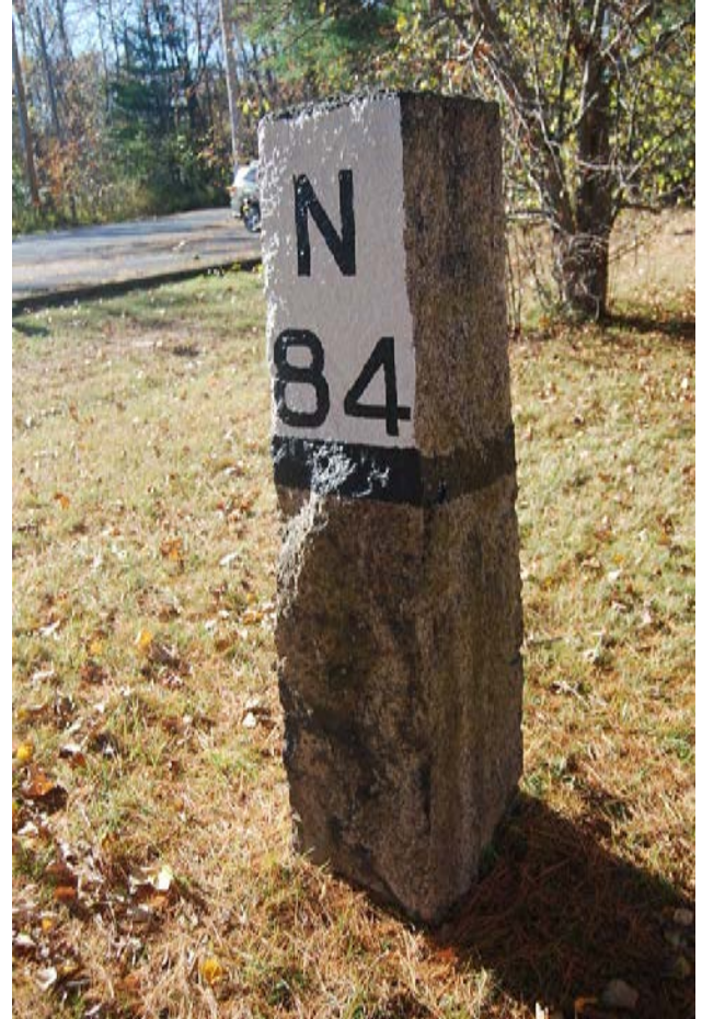
Milepost 20.0. East and north elevations. View looking SW.
