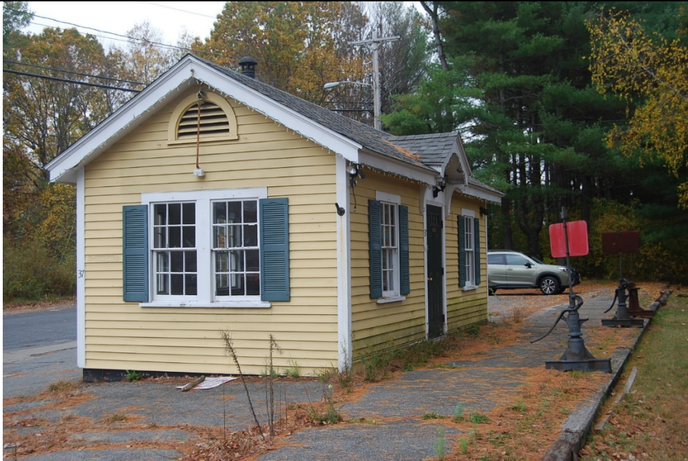
South Sudbury Station. View looking SW. Switchstands at platform edge.
