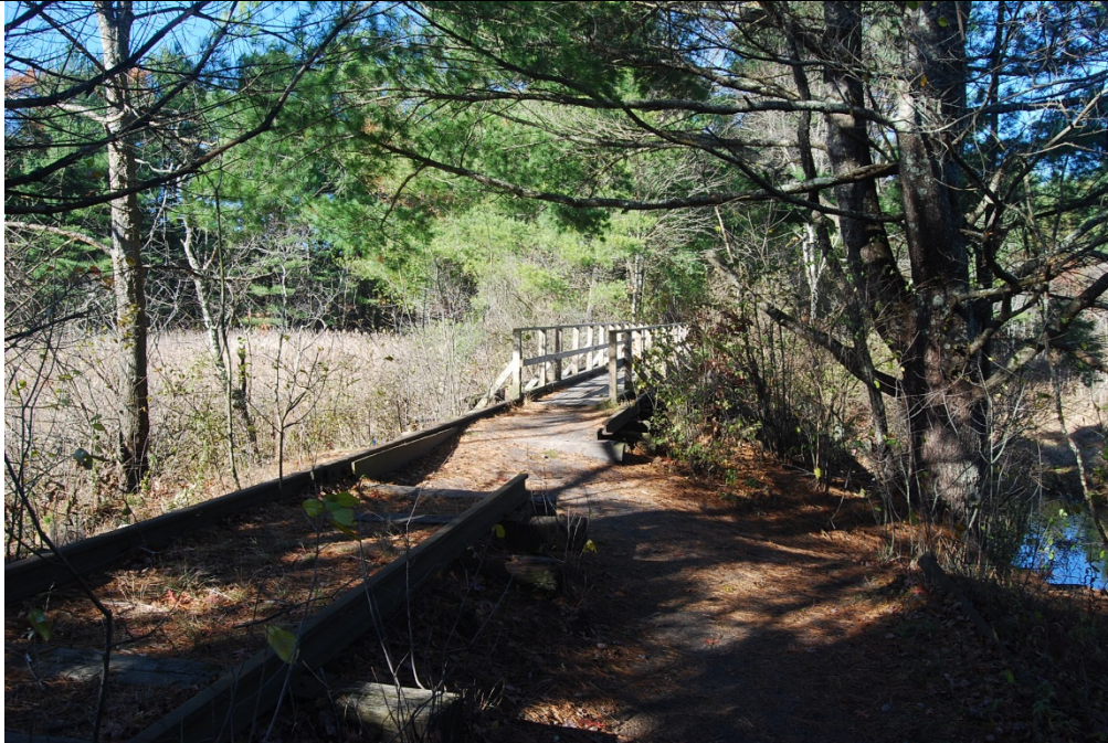
Railbed at east approach to Bridge 128, MP 22.24. View looking SW.
