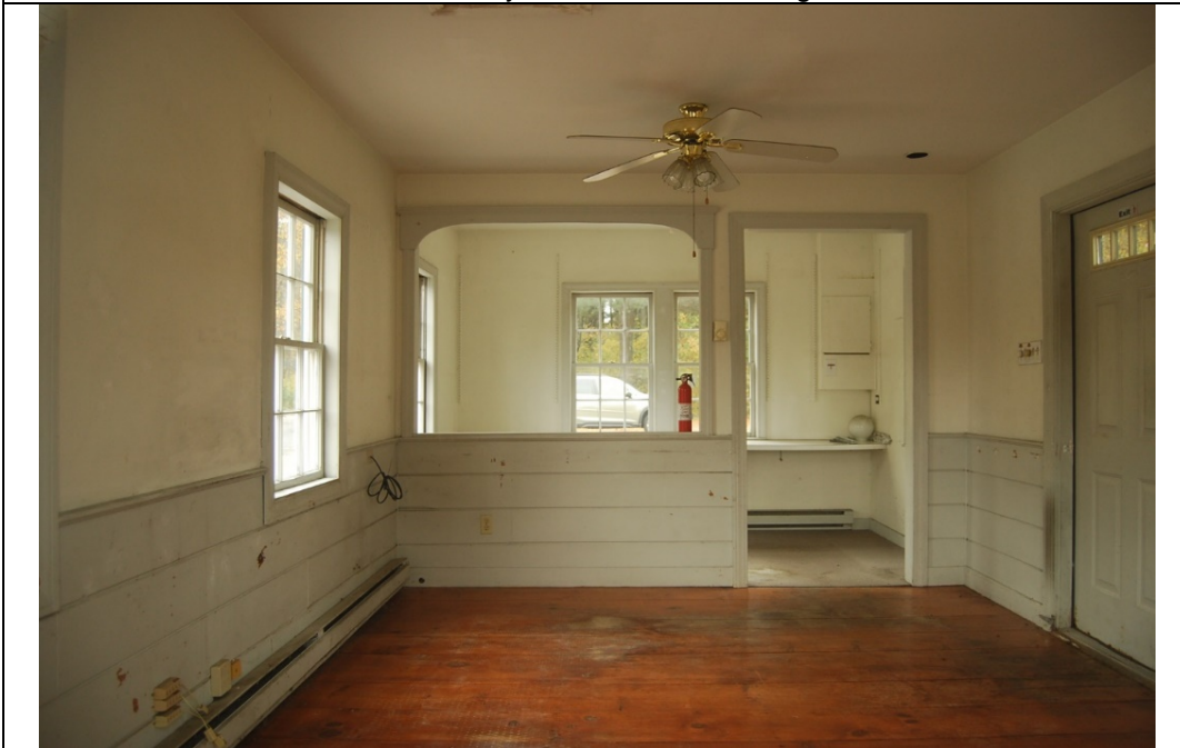
South Sudbury Station. Interior. View looking W.
