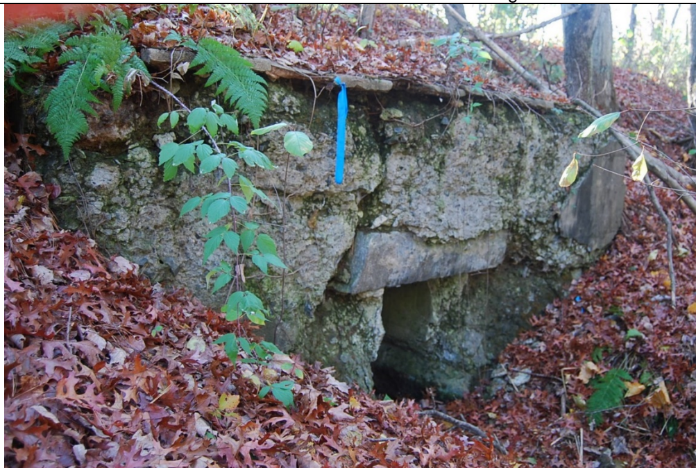
Culvert 127E. South elevation. View looking NE.
