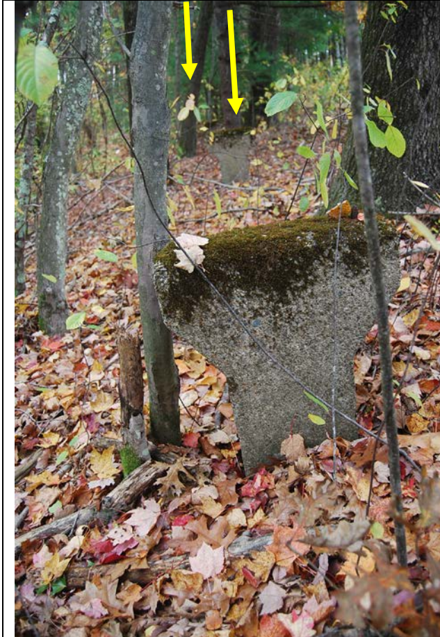
Rail Rest at MP 20.09. View looking E.
