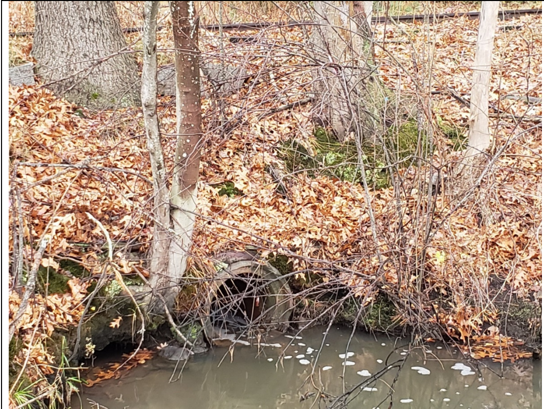
Culvert 127B. North elevation. View looking S.
