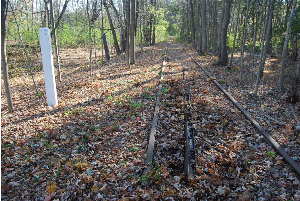
Railbed at grade near Section Tool House, near MP 19.75. View looking E. Whistle Post at left.
