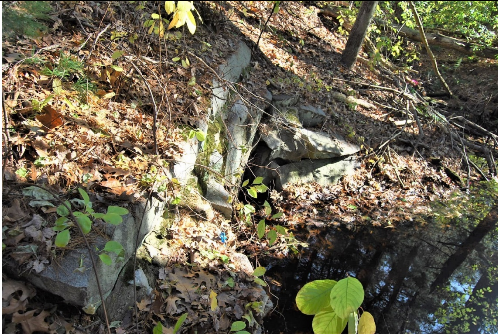
Culvert 127F. South elevation. View looking NE.
