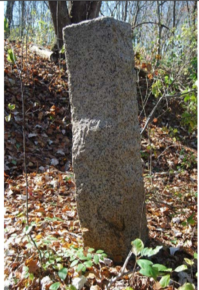
Milepost 19.0. East and north elevations. View looking SW.
