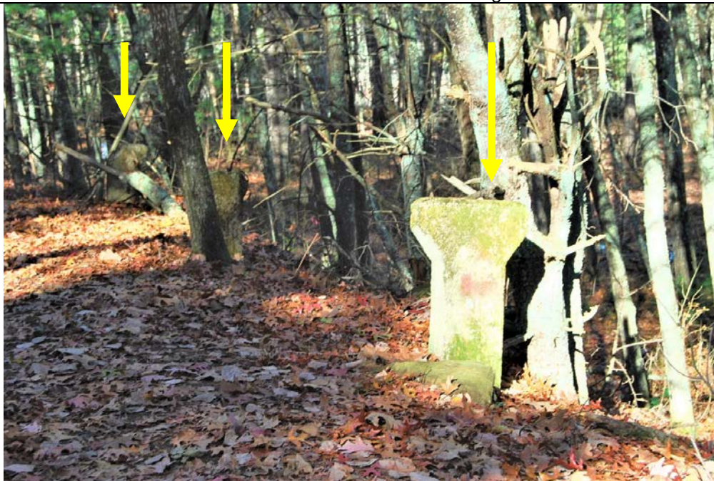
Rail Rest at MP 21.94. View looking W.
