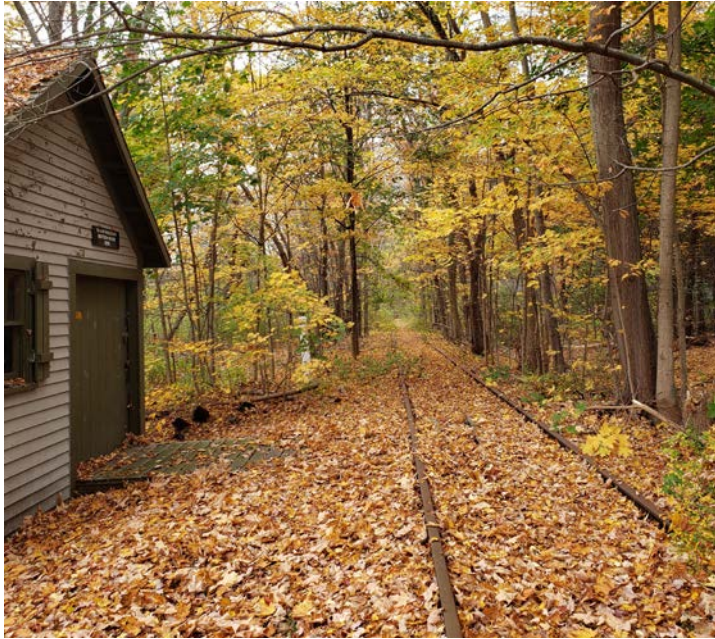
Central Massachusetts RR Corridor, looking east from Boston Post Road.
