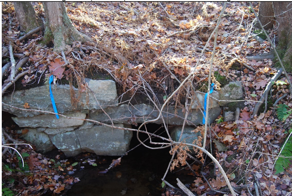
Culvert 126B. North elevation. View looking S.
