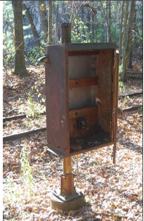
Relay Box at MP 20.13. North side of tracks. View looking SW "Candlestick" type.
