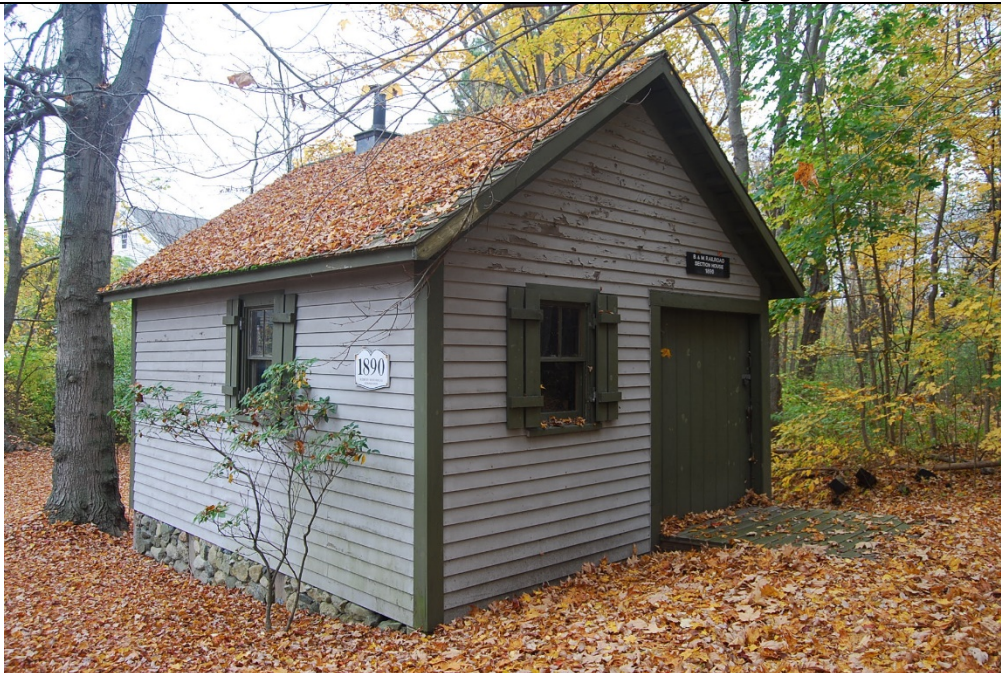
Section Tool House. West and South (trackside) elevations. View looking NE.
