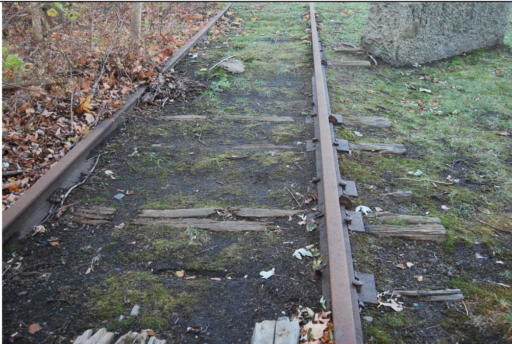
Railbed near Section Tool House, near MP 19.75. View looking W.
