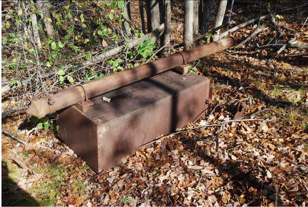
Signal Relay Box at MP 19.37. North side of track. "Candlestick" type.
