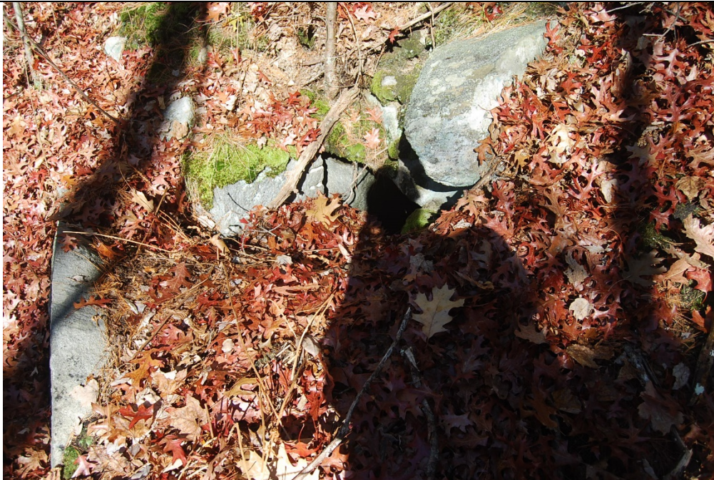
Culvert 127J. South elevation. View looking N.
