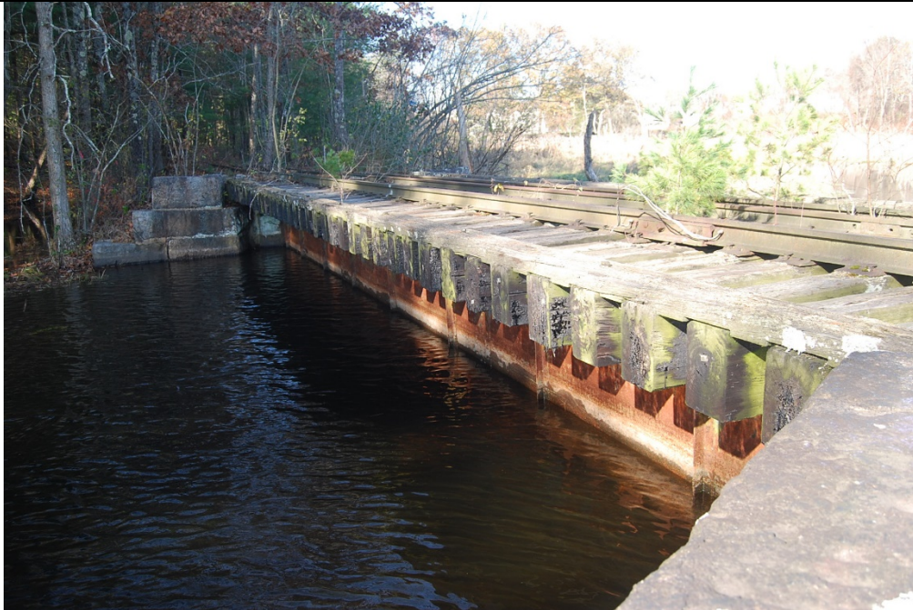
Bridge 127. (SUD.901) South elevation. View looking NW.
