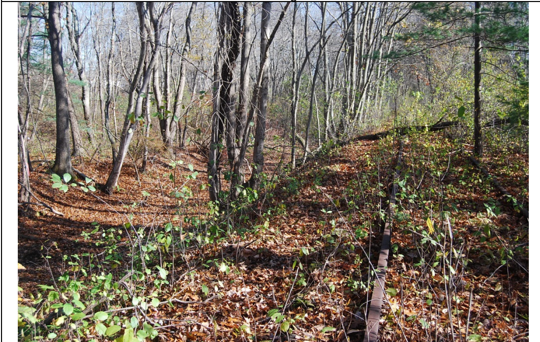
Railbed near MP 19.06, showing typical raised bed. View looking E.
