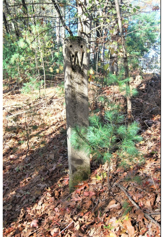
Whistle Post at MP 21.66. View looking NW.
