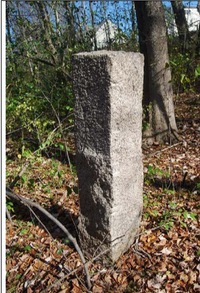
Milepost 19.0. West and south elevations. View looking NE. Notice smoother dressed area at top, where it would have been painted.
