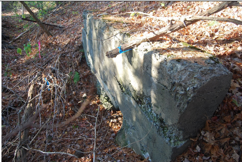
Culvert 127E. North elevation. View looking SE.
