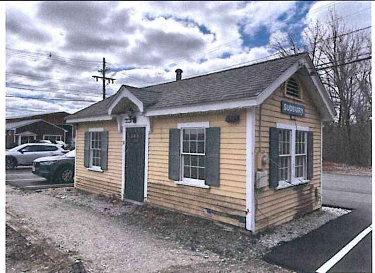
View to the southeast toward the station.
