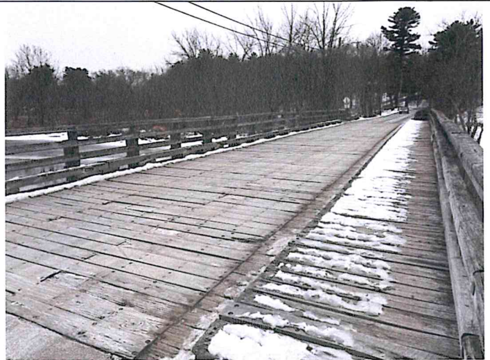
View to the south-southwest of the bridge planks and walkway.
