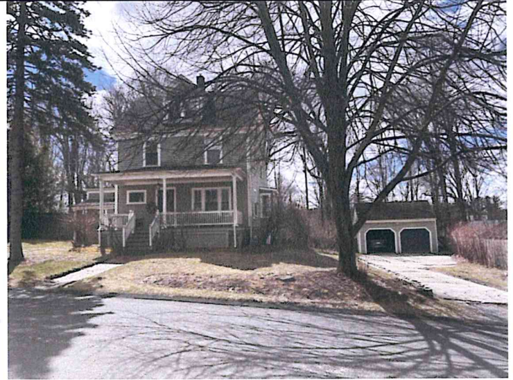
Photo 14. View to the south toward the Clifford Burr House (1905, SUD.226) at 9 Church Street.
