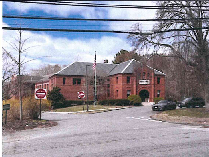
Photo 3. View to the west-northwest toward the Goodnow Public Library (1862, SUD.78) at 21 Concord Road.
