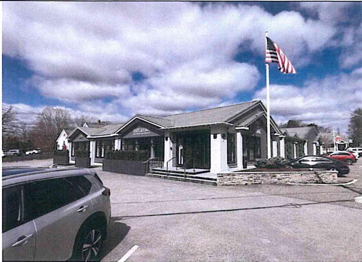
Photo 17. View to the northwest toward 5-15 Concord Road (1956, SUD.376).
