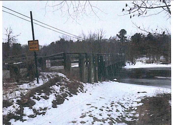
View to the southwest toward the bridge, from the east bank of the Sudbury River.
