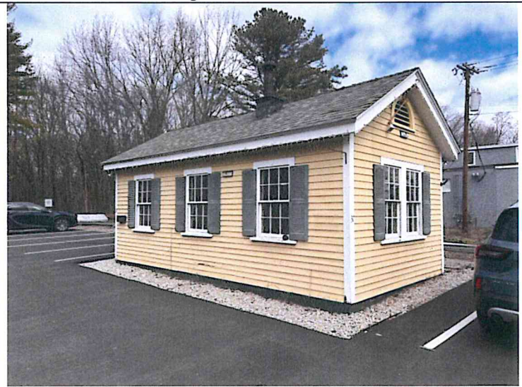
View to the northwest toward the station.
