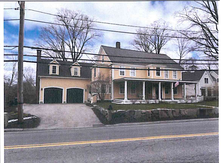
Photo 6. View to the west toward the Israel How Brown House (ca. 1725, SUD.85) at 71 Concord Road.
