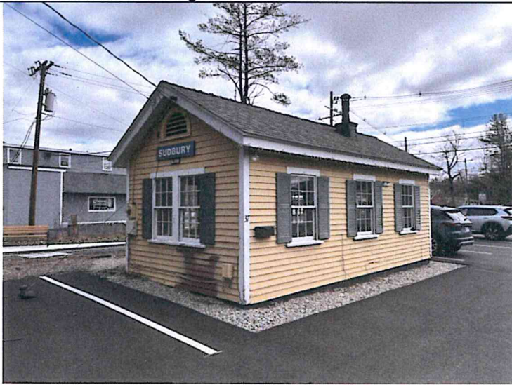
View to the northeast toward the station.
