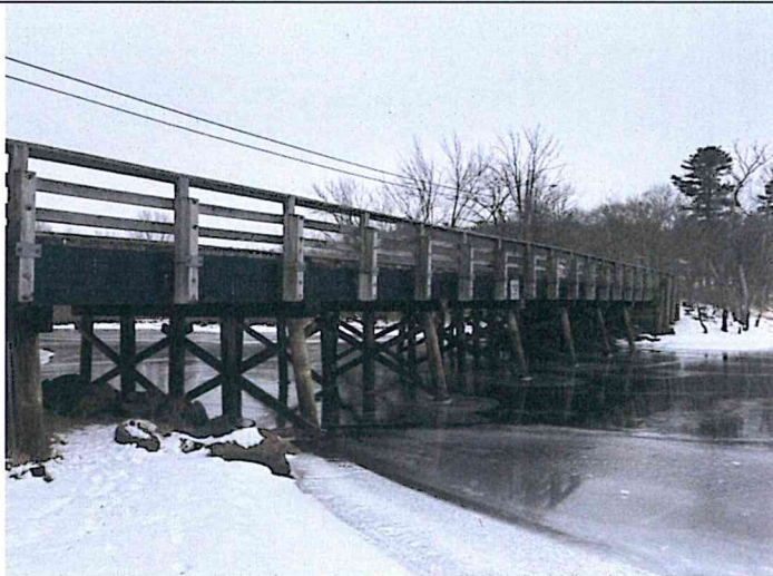
View to the south-southwest toward the bridge.
