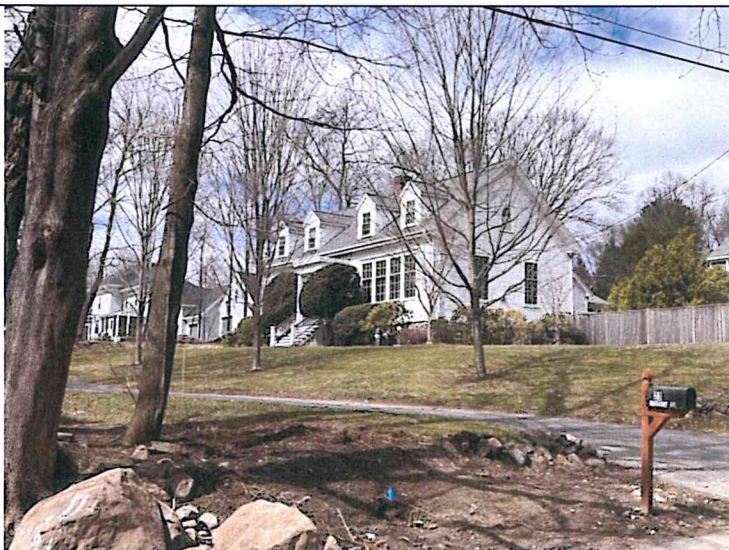
Photo 19. View to the northwest toward the Lanham Elementary School (1891, SUD.280) at 23 Massasoit Avenue.
