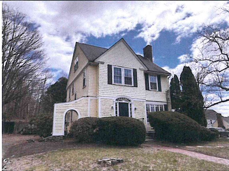
Photo 15. View to the east toward the Archer H. Townes House (1905, SUD.232) at 10 Concord Road.
