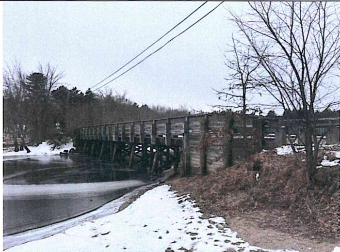
View to the west toward the bridge, from the east bank of the Sudbury River.
