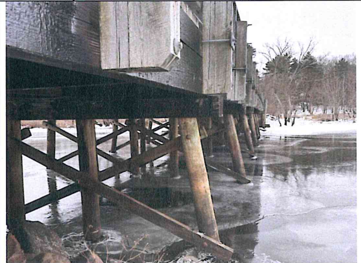
Detail view to the west-southwest of supports beneath the bridge, from the Wayland side.
