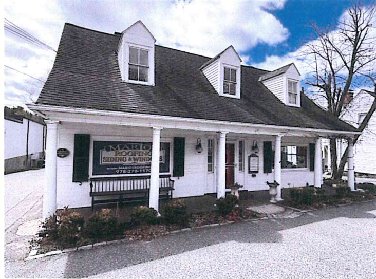
Photo 1. View to the southwest toward the Richardson House (1720, SUD.16) at 353 Boston Post Road.
