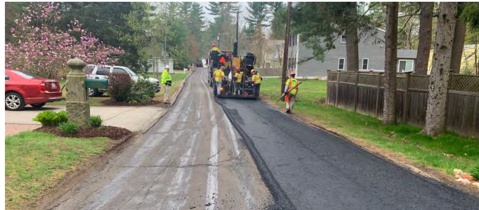
Road paving on a Sudbury street. Photo Credit: Town of Sudbury.
