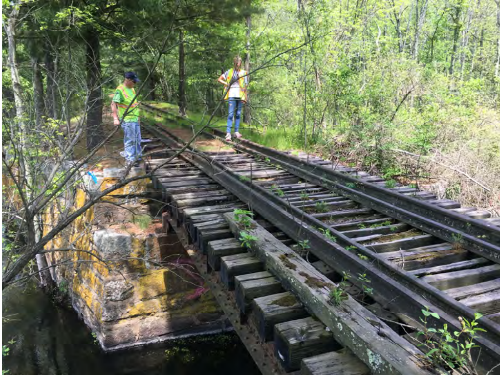
Photo 1: North Approach (Looking North)
