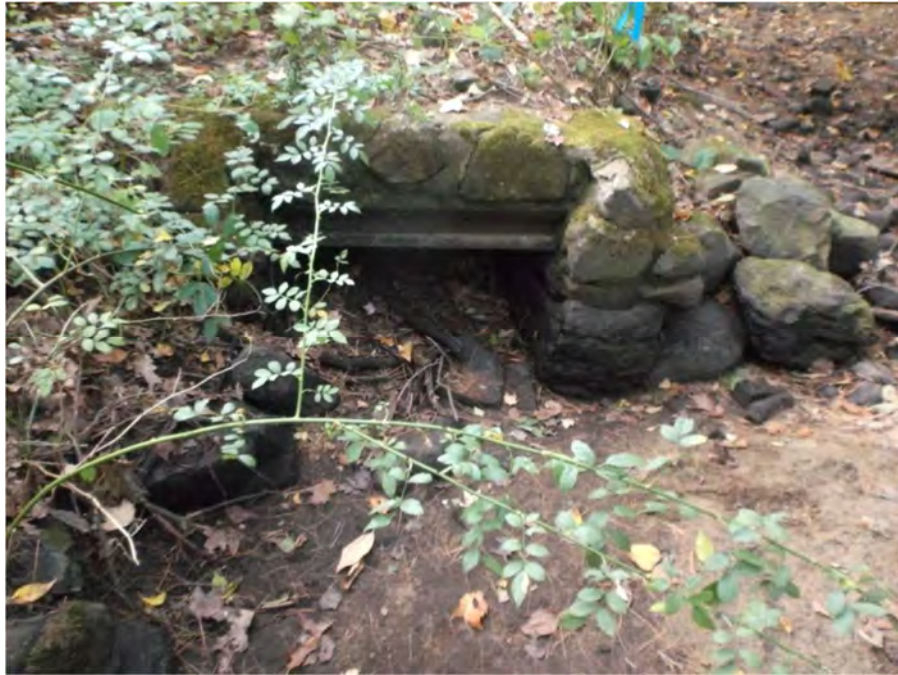
Photo 1: Upstream side of culvert
