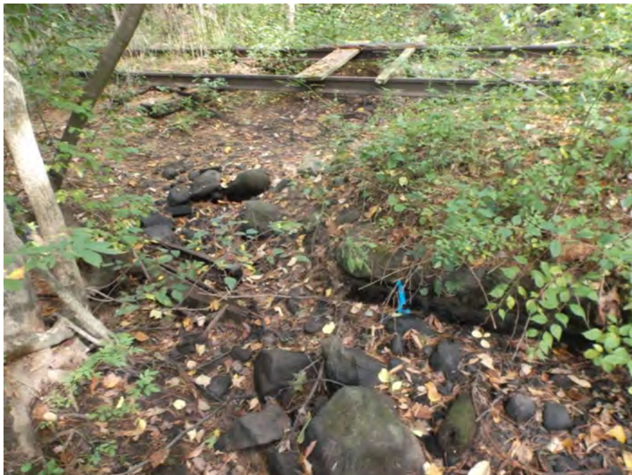
Photo 2: Downstream side of culvert
