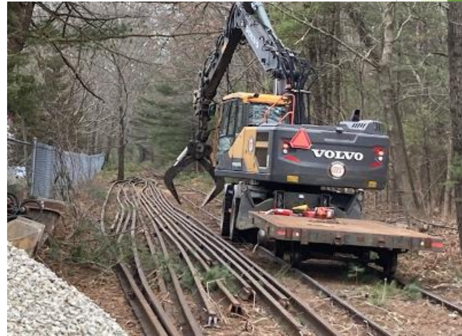
Construction Work at Hudson Road
