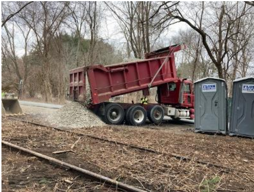
Gravel Dump at Hudson Road
