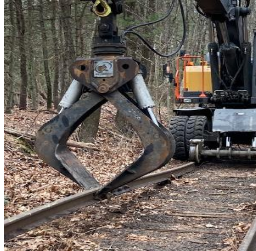
Lifting Rail South of Morse Road
