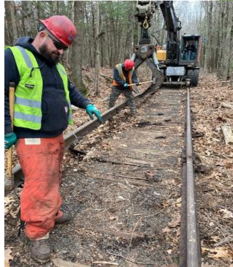
Removing Clips South of Morse Road
