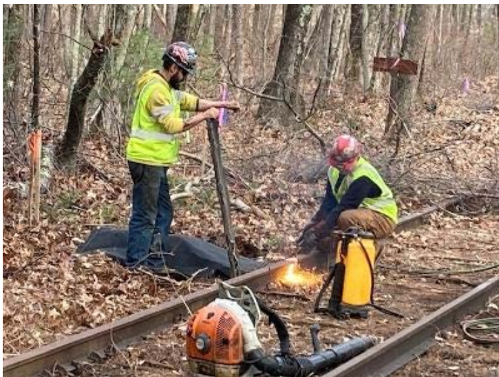
Cutting the track at the Diamond
