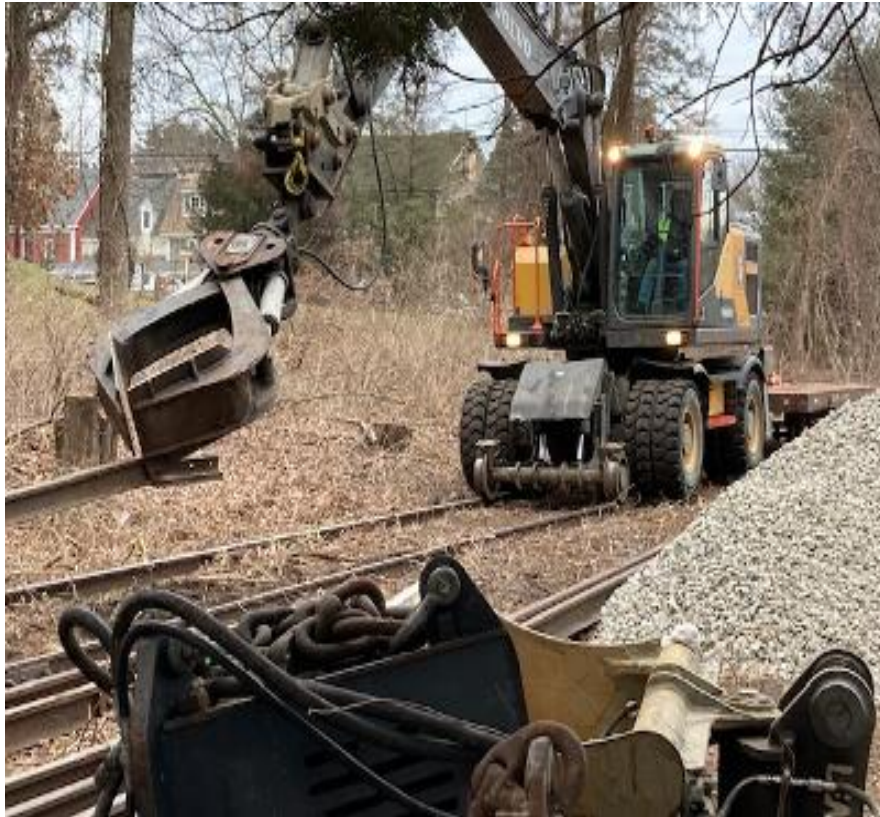
Construction Work at Hudson Road
