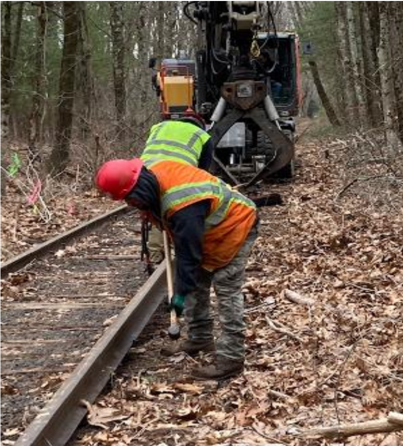
Removing Clips South of Morse Road
