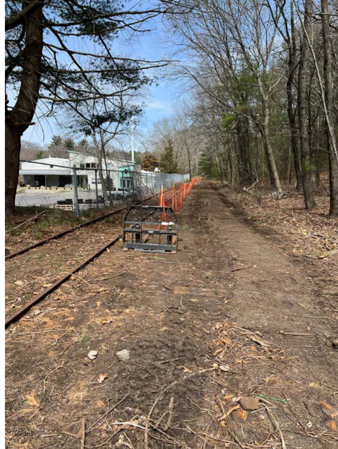
View North at Hudson Road
