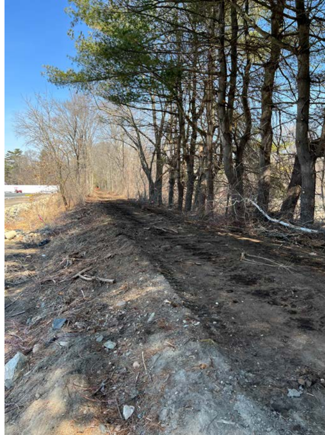
View North at Codjer Lane
