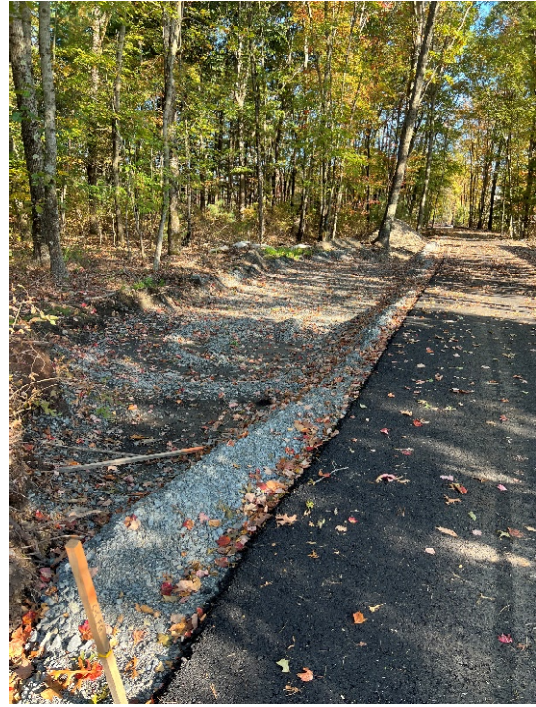
Photo 2: Sta. 101+00 looking north at the proposed rest area.
