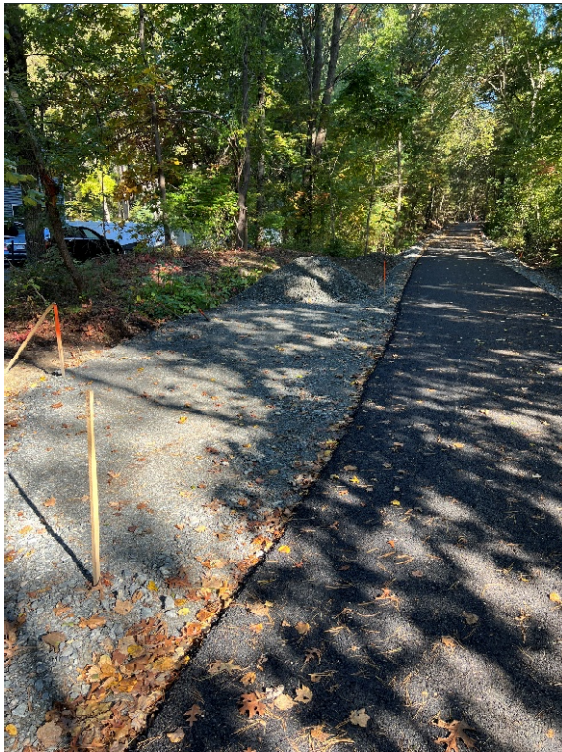
Photo 5: Sta. 143+00 looking north at the proposed rest area.
