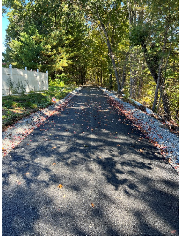
Photo 10. Sta. 325+00 looking north.
