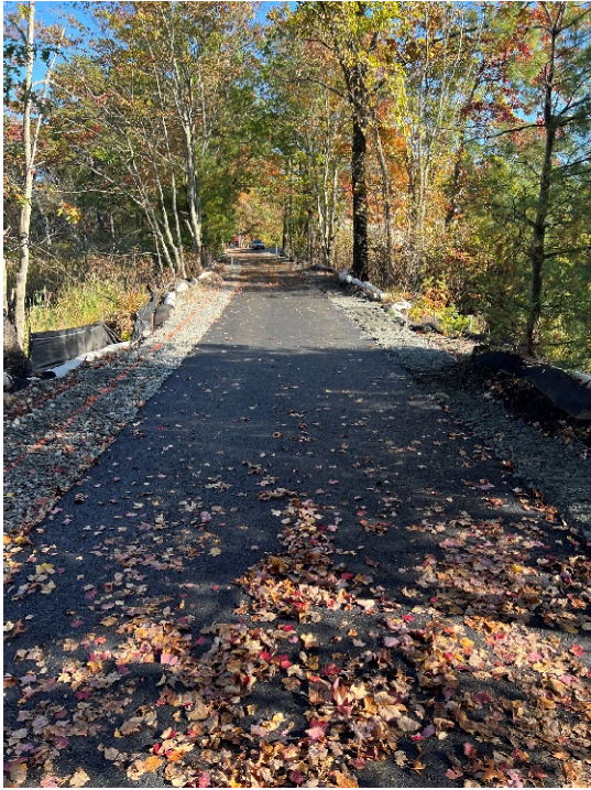
Photo 1: Sta. 106+00 looking north.
