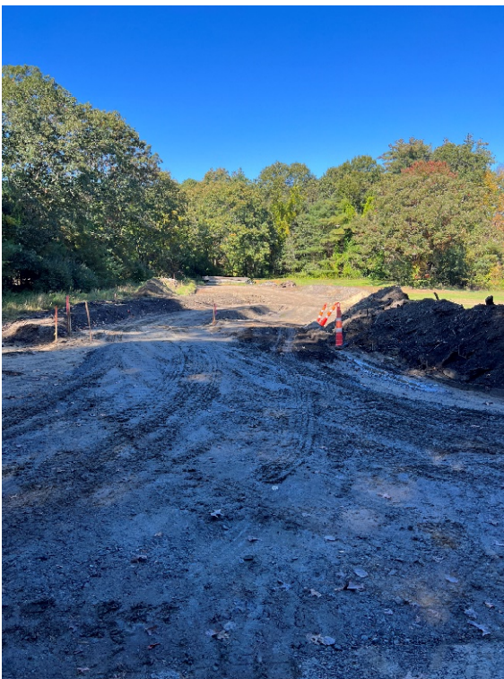
Photo 7: Sta. 184+50 looking west at the spur path.
