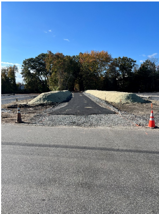
Photo 3: Sta. 116+00 looking south at the constructed berms.
