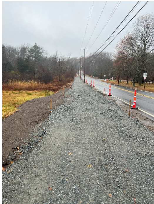
Photo 12: Sta. 1103+00 looking west at the trail grading efforts along North Road.
