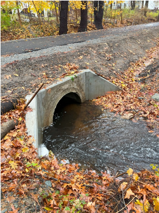
Photo 5: Sta 167+00 looking at the 48" culvert.
