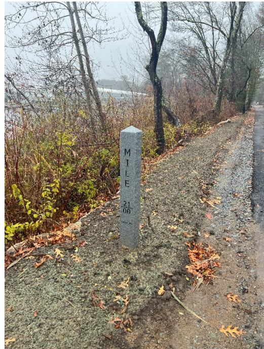
Photo 2: Sta. 120+00 looking north at a newly installed granite mile marker.
