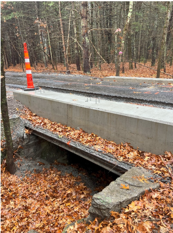
Photo 7: Sta. 190+50 looking at the cattle crossing currently under construction.
