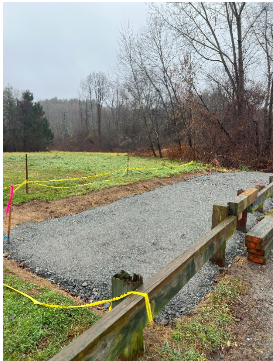
Photo 11: Sta. 1107+50 looking at the end of the Davis Field spur path.
