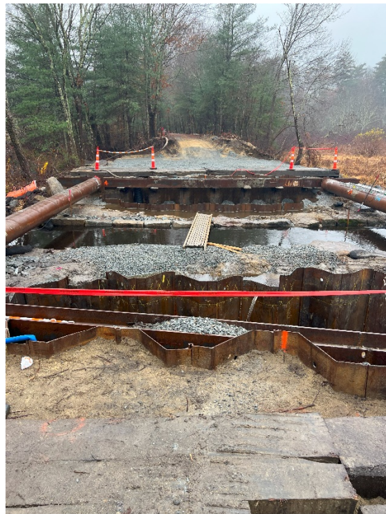
Photo 8: Sta. 265+00 looking south at Pantry Brook.
