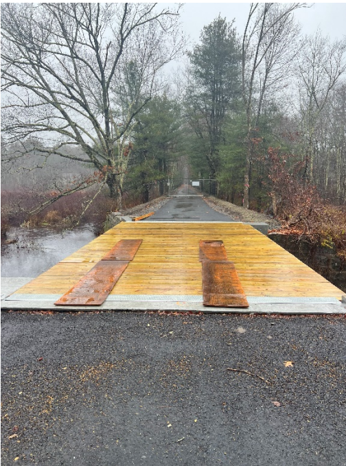
Photo 3: Sta. 126+00 looking north at the Hop Brook bridge.
