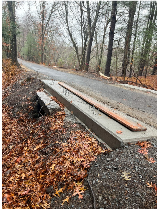
Photo 10: Sta. 321+50 looking at the cattle crossing under construction.
