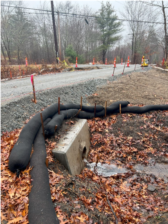
Photo 9: Sta. 306+50 looking north at the trail grading efforts.
