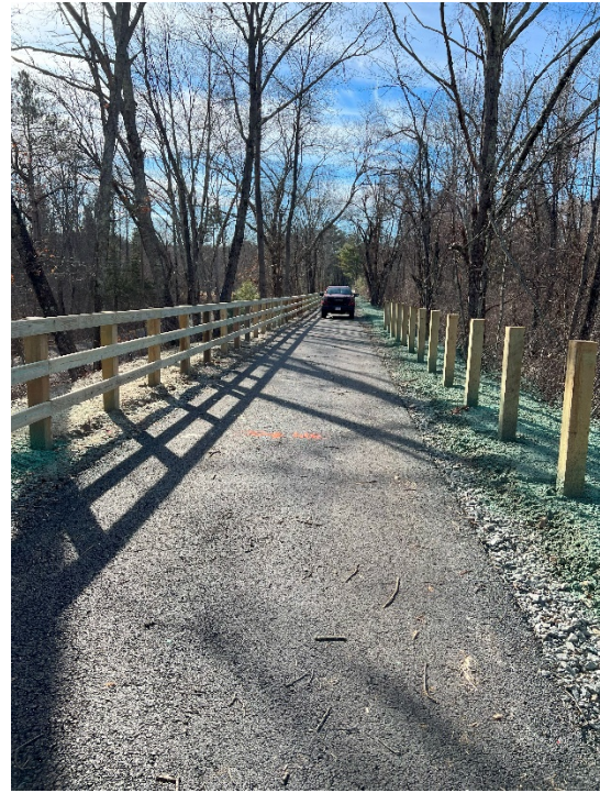
Photo 10: Sta. 314+50 looking south at the completed and in construction timber fencing.
