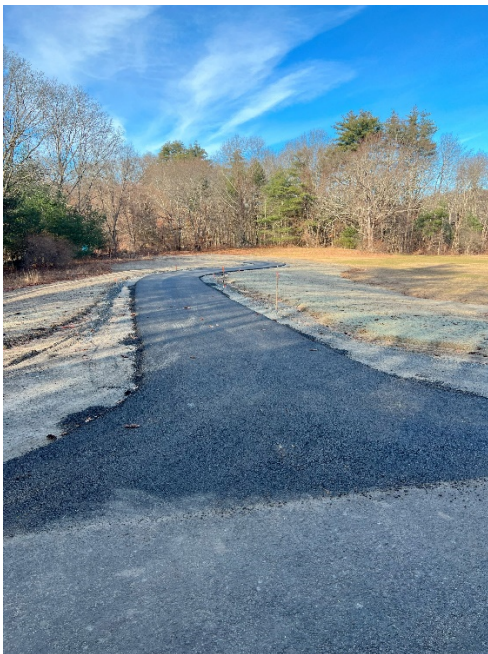
Photo 3: Sta. 184+50 looking west at the Parkinson's Lot spur path.
