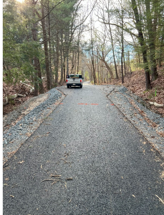
Photo 6: Sta. 234+00 looking south at the paved path and vehicle turnaround.
