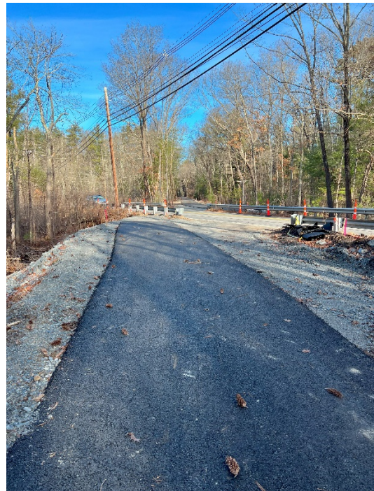
Photo 8: Sta. 283+00 looking north at Pantry Road.
