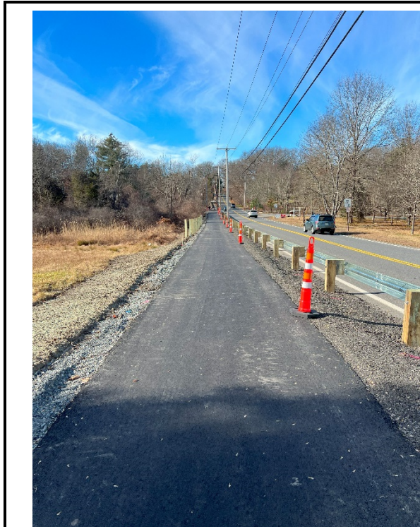
Photo 9: Sta. 1104+00 looking west at the paved spur path and installed guardrail.
