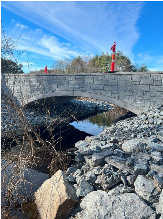
Photo 7: Sta. 164+50 looking at the newly constructed Pantry Brook bridge.
