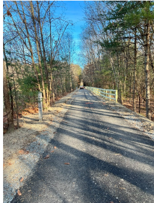
Photo 4: Sta. 185+00 looking north at the timber fencing.
