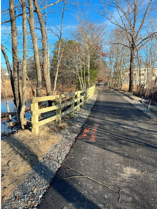
Photo 1: Sta. 104+50 looking north at the timber fencing.
