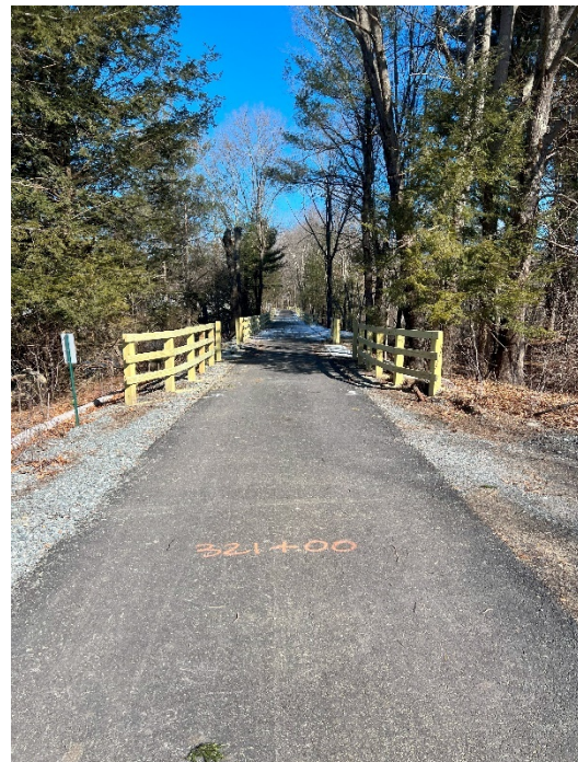
Photo 4: Sta. 321+00 looking north at the timber fencing.
