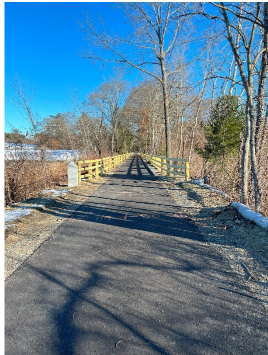
Photo 6: Sta. 119+50 looking north towards Hop Brook.
