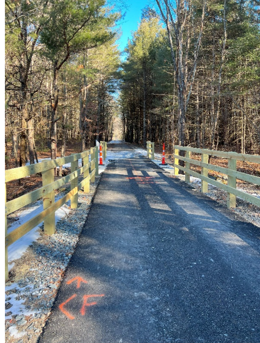
Photo 2: Sta. 190+00 looking north at the timber fencing.
