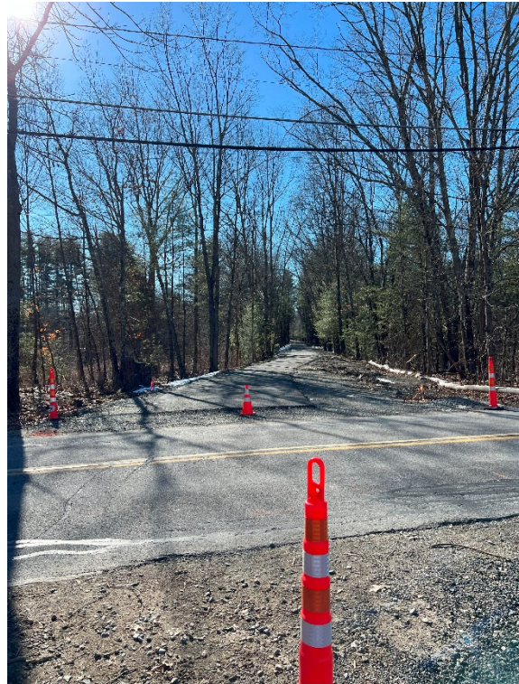
Photo 10: Sta. 275+50 looking south across Haynes Road.
