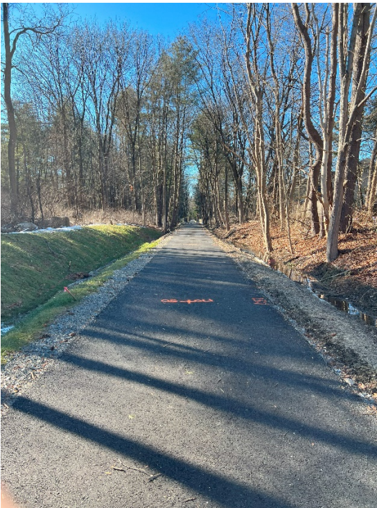
Photo 7: Sta. 180+00 looking south away from Hudson Road.
