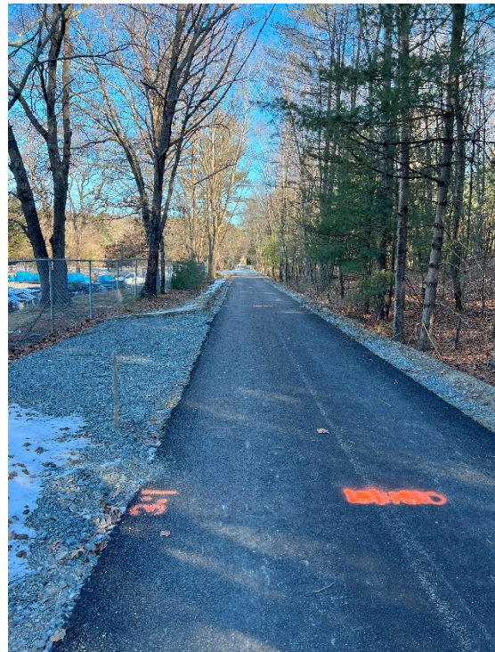
Photo 8: Sta. 181+50 looking north at the proposed rest area location.
