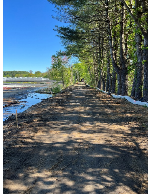
Photo 2: Sta. 116+00 looking north, standing at Codjer Lane.
