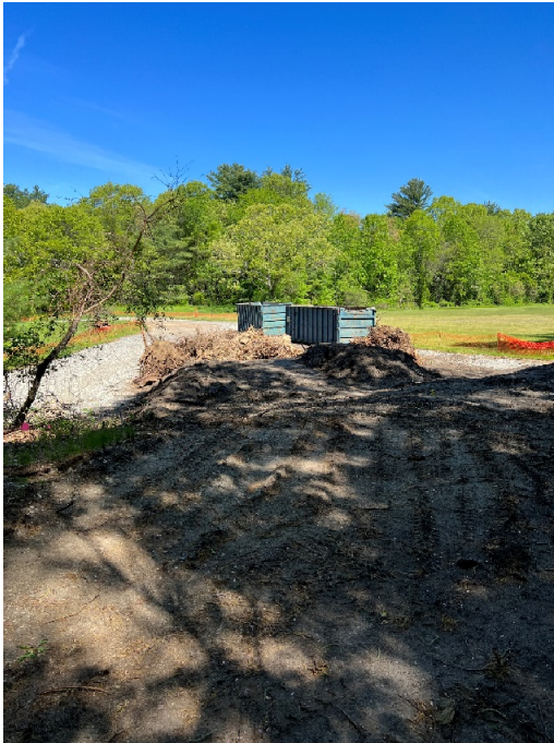
Photo 5: Sta 184+50 looking east towards the spur path behind Ti-Sales
