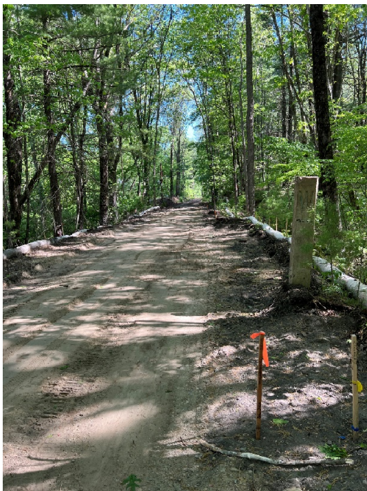
Photo 3: Sta. 161+50 looking north
