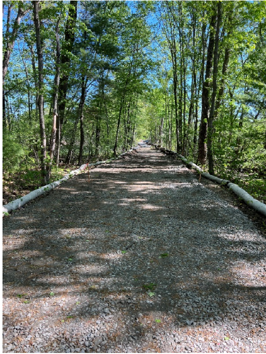
Photo 1: Sta. 105+00 looking north
