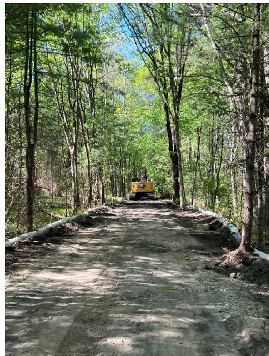
Photo 4: Sta. 158+00 looking south
