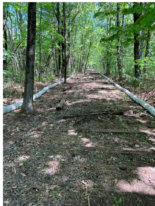
Photo 8: Sta. 278+00 looking north, standing towards Pantry Road
