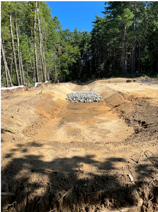
Photo 7: Looking at the detention basin in the proposed parking lot location
