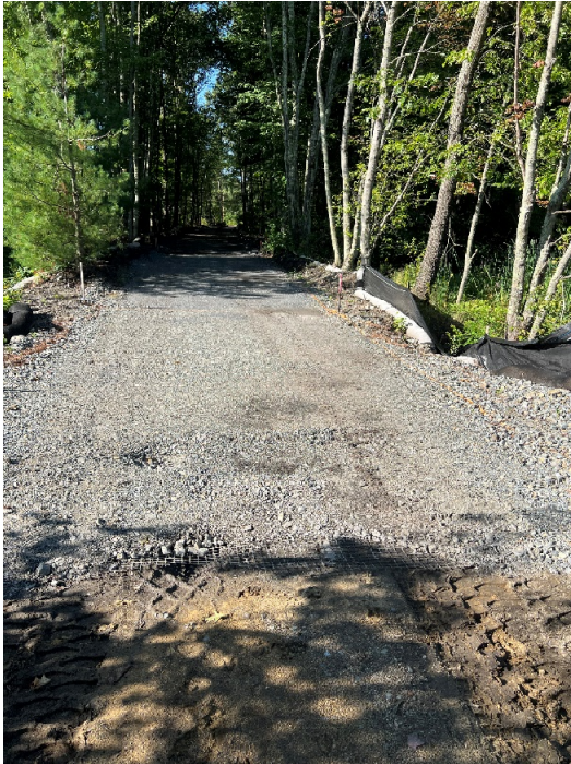
Photo 1: Sta. 105+25 looking south at the soil separation fabric
