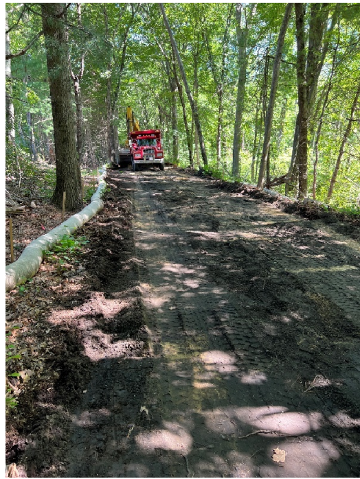
Photo 10. Sta. 330+00 looking north at the removal of topsoil
