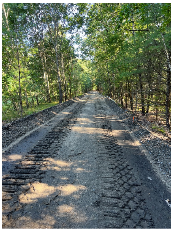
Photo 6: Sta. 187+00 looking north along the trail
