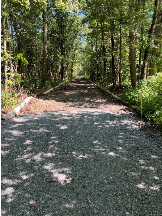
Photo 9. Sta. 279+00 looking north at the gravel course
