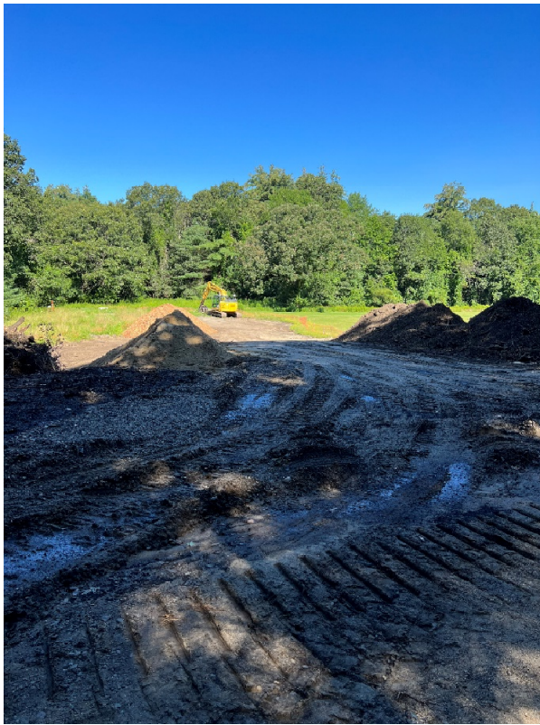
Photo 5: Sta 184+50 looking west at the spur path
