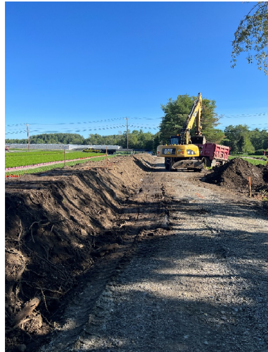
Photo 2: Sta. 114+00 looking north towards Codjer Lane at the proposed berms
