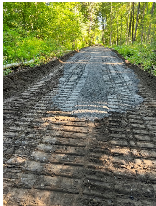
Photo 4: Looking north at the leveled soil around the culvert at Sta. 167+00
