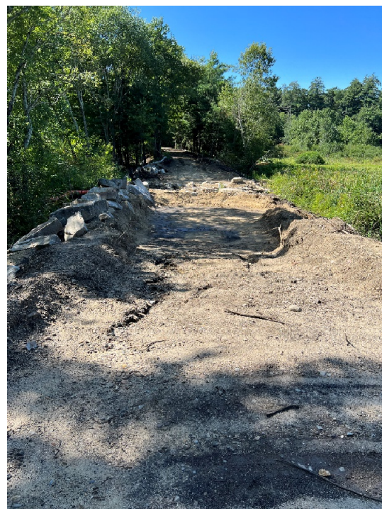
Photo 8: Sta. 265+00 looking south at the Pantry Brook bridge approach
