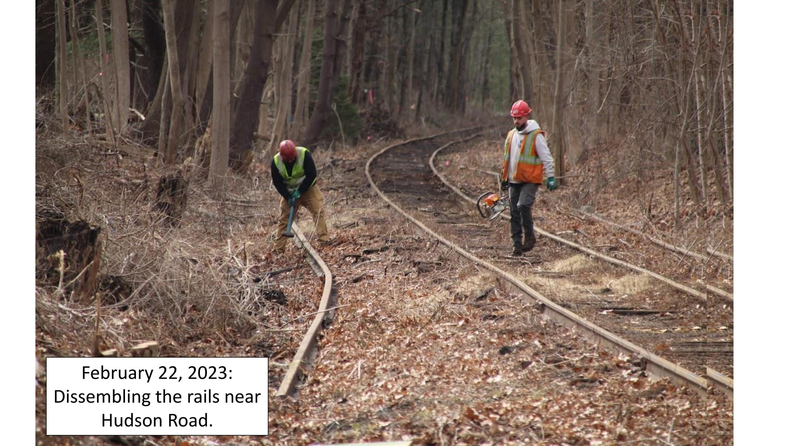
A photograph showing two workers in safety gear (hard hats and high-visibility vests) dismantling railroad tracks in a wooded area. The tracks are being removed from a path covered in fallen leaves and brush. One worker is using a tool to lift a rail, while the other is holding a chainsaw. The scene is set in a forest with many bare trees, suggesting a late autumn or winter setting.
