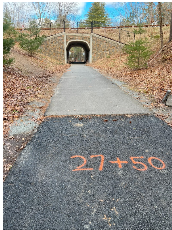
Photo 12: Sta. 27+50 in Concord looking north at the end of proposed work.
