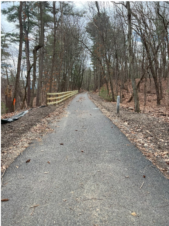
Photo 11: Sta. 23+00 in Concord looking south at the proposed fencing and granite mile marker.
