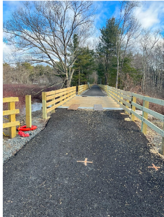
Photo 2: Sta. 126+00 looking north at the timber fencing across Hop Brook.
