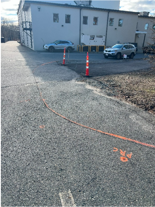
Photo 1: Proposed trail bump out sawcut and markings at the 71 Union Ave Driveway.
