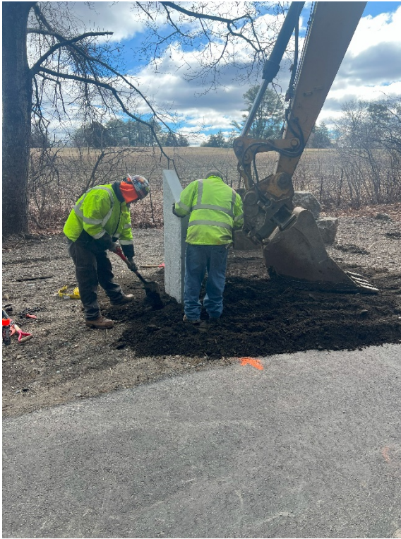
Photo 9: Sta. 261+00 looking at the proposed granite post being installed.
