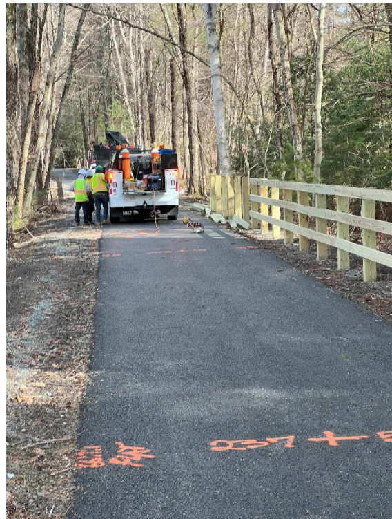
Photo 8: Sta. 237+00 looking north at fence installation.
