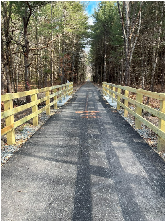
Photo 5: Sta 190+00 looking north at the fencing over the cattle crossing.
