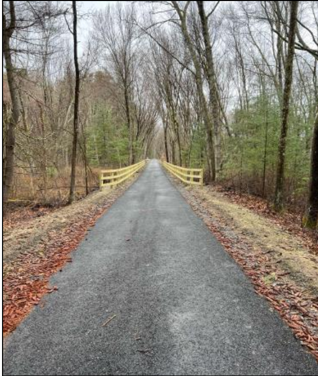
Mineway Brook Crossing
