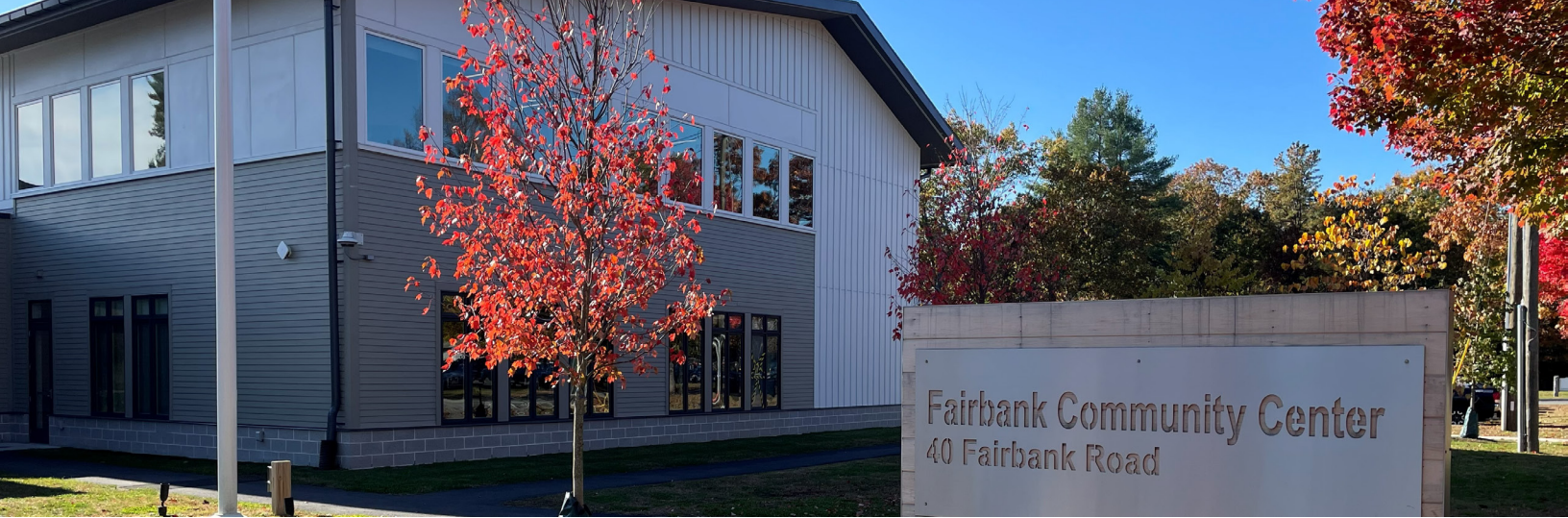
Fairbank Community Center, Credit: BSC Group
