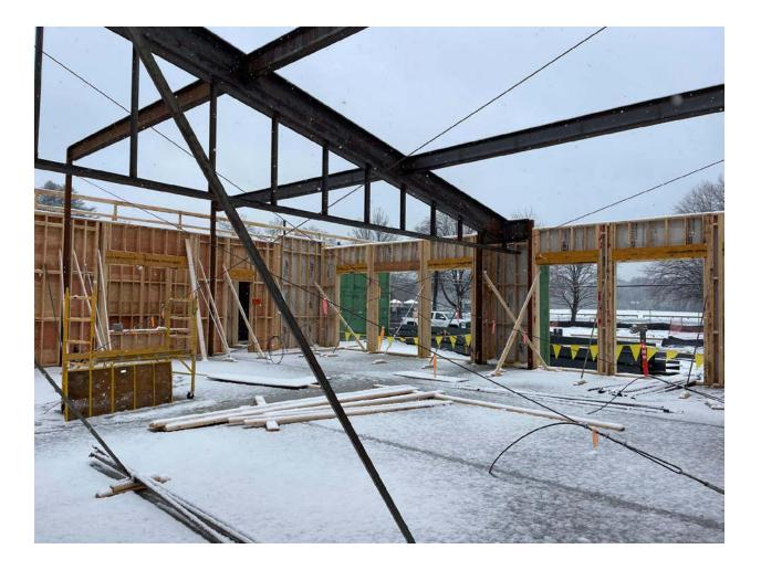
The framers continue to work on the walls that will form the rest of the building, and have begun work on the roof over the shared spaces in the middle - the multipurpose, fitness, and arts & crafts rooms. Curbing is complete for the locker room partitions.
