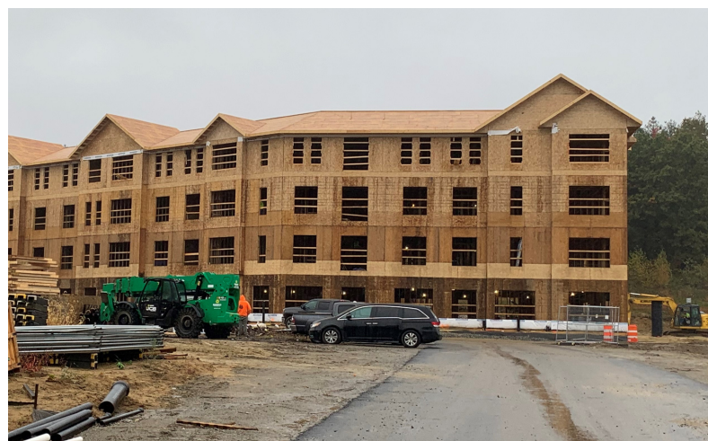
Cold Brook Crossing units under construction.
