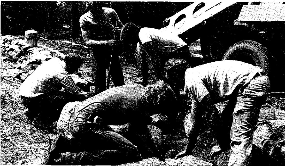
CONCORD ROAD WALKWAY CONSTRUCTION progressed through the summer on schedule as a result of the good planning of the Town Engineering Department. Here a stone wall was moved to make room for the walkway. (Clay Allen photo)
