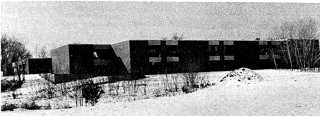
PETER NOYES SCHOOL ADDITION was completed this year under direction of the Permanent Building Committee. (Clay Allen photo)
