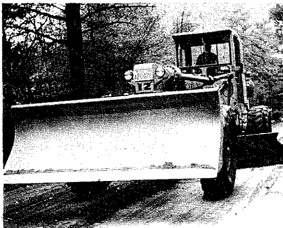
LONG-AWAITED RECONSTRUCTION of Pratts Mill Road took place this year. (Jordan photo)
