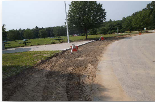
Pictured Above: Walkway construction in progress at Curtis Middle School
