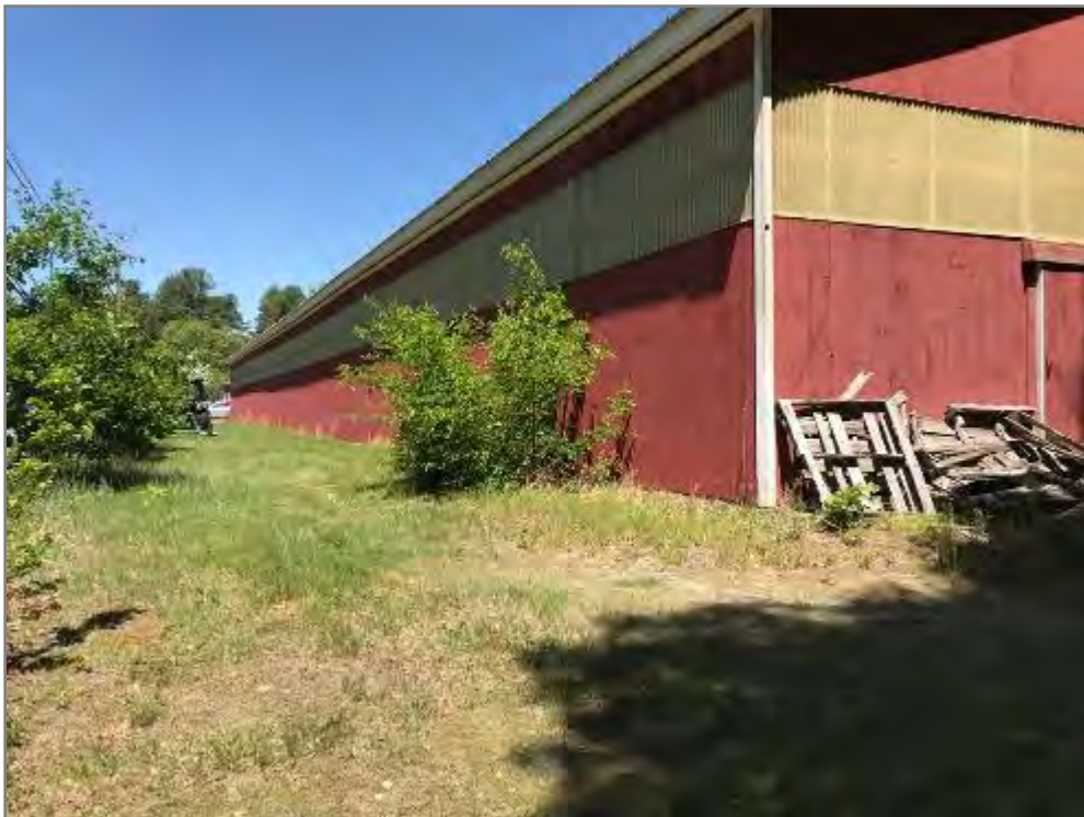
Photo #8 – Indoor riding arena on northeastern portion of F09-0002.
