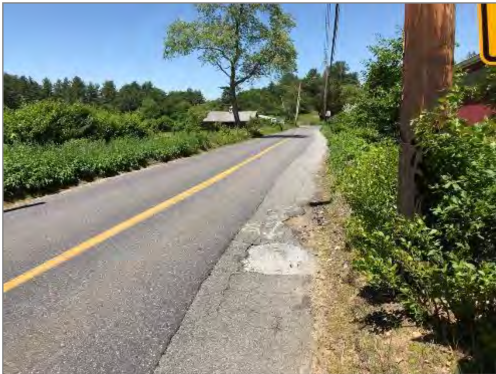
Photo #10 – Additional northwesterly view of Morse Road frontage.
