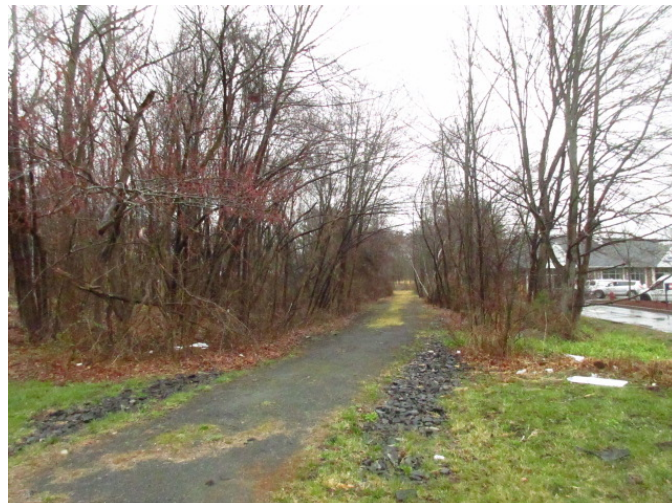
2. NORTHERLY DIRECTION ALONG RAIL CORRIDOR AT BOSTON POST RD
